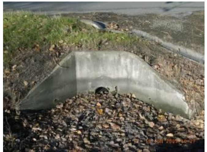
Culvert Headwall. This is not a retaining wall.
