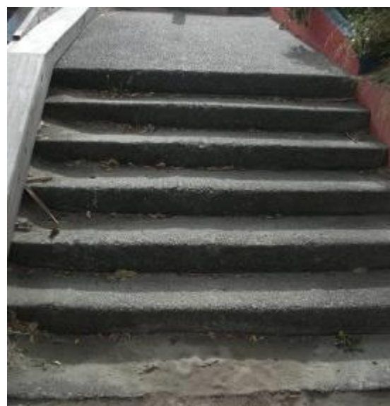
Concrete constructed stairs.
