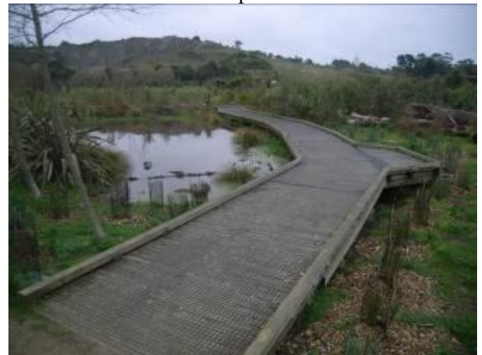
Boardwalk constructed of wood. This boardwalk has no handrail but does have a plastic geotech product non-slip surface.
