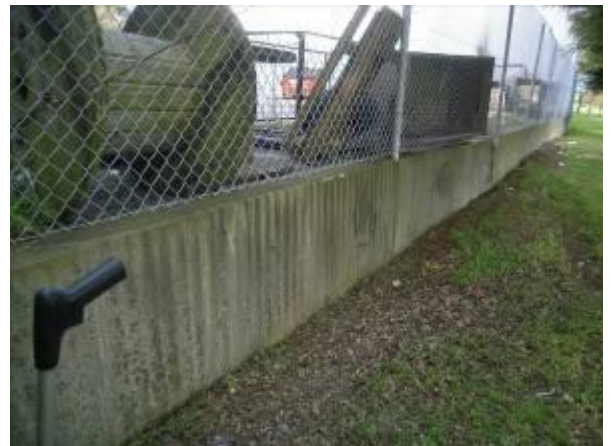
Concrete Retaining wall. This is a privately owned as it supports fill on private property.
