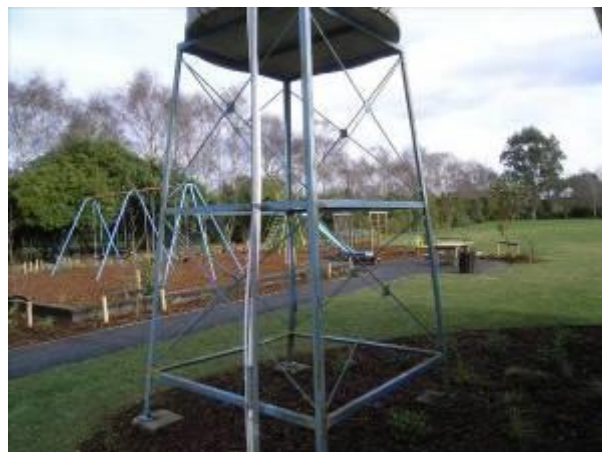
Steel water tower.
