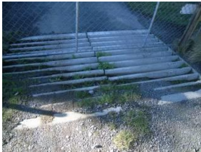
Concrete Cattle Stop. This cattle stop will be wider than it is long.
