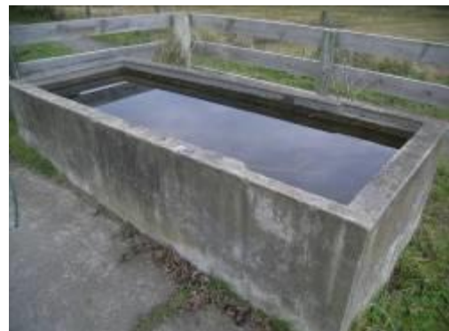
Rectangular concrete water trough. No ballcock.
