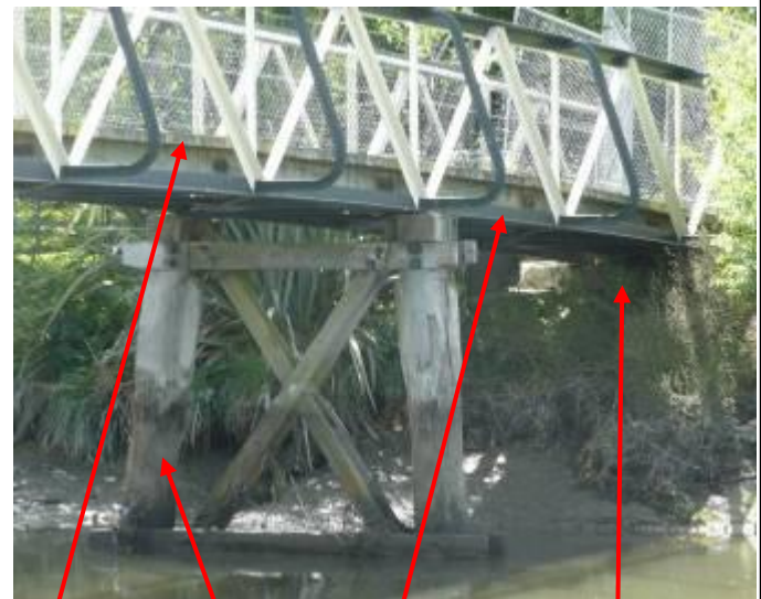
Deck Support Beam Abutment
