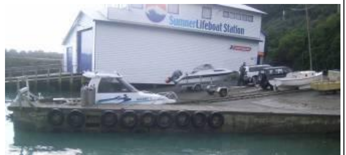
Solid Concrete Jetty
