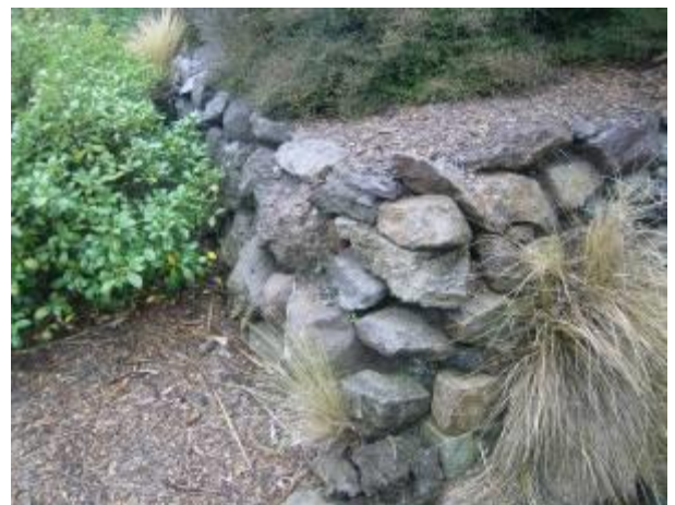
Council owned stone retaining wall.
