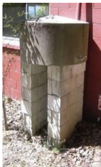
Concrete block water tower.
