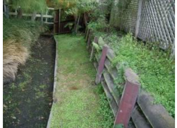
Wooden Retaining wall. This is a privately owned as it supports fill on private property.
