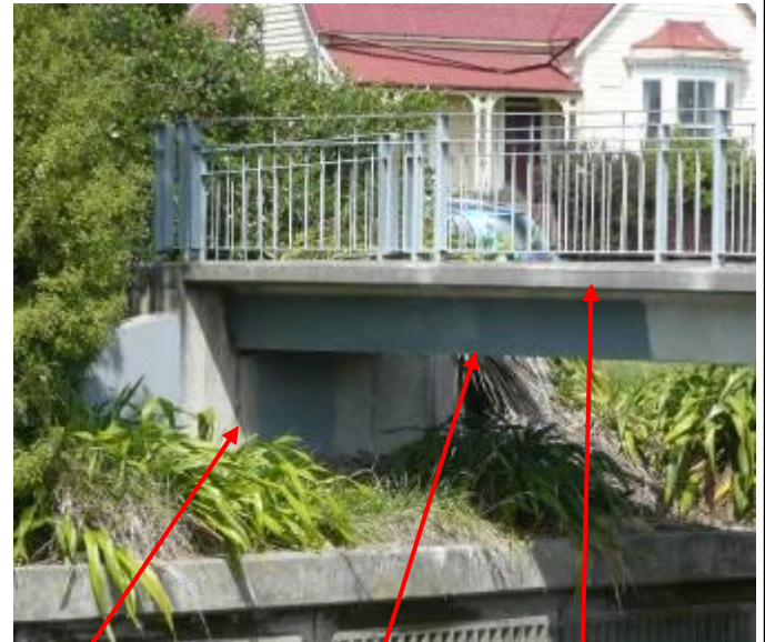
Abutment Beam Deck
