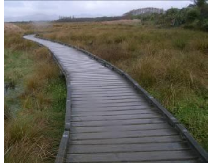
Boardwalk constructed of wood. This boardwalk has no handrail or non-slip surface
