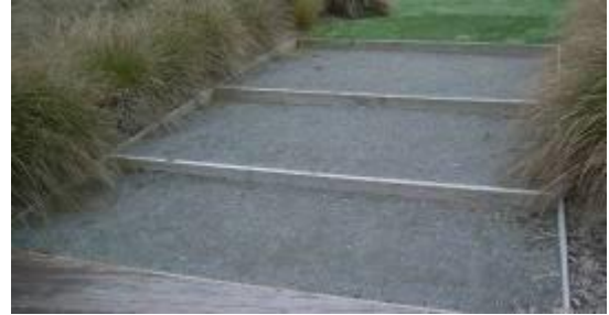
Inground stairs with wooden stringers and gravel tread.
