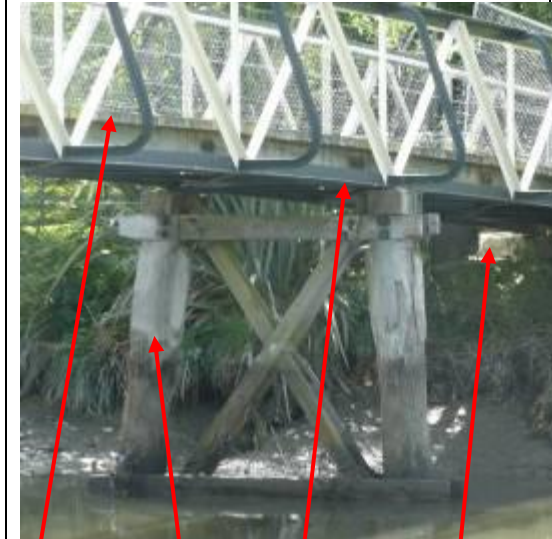
Deck Support Beam Abutment
