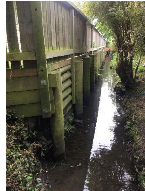
Timber lining true left and a retaining wall
