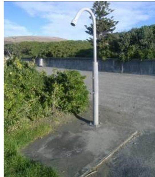
Steel shower with a galvanised surface finish. This shower has one shower head and a tap. No grate, drainage to the ground
