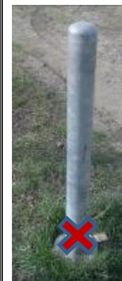
Steel removable and lockable bollard with a galvanized surface finish.
