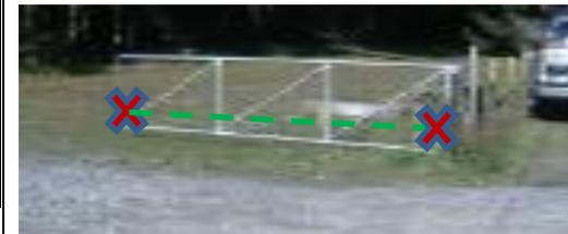
Gate Type of vehicular, gate style of standard farm gate, construction material of steel, post material of wood, surface finish of galvanised
