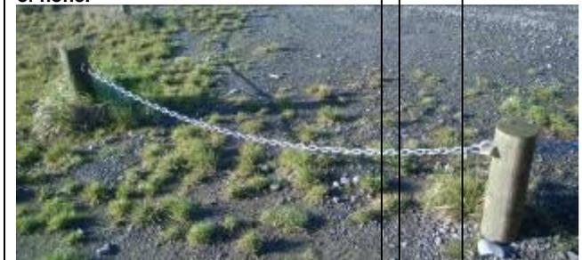
Gate type of vehicular, gate style of post and cable, construction material of chain, post material of wood, surface finish of galvanised
