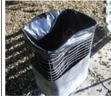
Steel cage style litter bin with bag but no liner. This bin has a galvanised surface finish and a concrete footpad.
