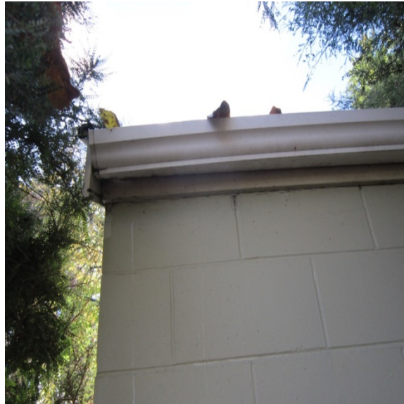
Photo 9: Gutter and south masonry wall.
