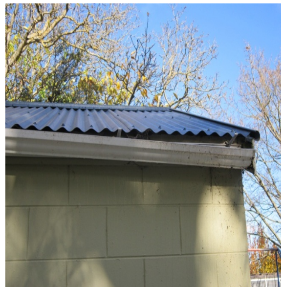
Photo 16: Sloped gutter on north side due to loose support connection.
