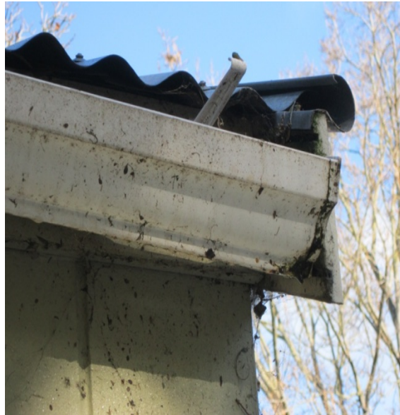
Photo 17: Sloped gutter on north side due to loose support connection.
