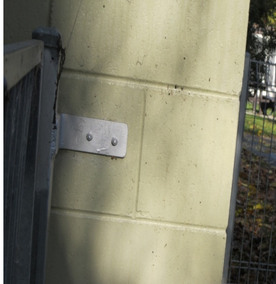
Photo 21: Anchors into masonry elements on north side for top gate connection.
