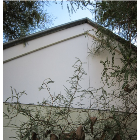
Photo 14: Roof cladding over south masonry wall.
