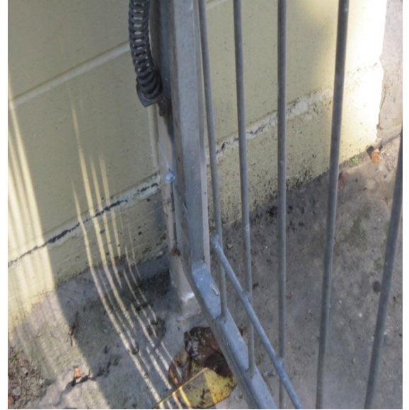
Photo 22: Gate ground connection on north side.
