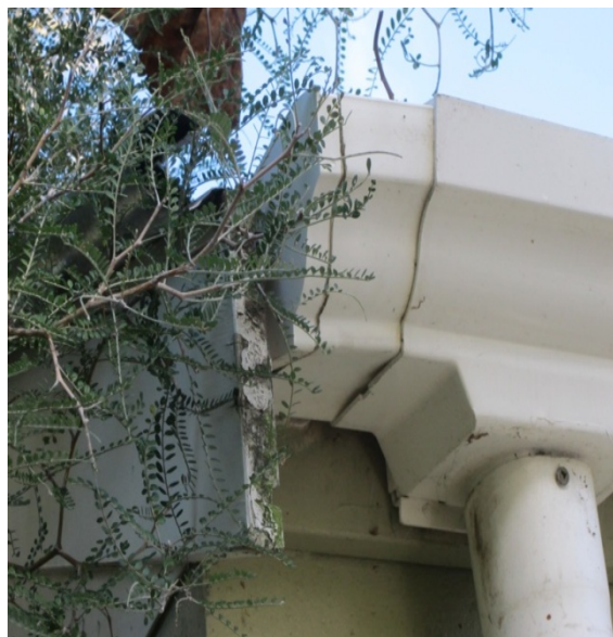
Photo 15: Gutter and downpipe on north side.
