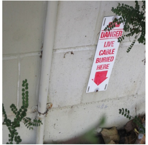
Photo 10: West masonry wall and footing underneath.
