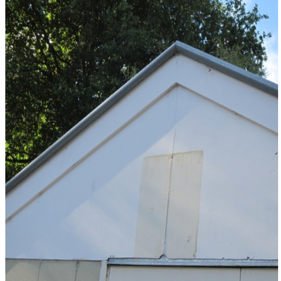
Photo 6: Roof cladding over west masonry wall and entrance.
