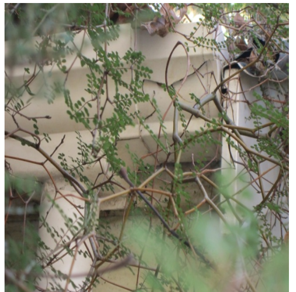
Photo 12: Gutter and downpipe on south side.
