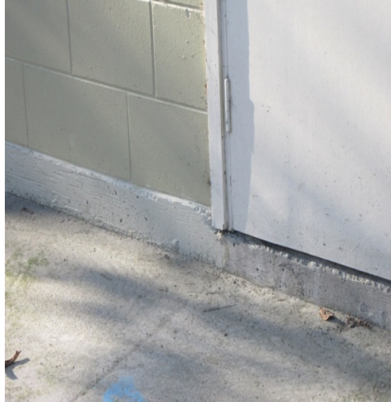
Photo 5: Concrete footing under masonry wall and entrance on west side.
