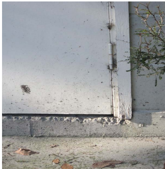
Photo 7: Spalling of low quality concrete footing under entrance on west side.
