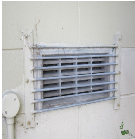
Photo 11: Ventilation grate on west wall. Anchors in masonry blocks.
