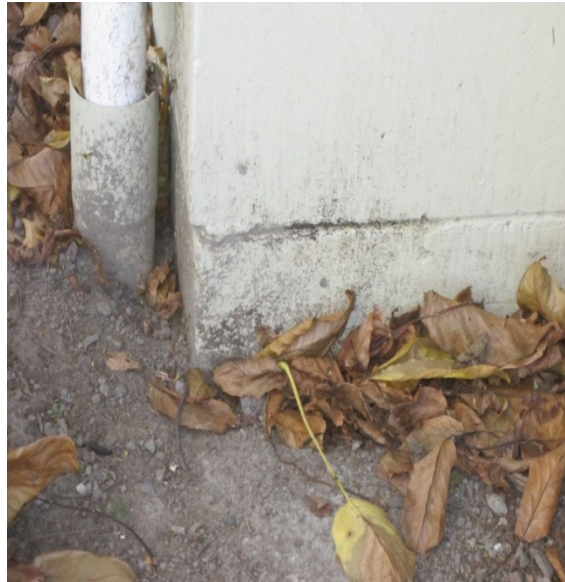
Photo 13: Downpipe from south gutter and footing on east side.
