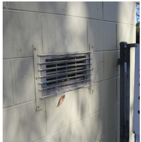
Photo 20: Ventilation grate on east wall. Anchors in masonry blocks.
