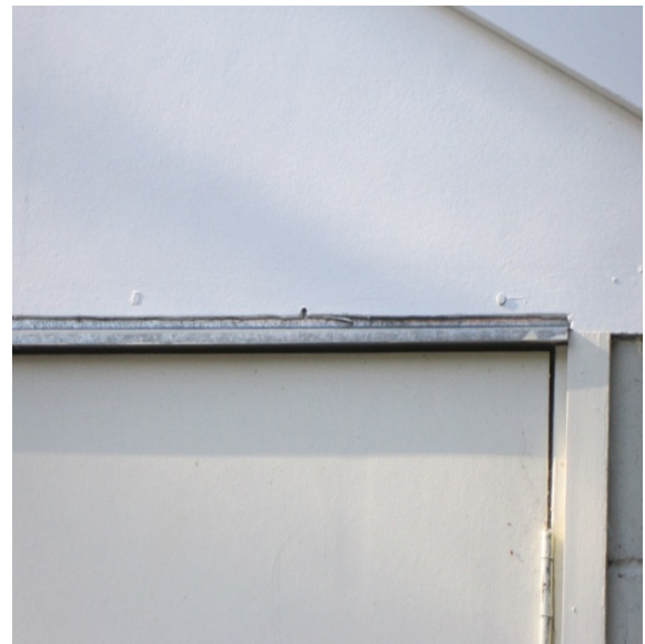
Photo 8: Doorframe for entrance on west side.
