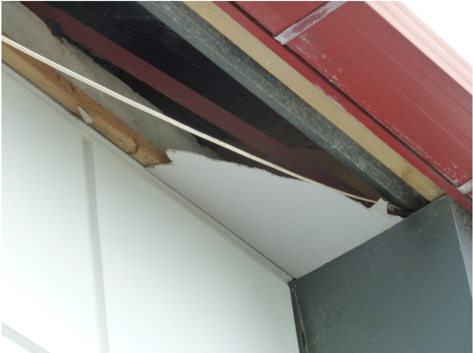
Photo 14 - External view of west wall precast panel
