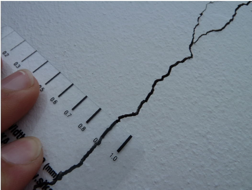
Photo 11 - Diagonal crack along the south wall exterior approximately 0.9mm
