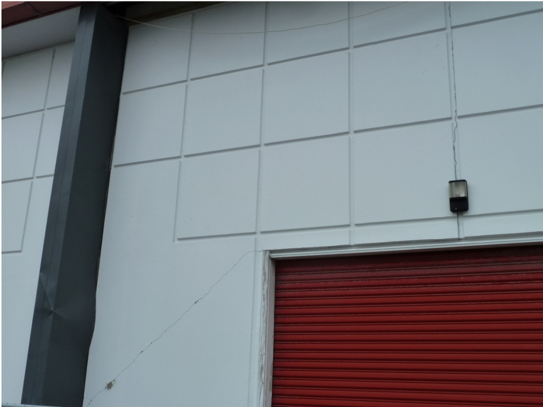
Photo 8 - Cracks located around the large access opening
