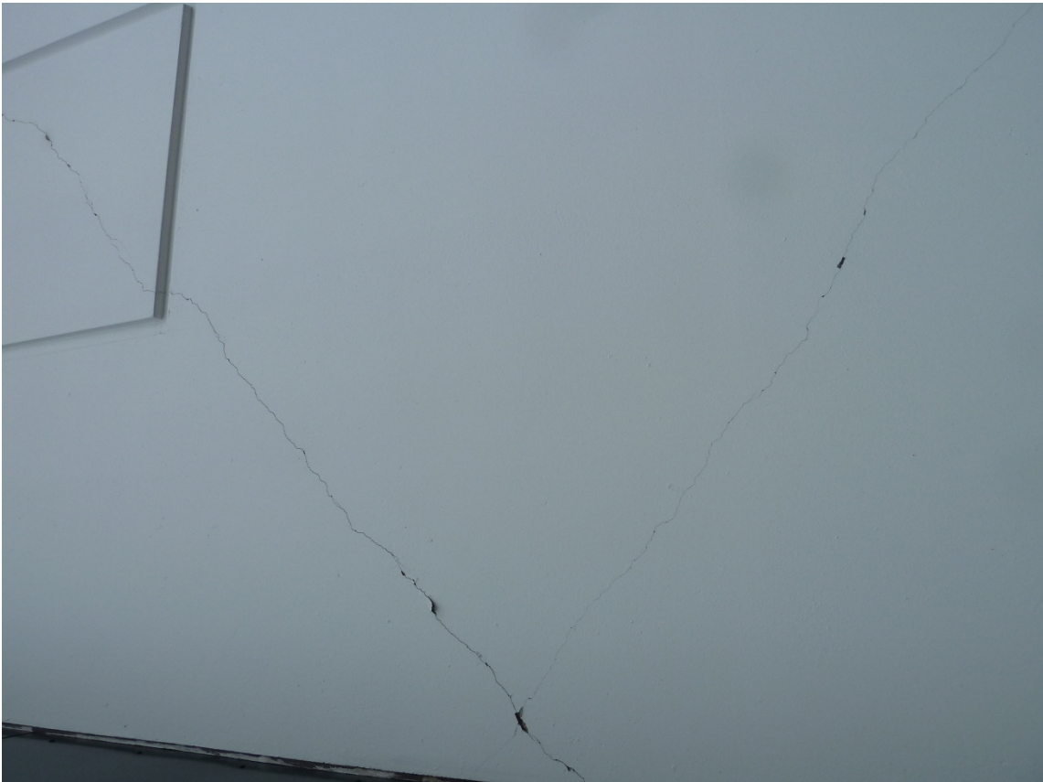
Photo 2 – Diagonal cracks in the west wall precast panel
