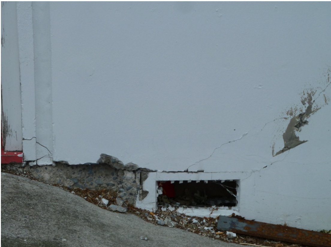
Photo 12 - Cracking/Spalling at the base of the south wall
