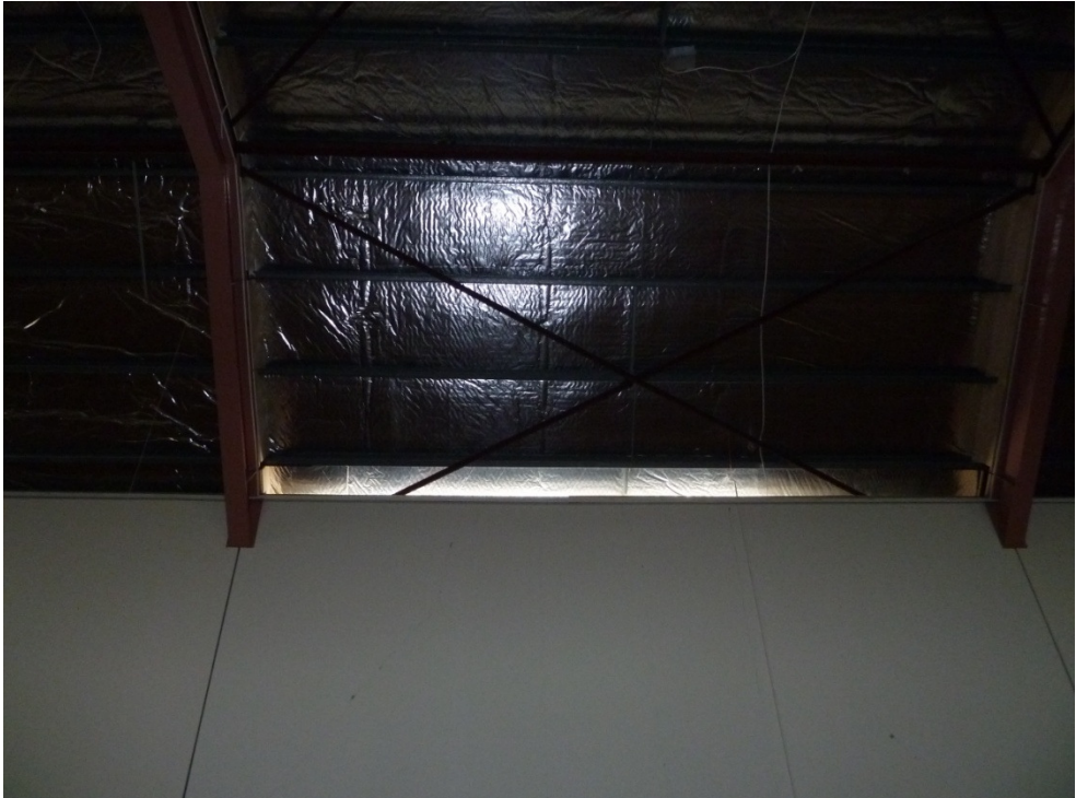
Photo 15 - Interior view of west wall precast panel
