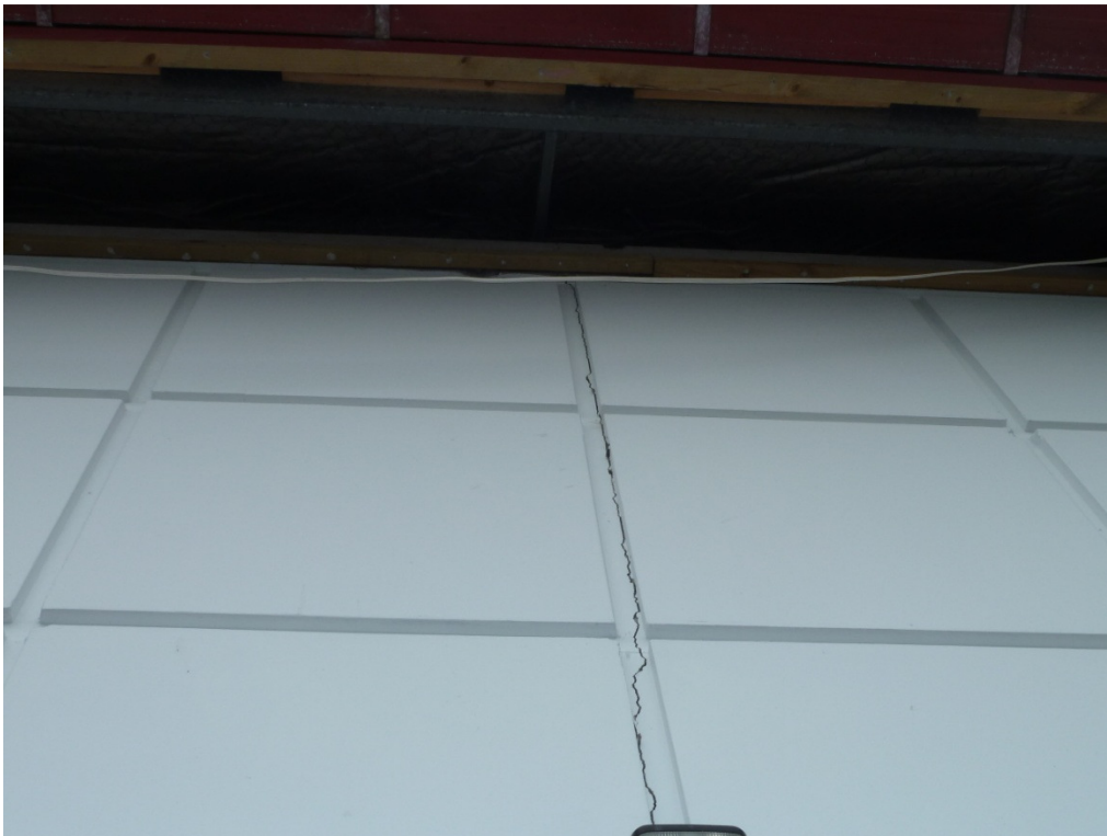
Photo 9 - Vertical crack propagating from the access way in the south wall panel approximately 5mm width
