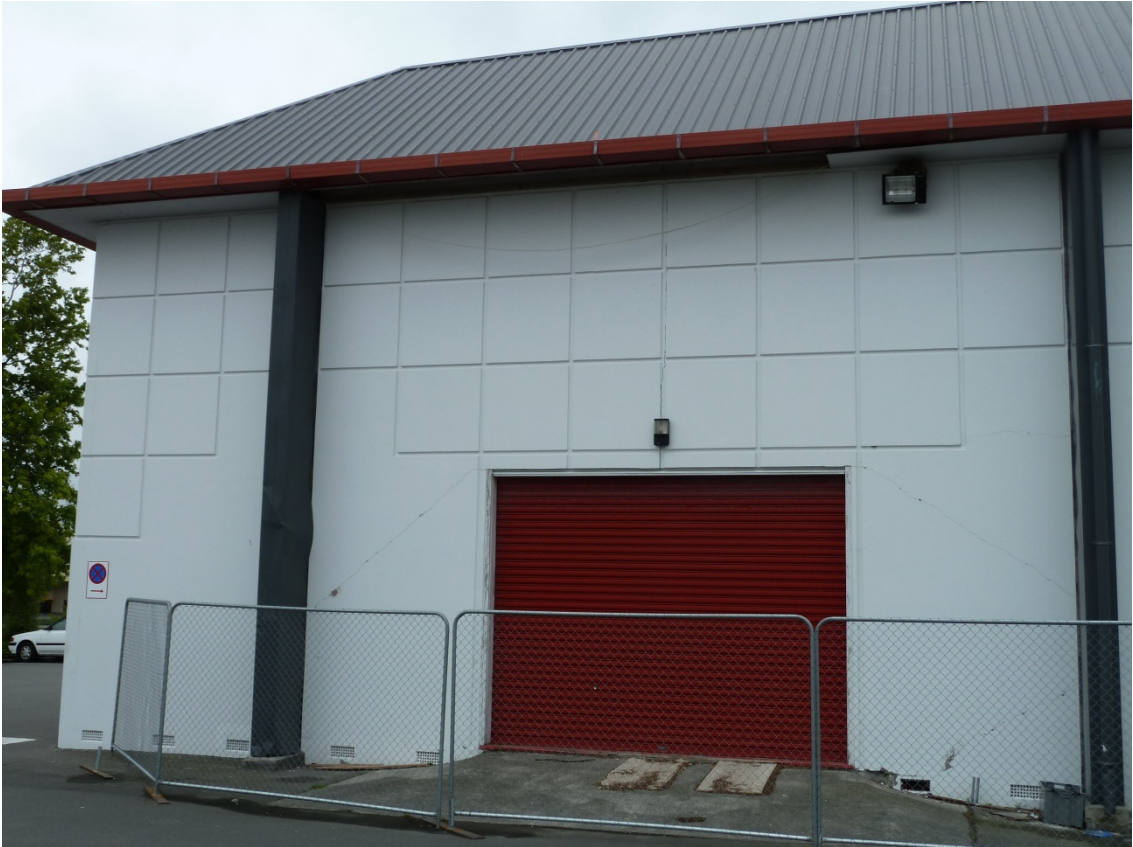
Photo 7 - South wall elevation
