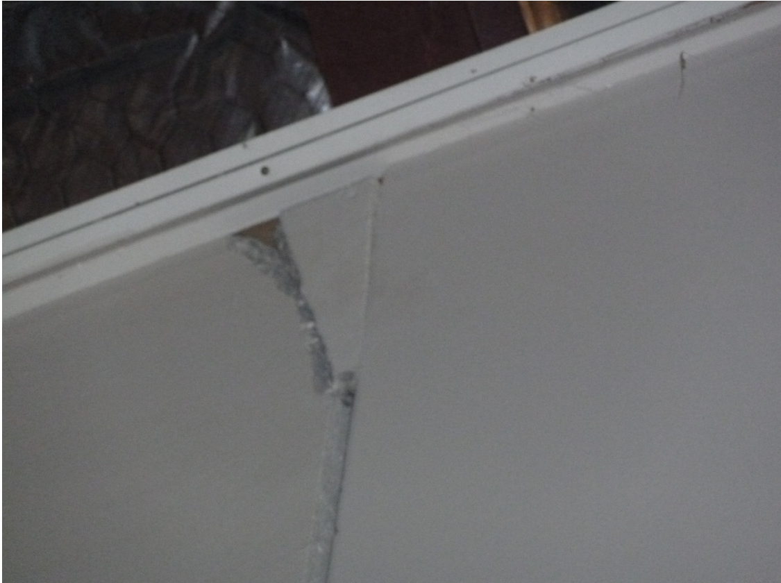
Photo 13: Cracking/Spalling at the top of the precast panel south wall, viewed internally to the east of the damaged panel shown previous
