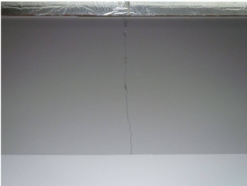
Photo 10 - Interior view of vertical crack on the south wall panel
