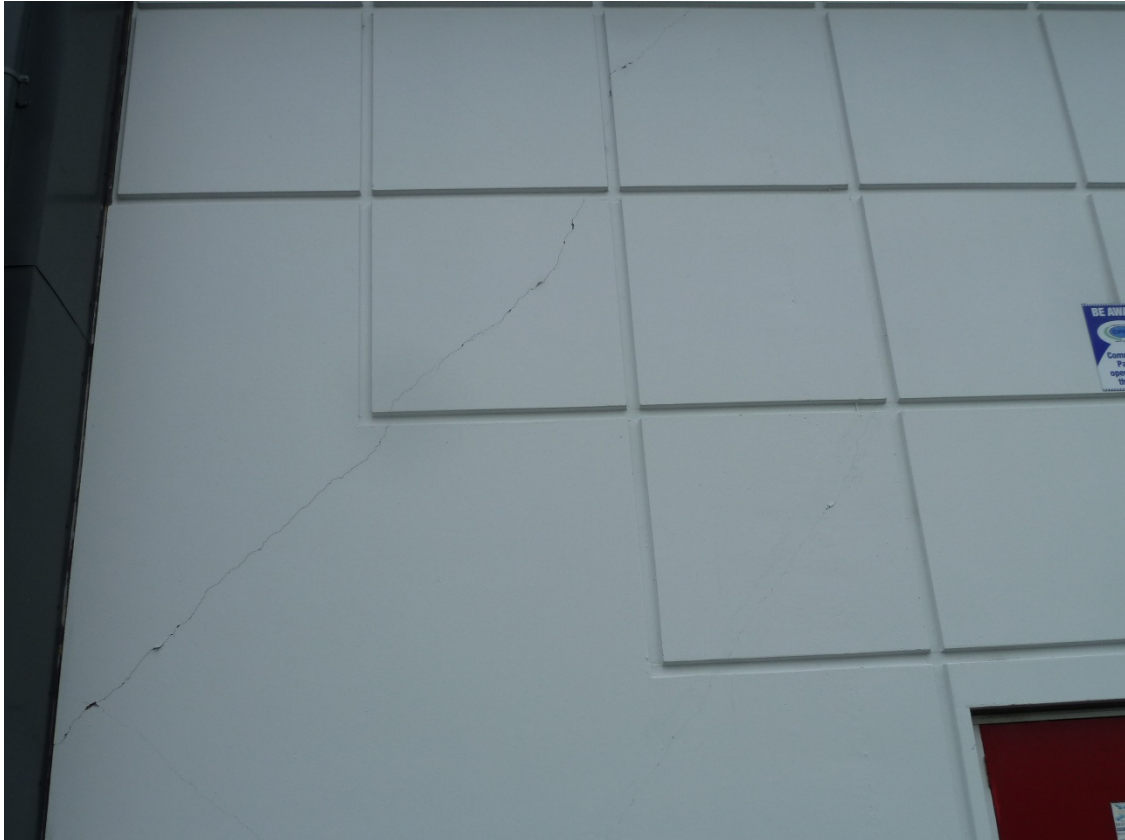
Photo 3 - Shear crack in west wall panel
