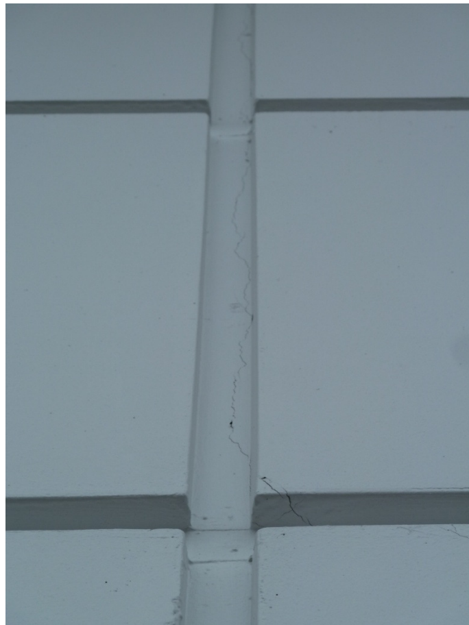
Photo 4 - Vertical crack in west wall panel
