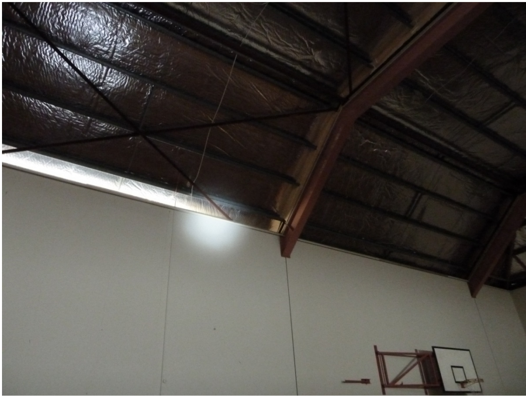
Photo 16 - Diagonal ties above west wall panel
