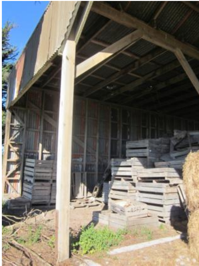
Photograph 4: View of interior at north end. Note braced eastern wall.
