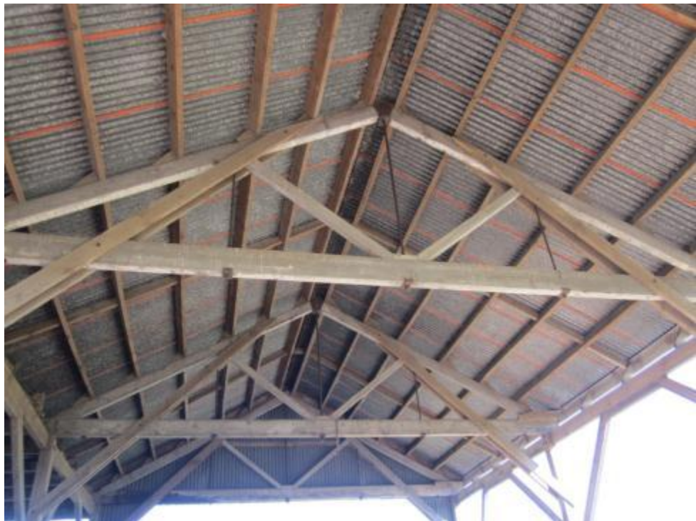
Photograph 6: Interior view of knee-braced timber and steel rod trusses.
