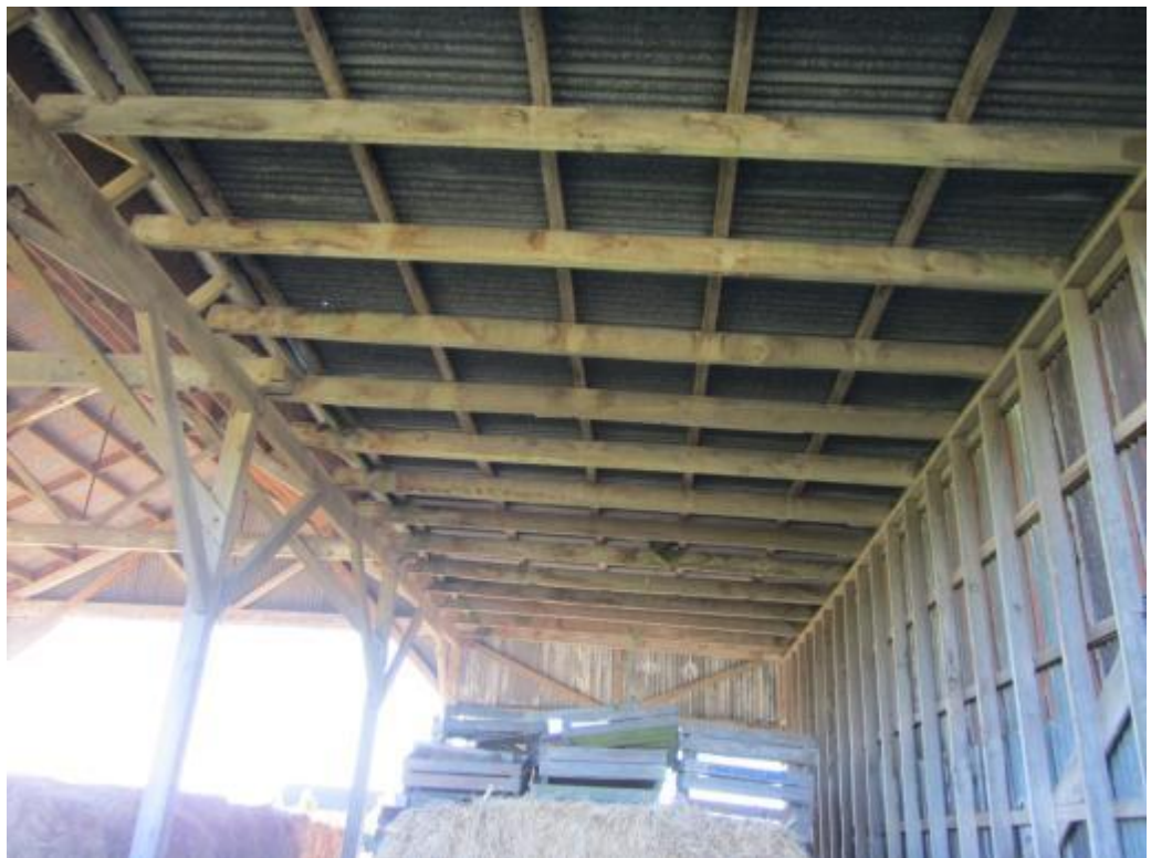
Photograph 8: Interior view of flat roof section.
