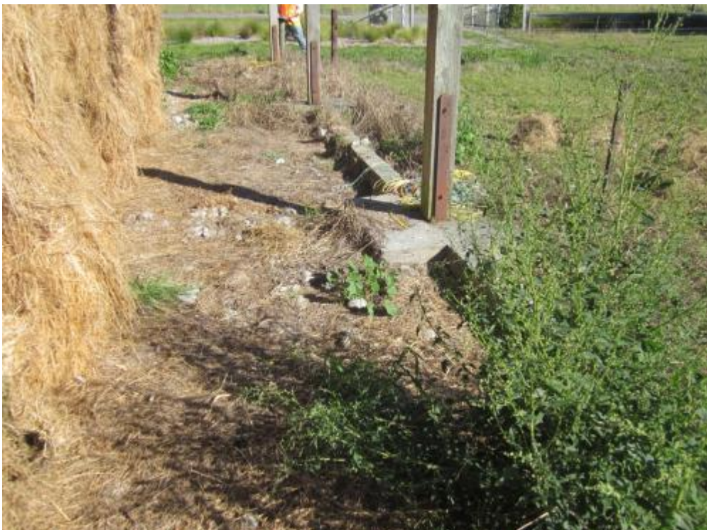
Photograph 10: Timber posts and pad foundations at western edge.
