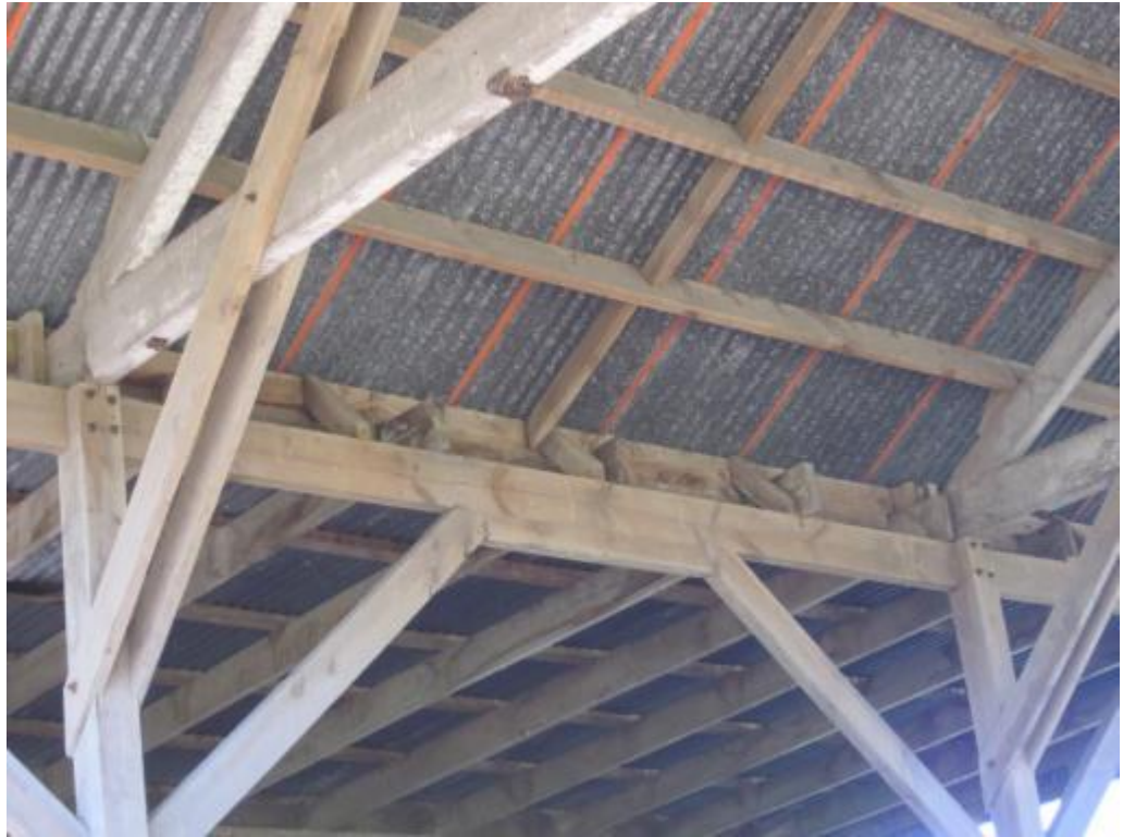
Photograph 7: Interior view of junction between flat and trussed roof sections.
