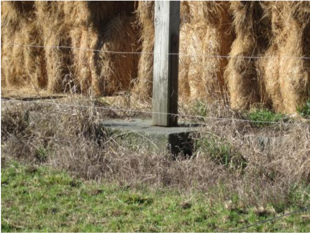
Photograph 9: Typical post and concrete pad.
