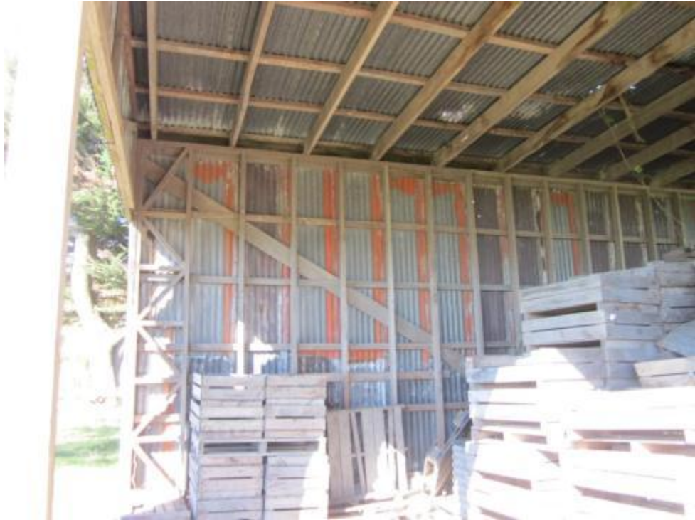
Photograph 5: Interior view of cross-braced east wall and timber roof members.
