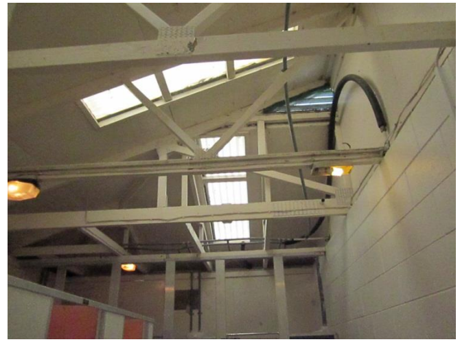
Timber purlins and pre-nailed trusses in the toilet block addition.
