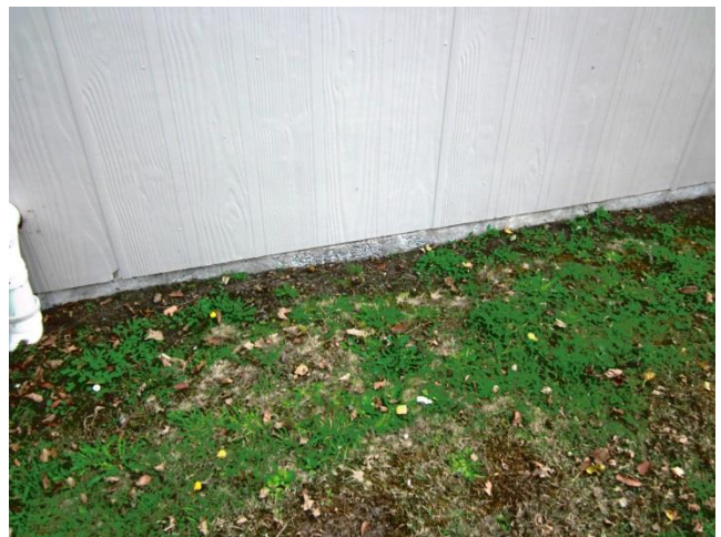
Vertical cement sheet boards and concrete slab below.
