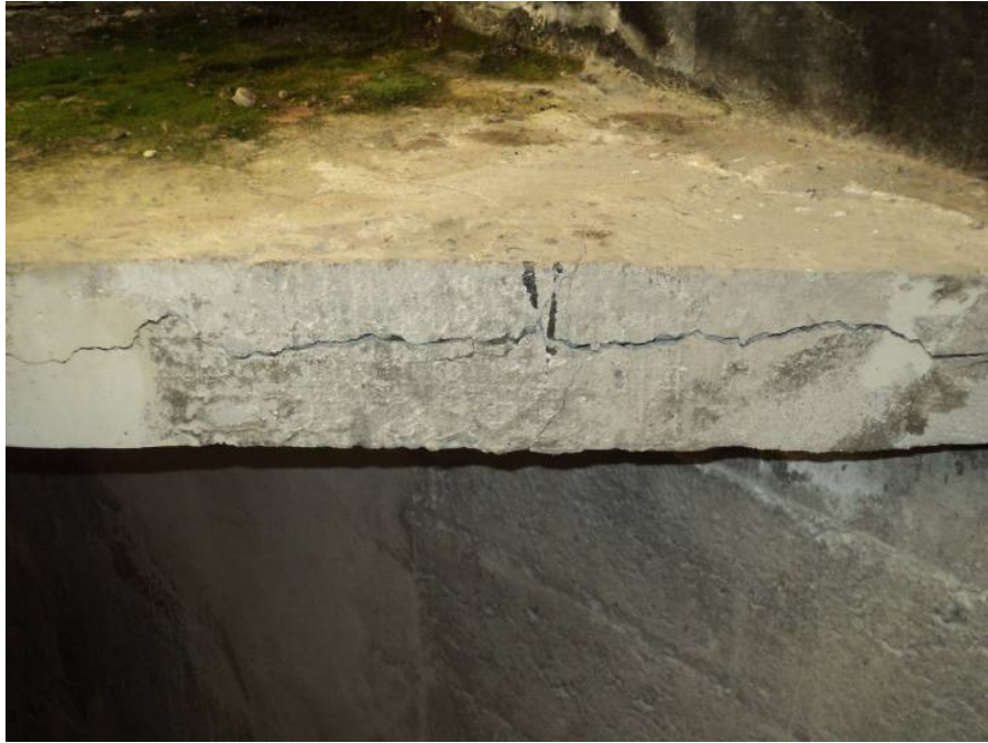
Figure 7e – Crack in concrete slab at 1 st floor
