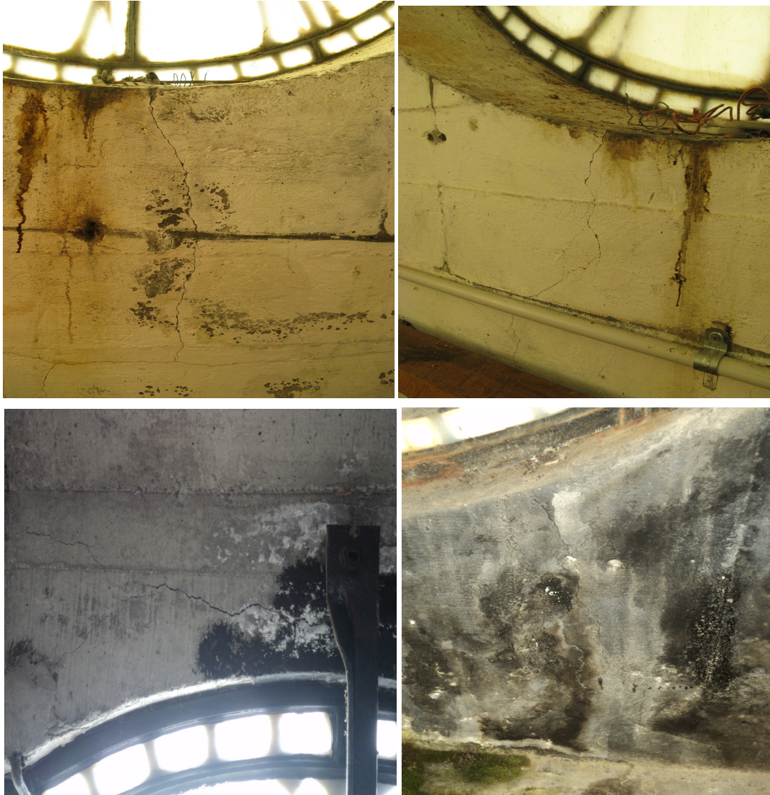
Figure 7b – Interior of the north and East faces showing the vertical cracks and moisture inside the clock tower
