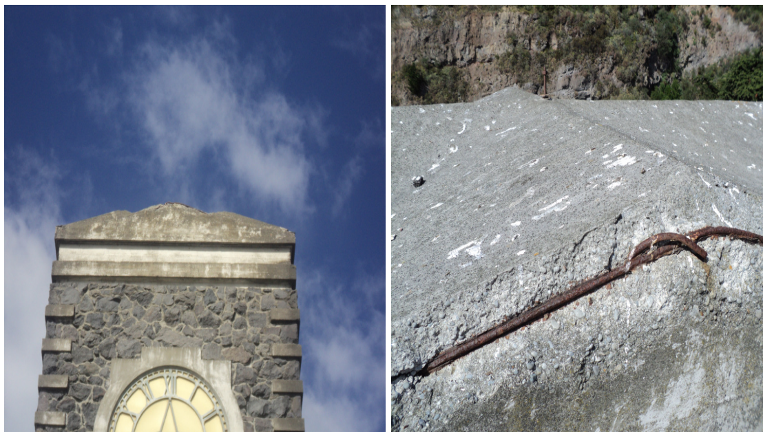
Figure 7d – Concrete spalling at the roof
