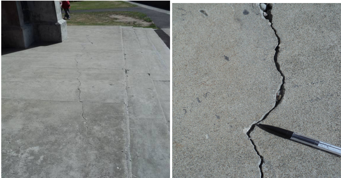
Figure 7c – Cracks around the slab around the perimeter of the tower
