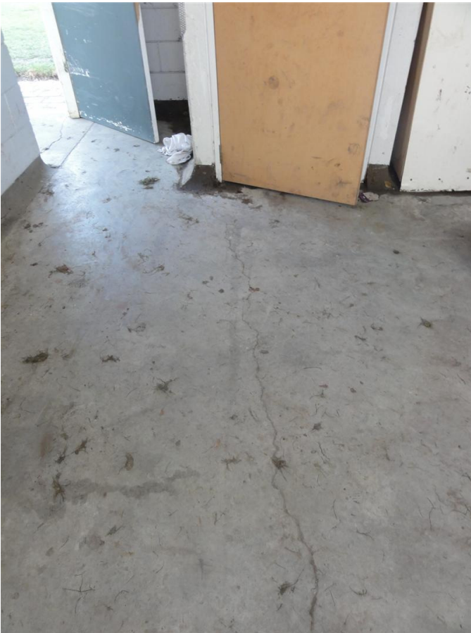
Photograph 8. Hairline crack along concrete slab in changing rooms.
