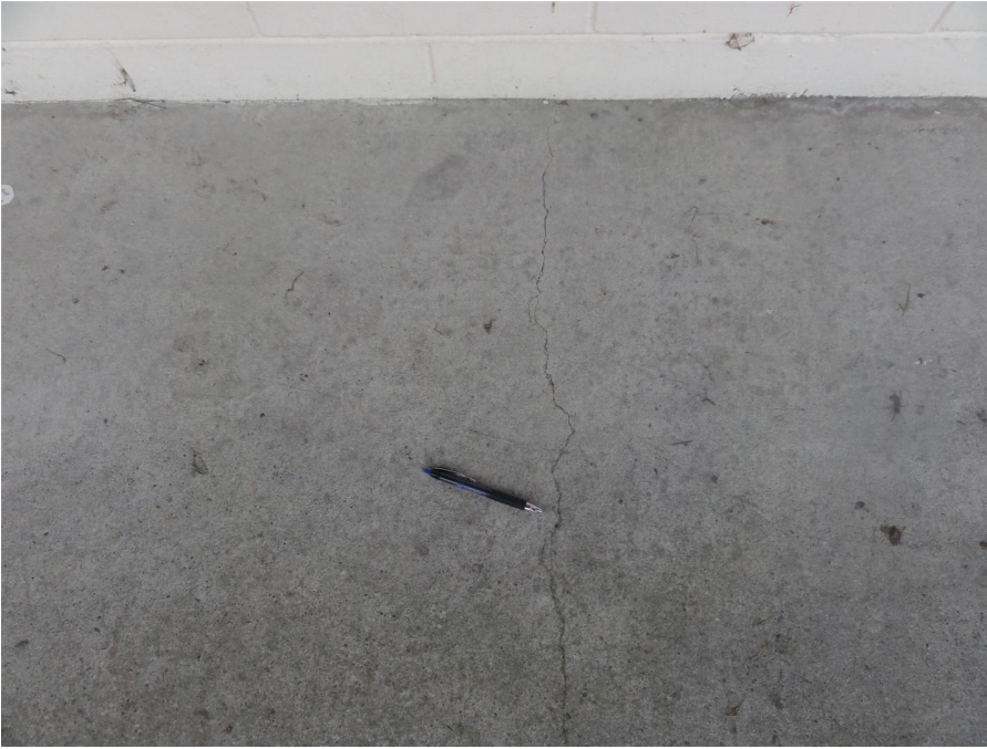
Photograph 7. Typical hairline crack through concrete slab along raised patio.
