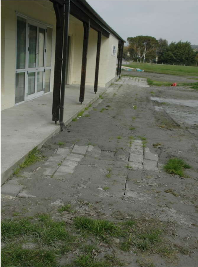
Photograph 3. View along western wall, showing ejected silts and sands.
