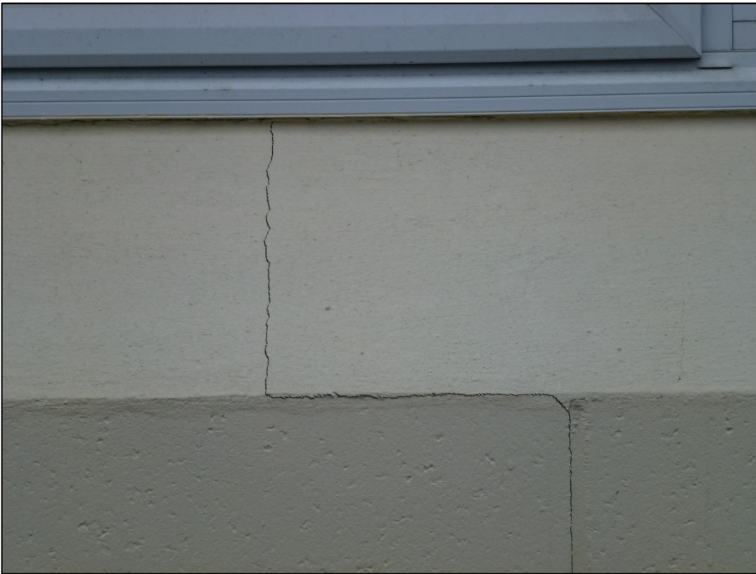
Photo 11: Cracking of sill below window opening.
