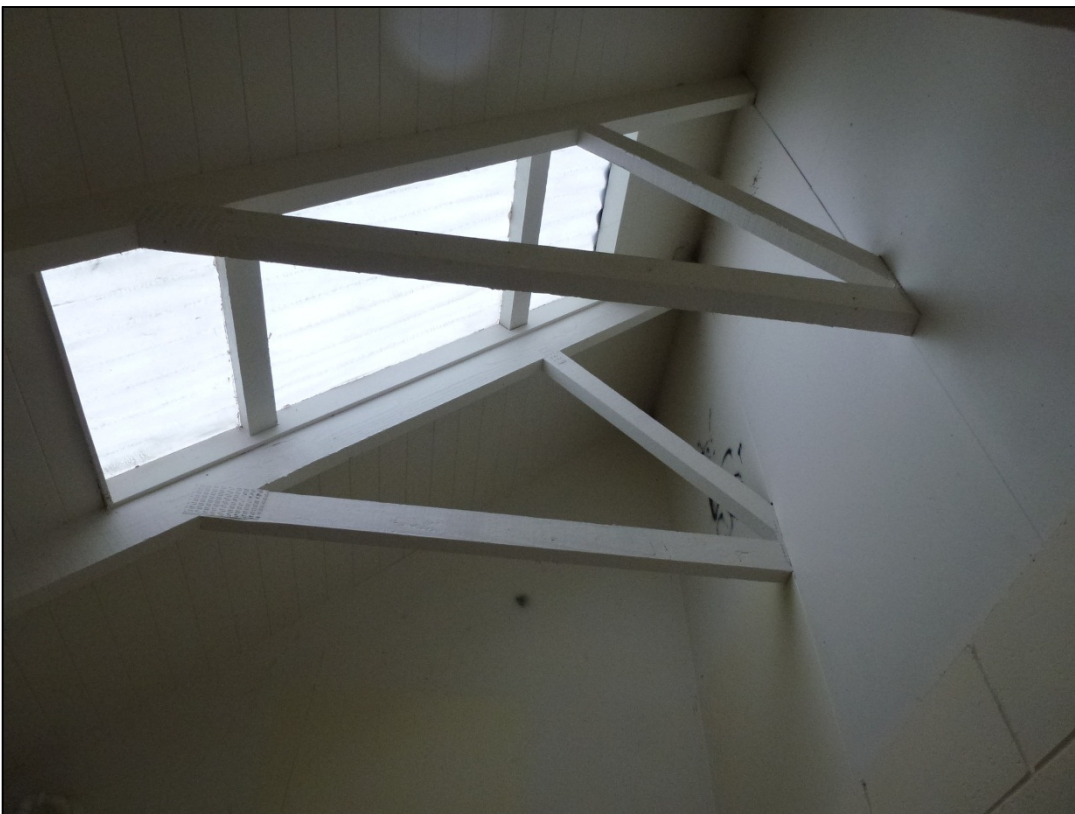
Photo 4: Typical view of roof truss in toilet area.
