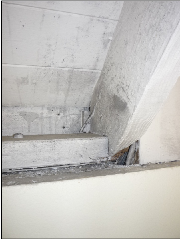
Photo 5: Typical truss connection to top plate.
