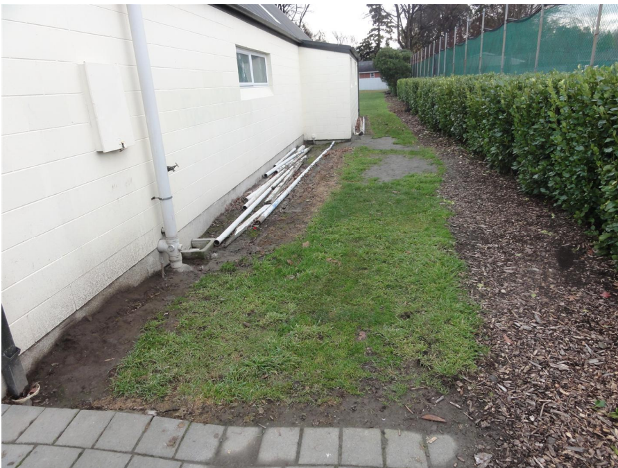
Photograph 4. View along eastern wall, showing ejected silts and sands.
