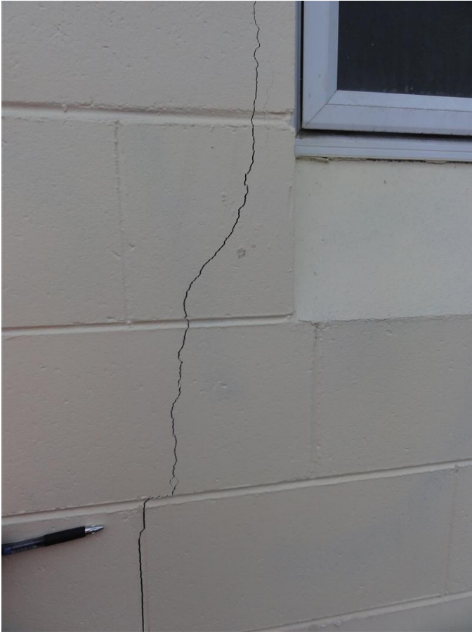
Photograph 5. 1.5mm wide crack in eastern external concrete block work.
