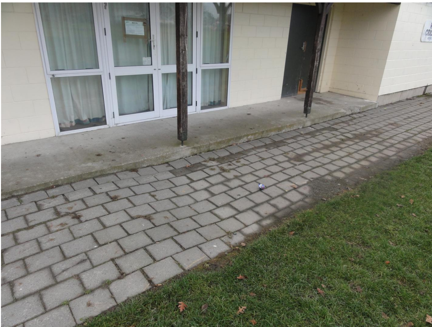
Photograph 6. Approximately 70mm heave of the pavers adjacent to the raised patio (western side of pavilion).
