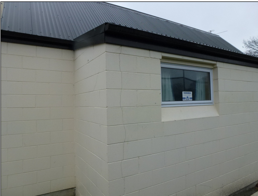
Photo 10: Vertical cracks on eastern wall (approx. 1.5mm wide).
