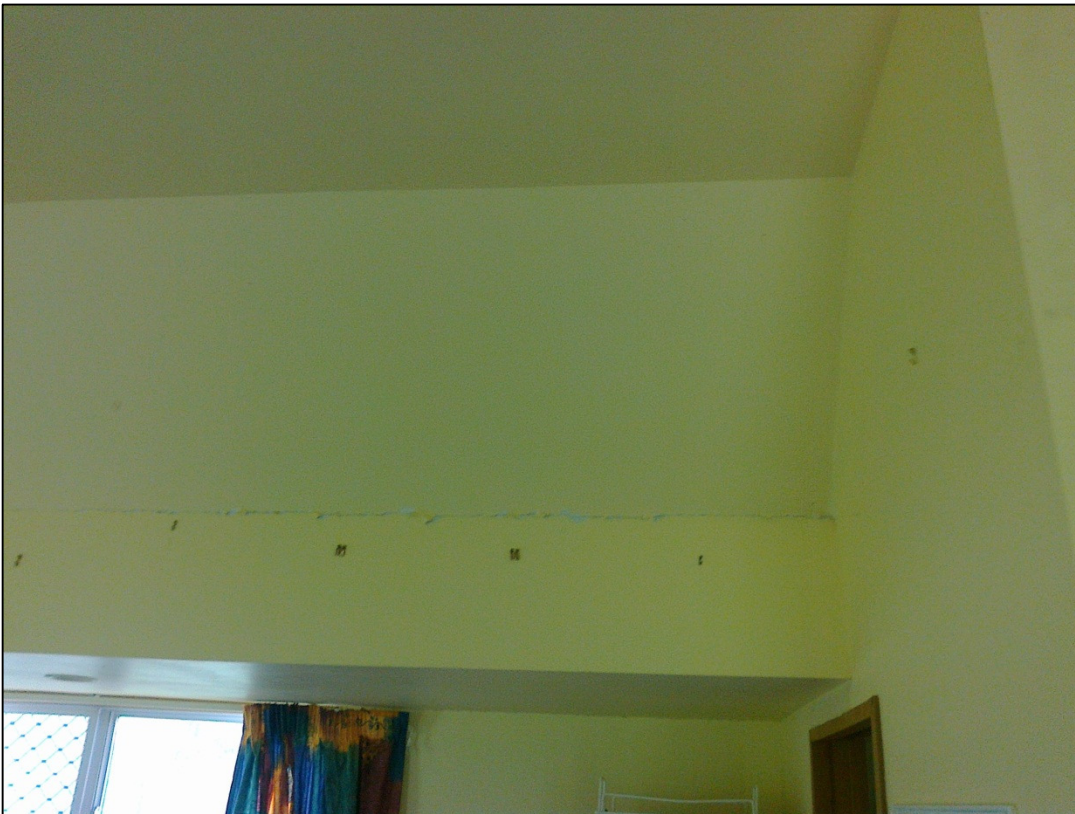
Photo 8: Cracking of ceiling seam.
