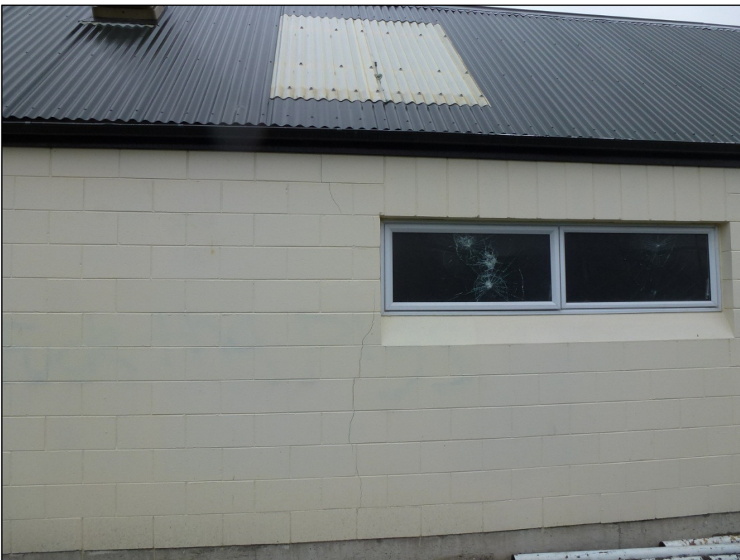
Photo 12: Vertical crack on wall.
