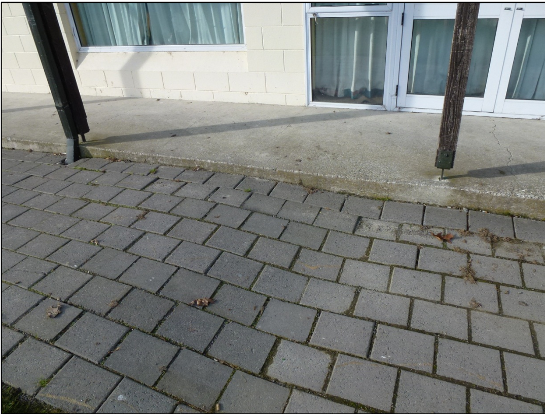
Photo 9: Cracks on slab on western side. Note settlement of paving due to liquefaction.
