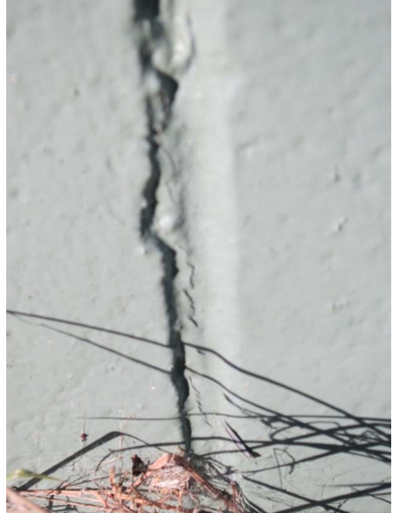
Photo 14: Cracking along mortar joints on west wall.
