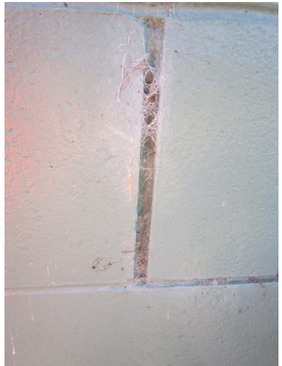
Photo 20: Existing low quality pointing of mortar on south wall.
