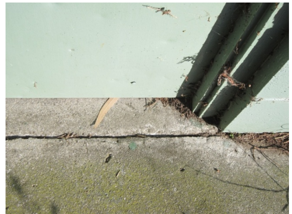
Photo 10: Gap opening up between low masonry wall and main north building wall.
