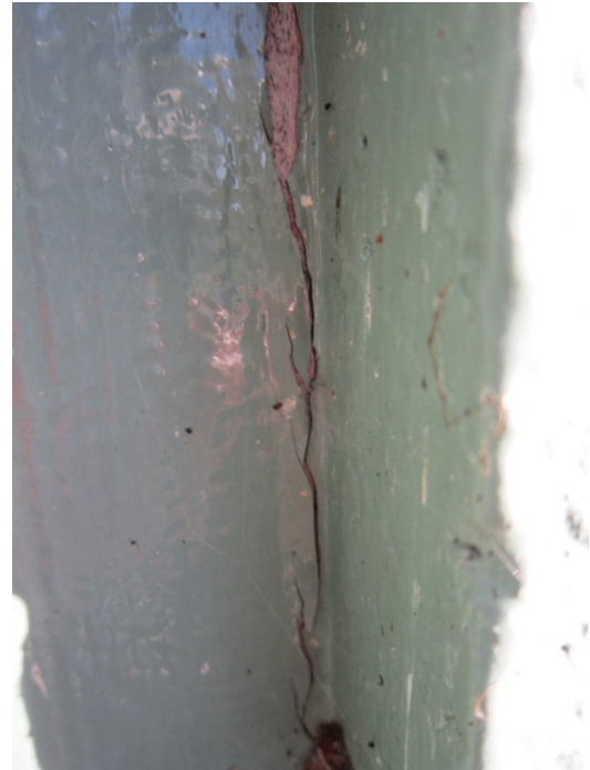
Photo 10: Gap opening up between low masonry wall and main north building wall.
