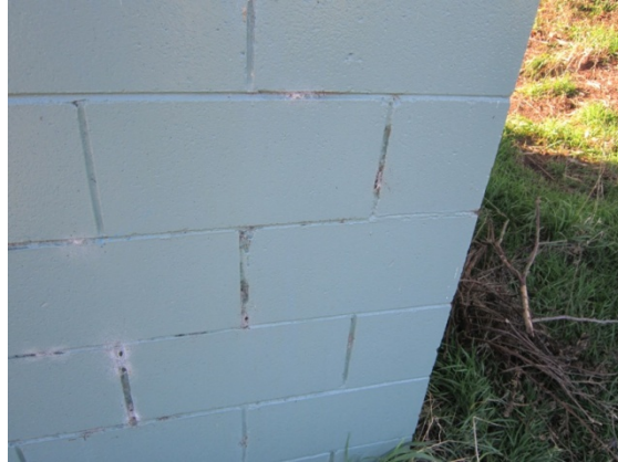
Photo 21: Existing low quality pointing of mortar on south wall.
