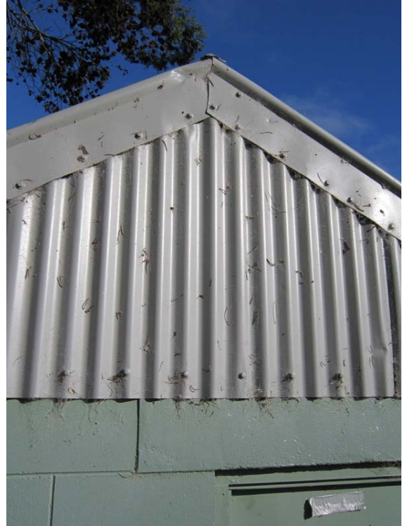
Photo 6: Corrugated steel roof cladding.
