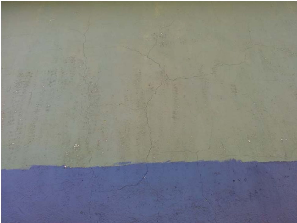
■ Figure 10 - Observed cracks in the wall
