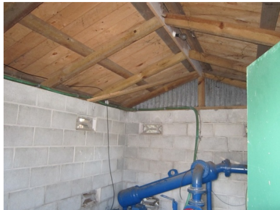
Photo 23: Interior of east pumphouse, indicative of timber-framed roof in west pumphouse.
