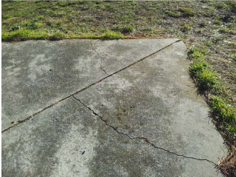
■ Figure 11 - Cracking in external concrete ground slab
