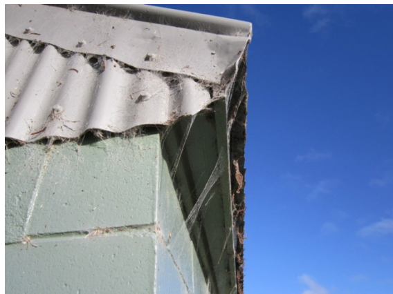
Photo 7: Corrugated steel roof cladding.
