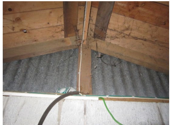
Photo 24: Interior of east pumphouse, indicative of timber-framed roof in west pumphouse.
