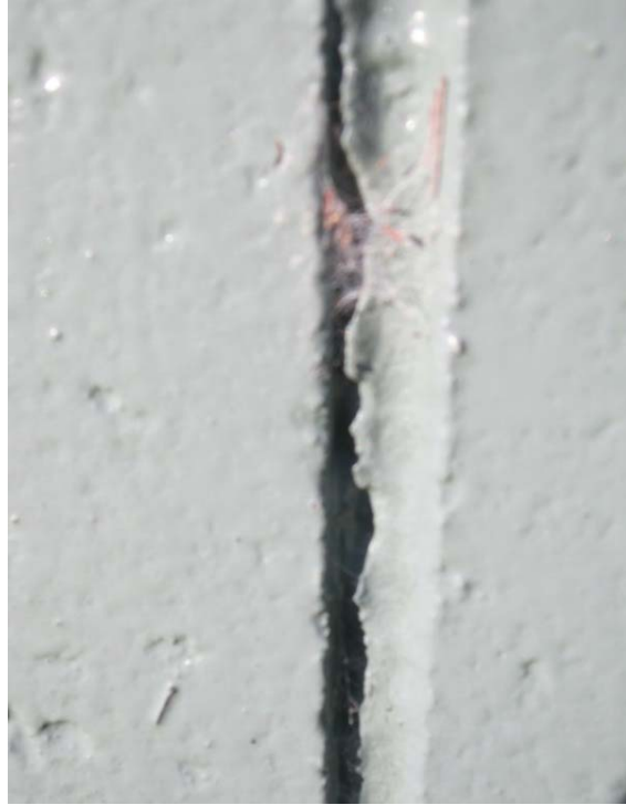
Photo 13: Cracking along mortar joints on west wall.
