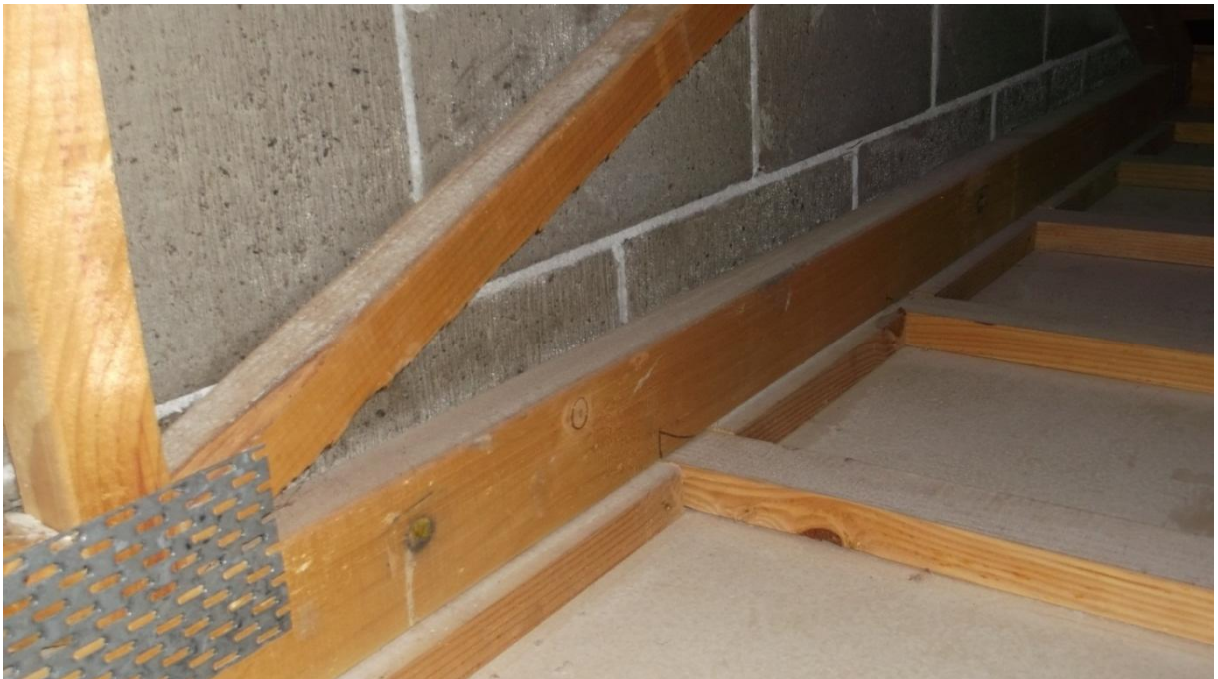
Photograph 12: Roof space, showing end blockwork wall and end timber roof truss
