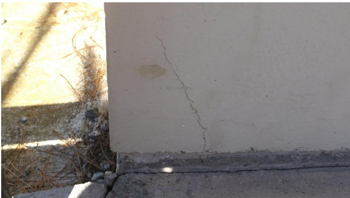
Photograph 6: Close up of crack through bottom concrete block
