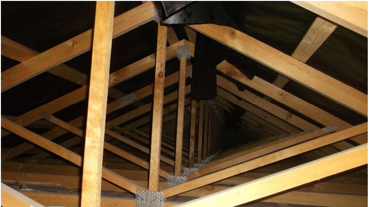
Photograph 11: Roof space, showing timber roof trusses and purlins
