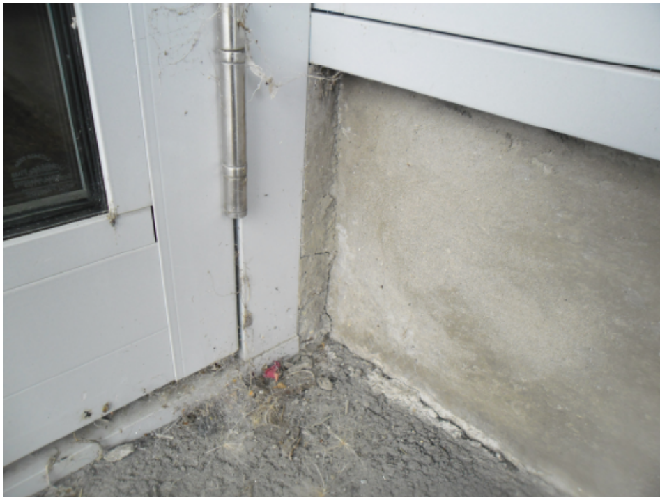
Observed Damage: Minor cracking to base of foundation slab potentially due to lateral spread or other ground movement such as liquefaction
