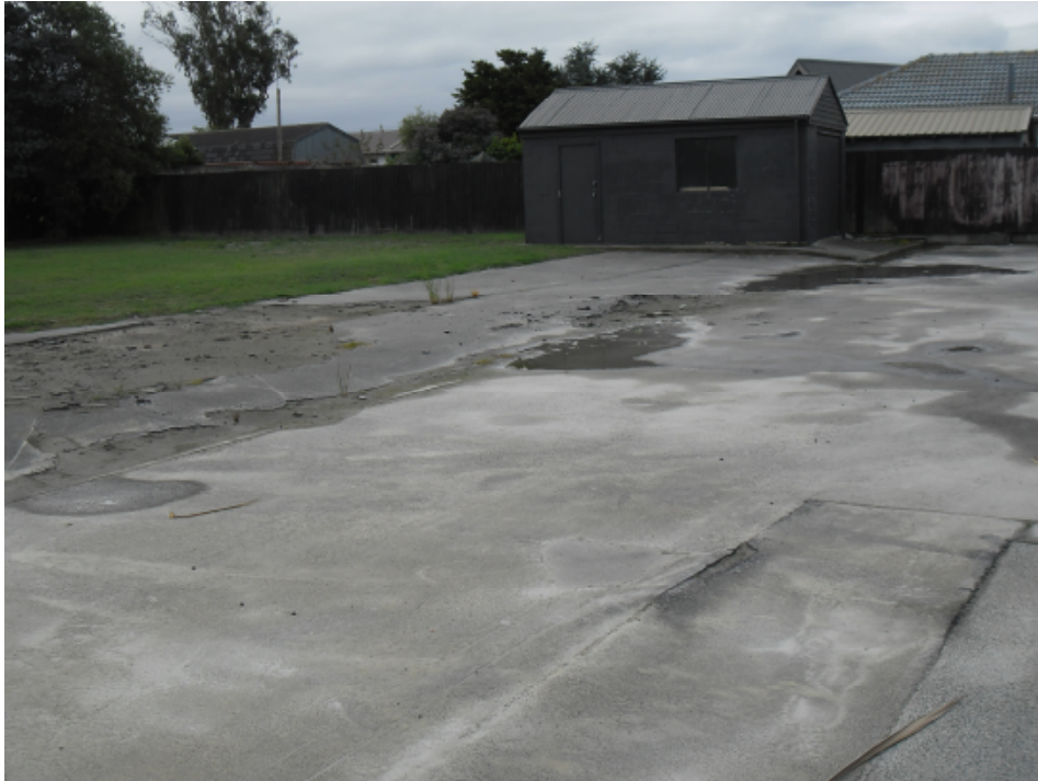
Observed Damage: Liquefaction in adjacent parking area
