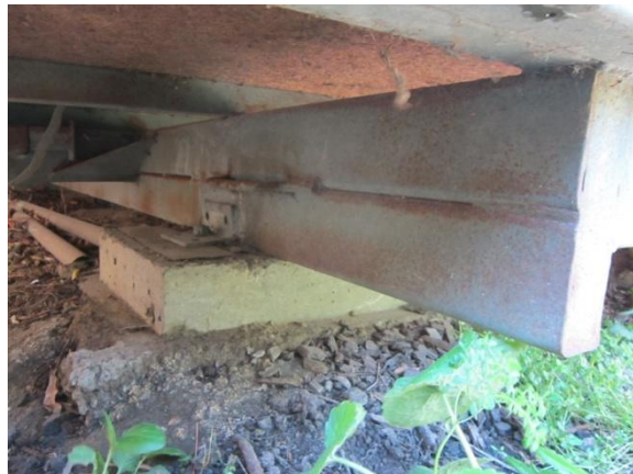
Photo 7: Foundation system showing rust on steel beam (typical)
