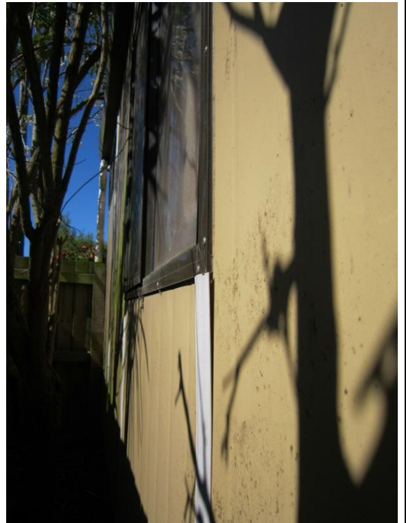
Photo 6: Gaps opening up between wall cladding elements
