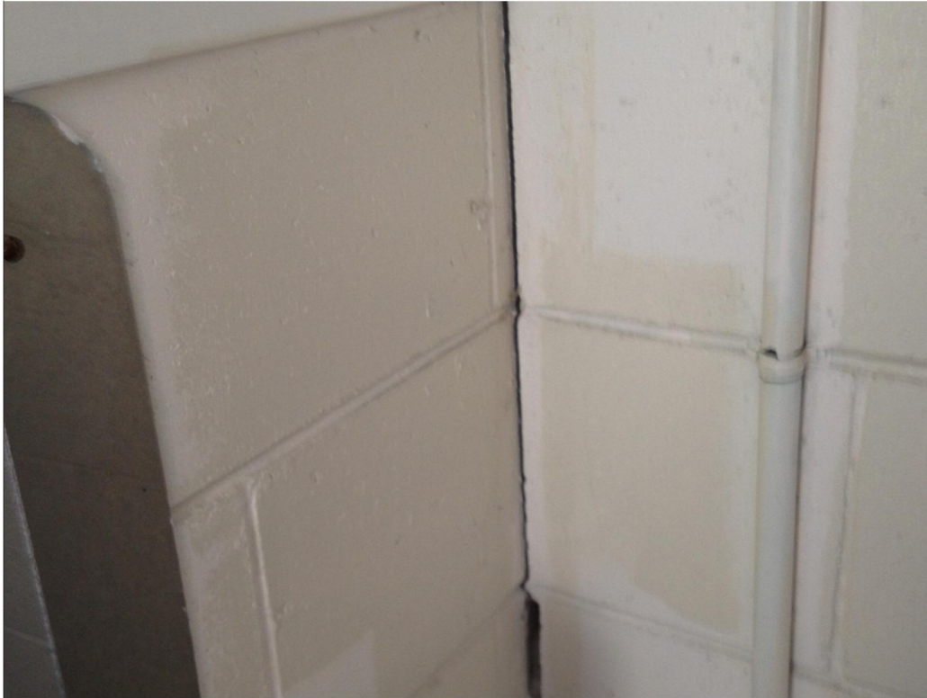
Photo 3: Adjacent internal walls.
