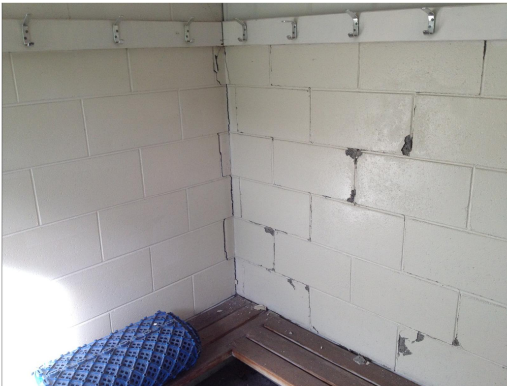
Photo 4: Change room internal walls.
