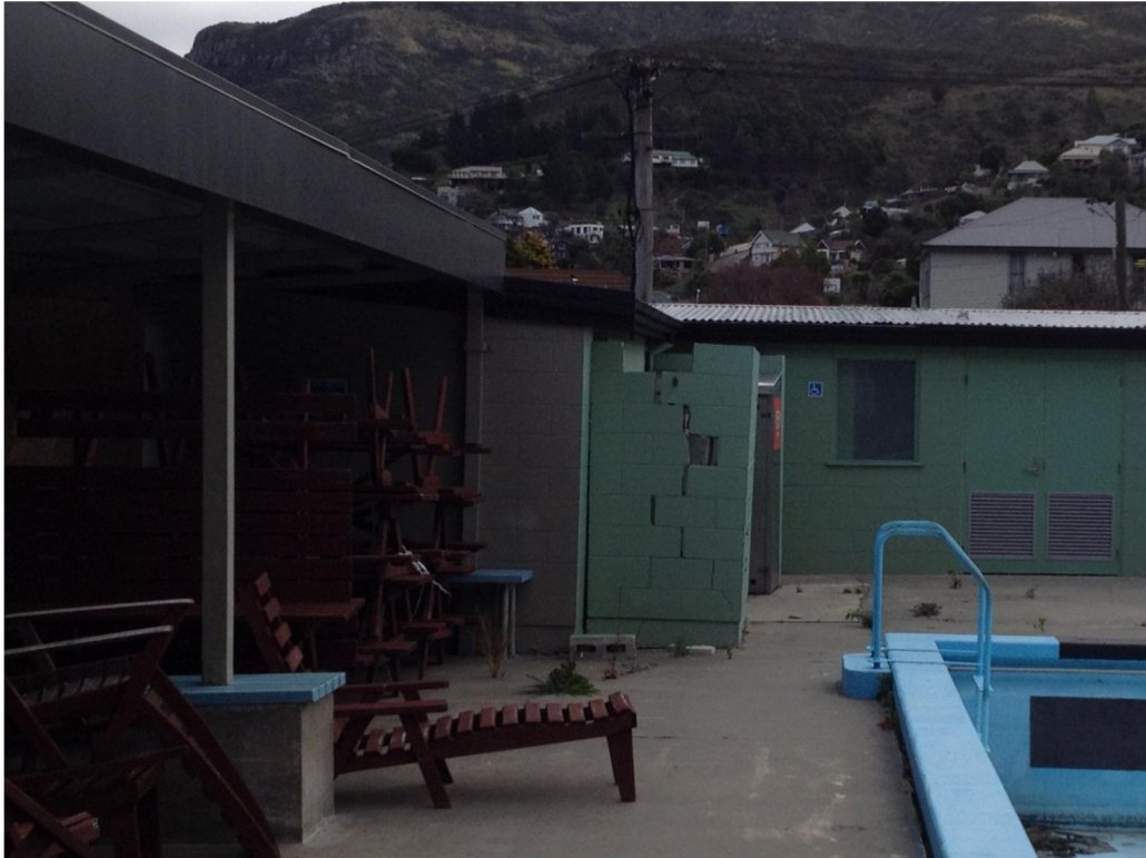
Photo 1: External view of the Ladies' Change Room (view from east).
