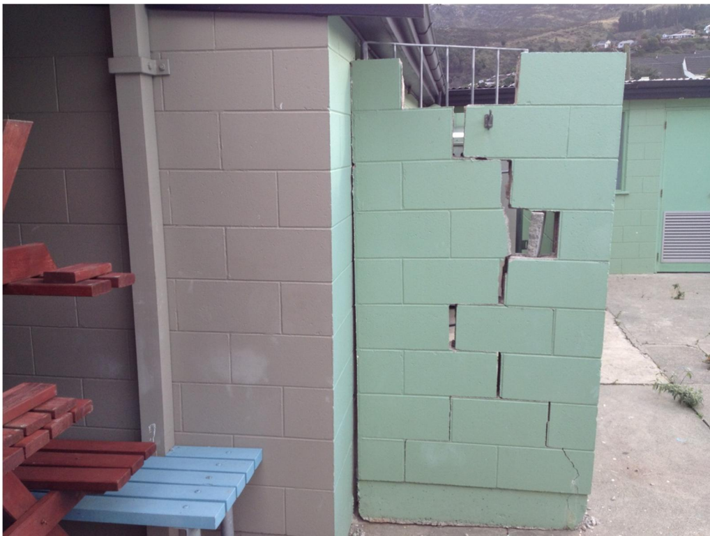
Photo 2: Entrance privacy wall of Ladies' Change Room.
