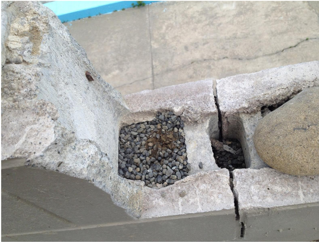
Photo 11: Concrete masonry fence to the north of the pool.
