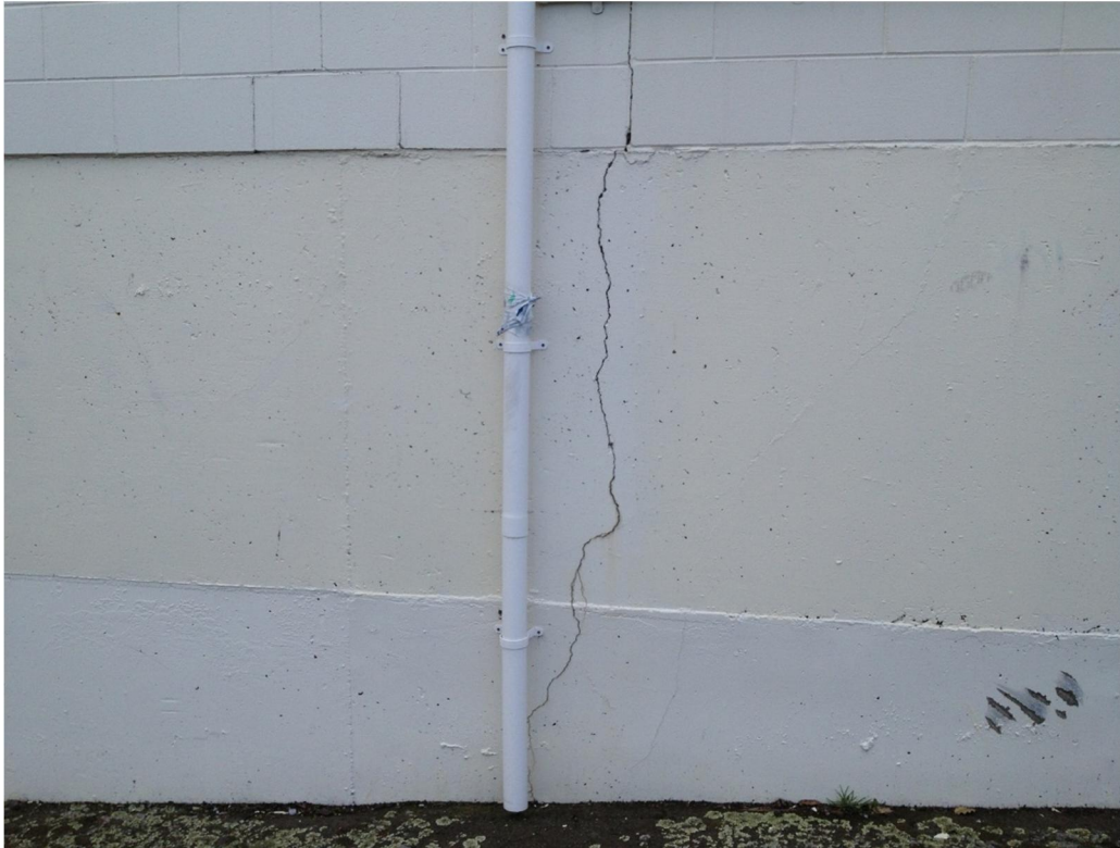
Photo 7: Concrete retaining wall on southern side of Ladies' Change Room. Damage Description: Cracking of concrete retaining wall and concrete masonry mortar.
