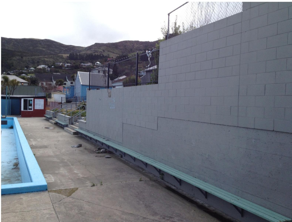
Photo 10: Concrete retaining wall and concrete masonry block fence to the north of the pool (view from south-east). Damage Description: Cracking and differential settlement of concrete masonry block wall.
