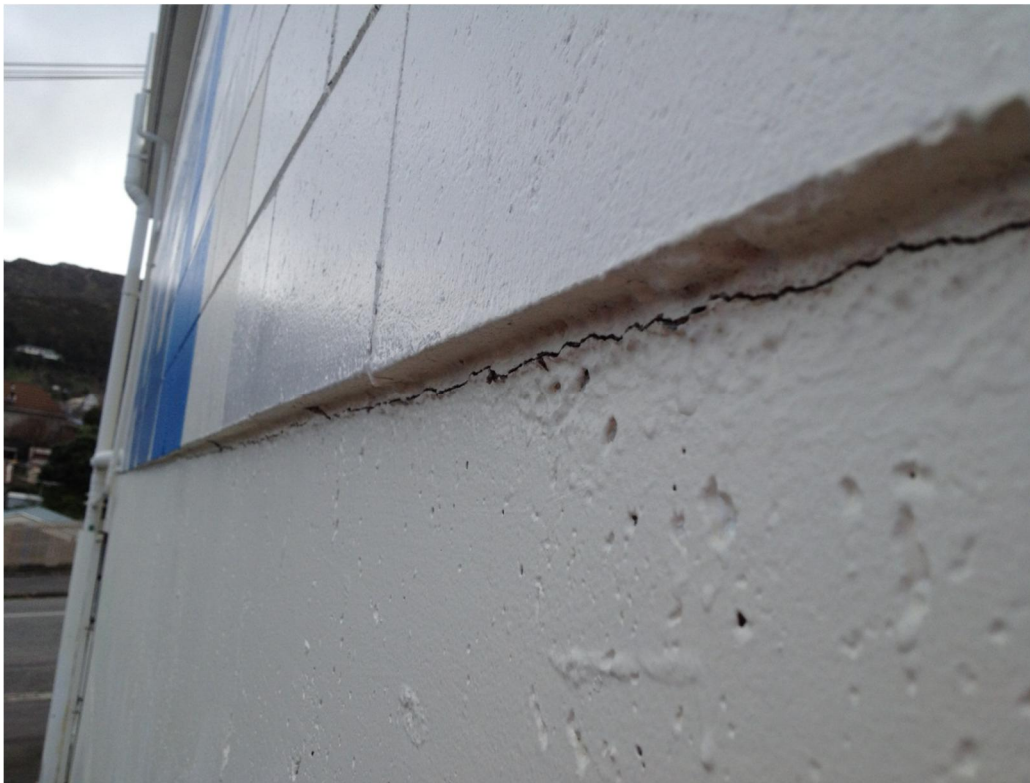
Photo 8: Junction between concrete retaining wall and concrete masonry block wall. Damage Description: Cracking between masonry and concrete retaining wall on southern side.
