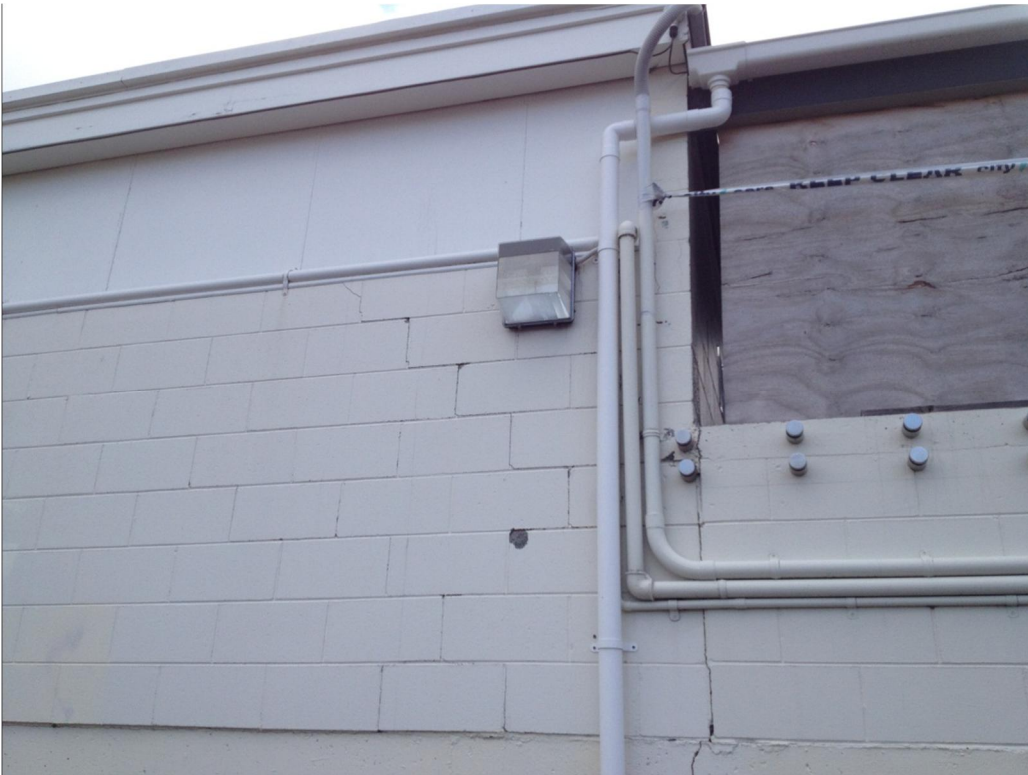
Photo 6: Southern concrete masonry block wall.
