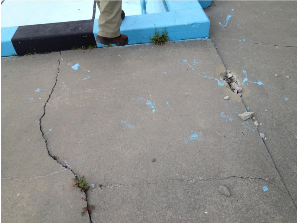
Photo 9: Pavement near Ladies' Change Room. Damage Description: Cracking in concrete pavement.
