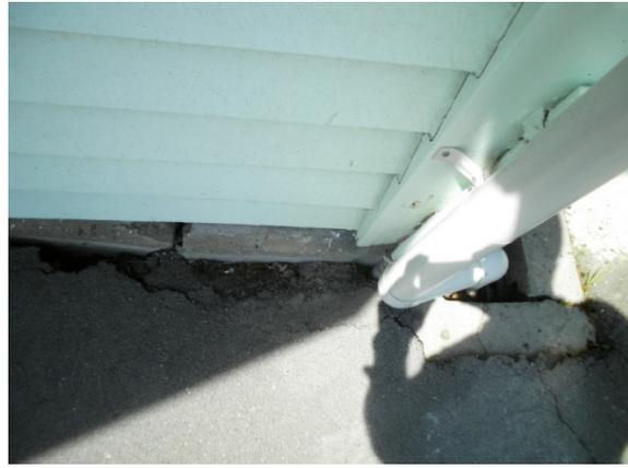
Horizontal crack in perimeter footing
