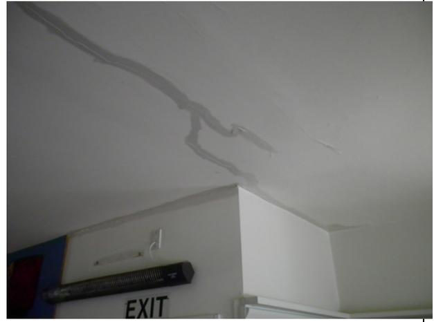
Vertical crack in wall above door opening.
