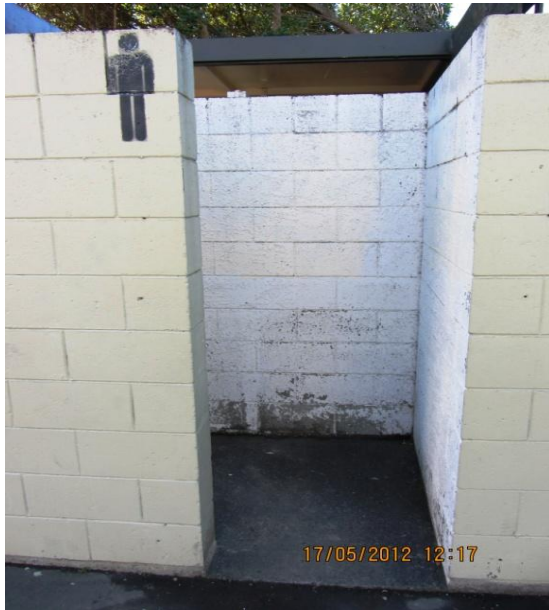
Photo 13: Men's toilet entrance
