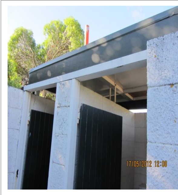
Photo 9: View of roof
