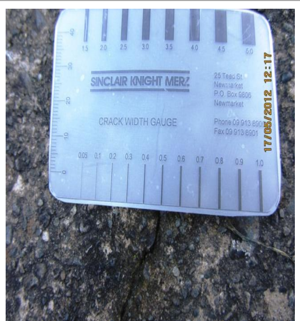
Photo 12: Close up view of photo 11 showing 0.5mm crack
