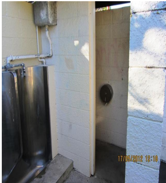
Photo 15: Men's toilet showing urinals and cubicle
