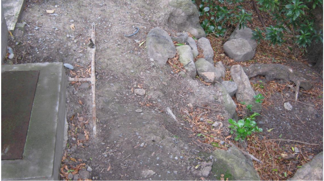
■ Figure 8 Failed dry stack garden wall behind the toilet block
