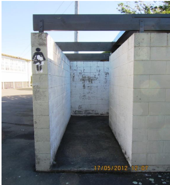
Photo 5: Entrance to women's toilet
