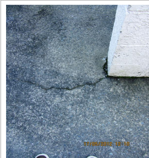
Photo 11: Crack in pavement in women's toilet
