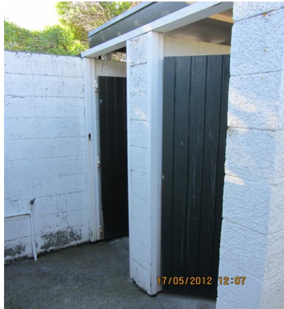
Photo 7: Women's toilet cubicle
