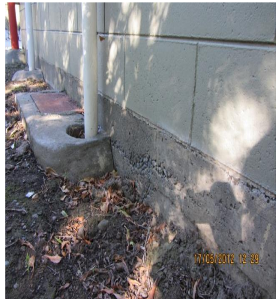
Photo 16: North east elevation showing 250mm of foundation slab above ground
