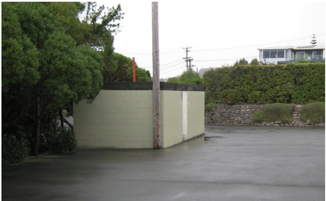
■ Figure 6 Toilet block at Old School Reserve.
