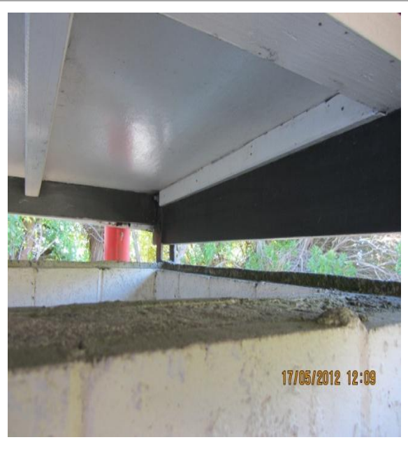
Photo 10: Timber roof showing filled masonry
