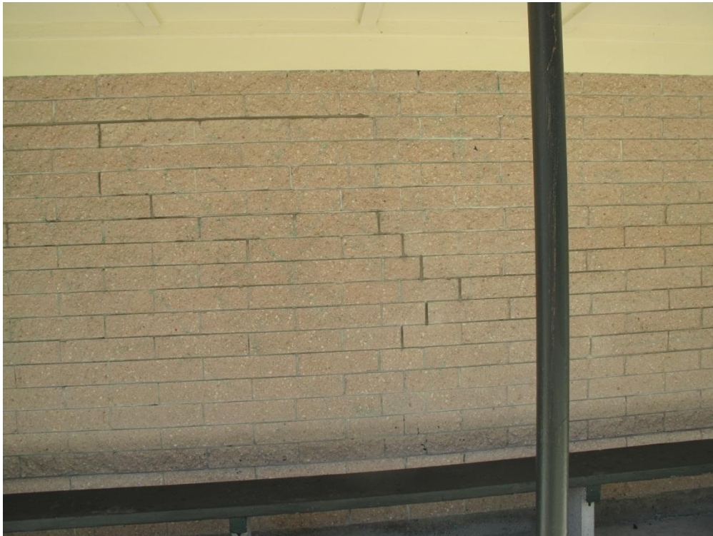
Photograph 7 Repairs to damaged mortar in the brick masonry walls.
