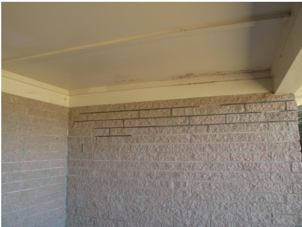
Photograph 5 Differential settlement of the concrete foundation slab.
