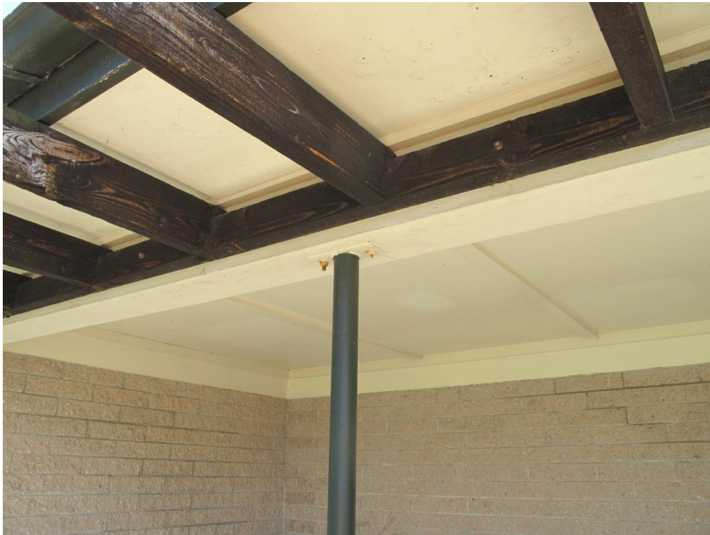
Photograph 9 Concrete bond beam at the top of the wall and perimeter of the roof..
