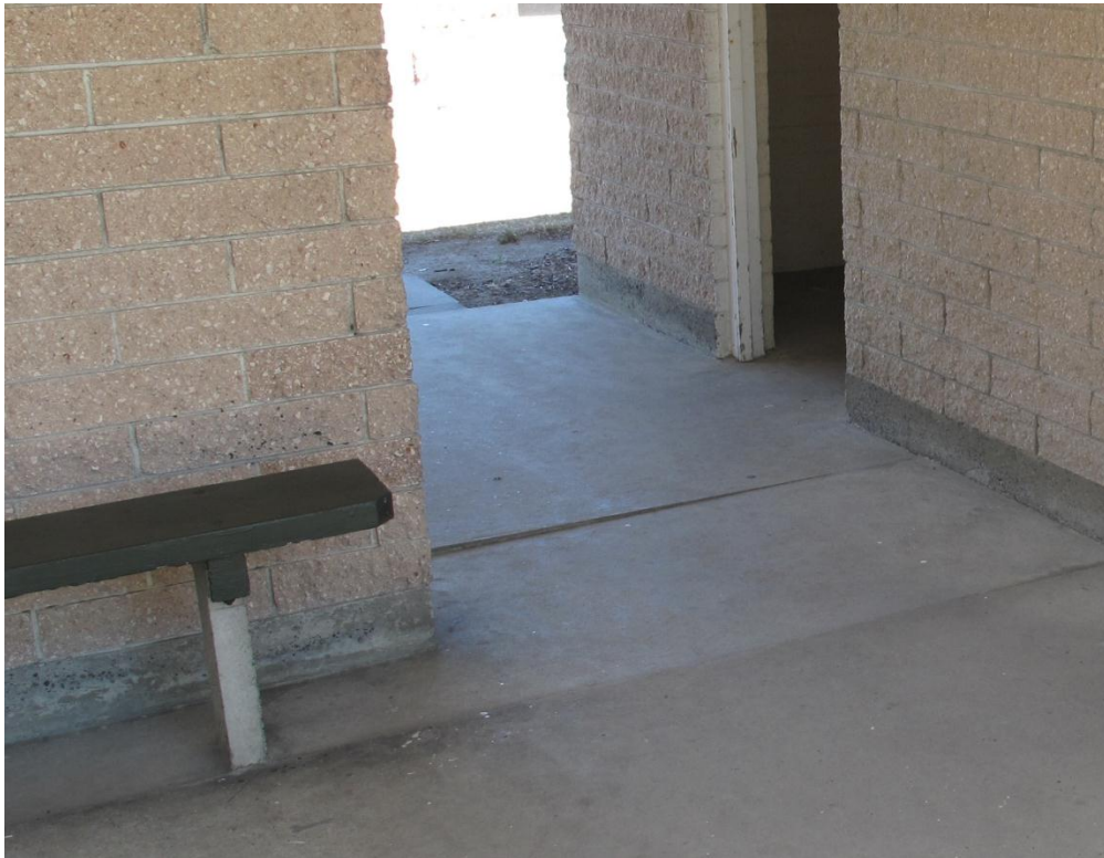
Photograph 5 Differential settlement of the concrete foundation slab.
