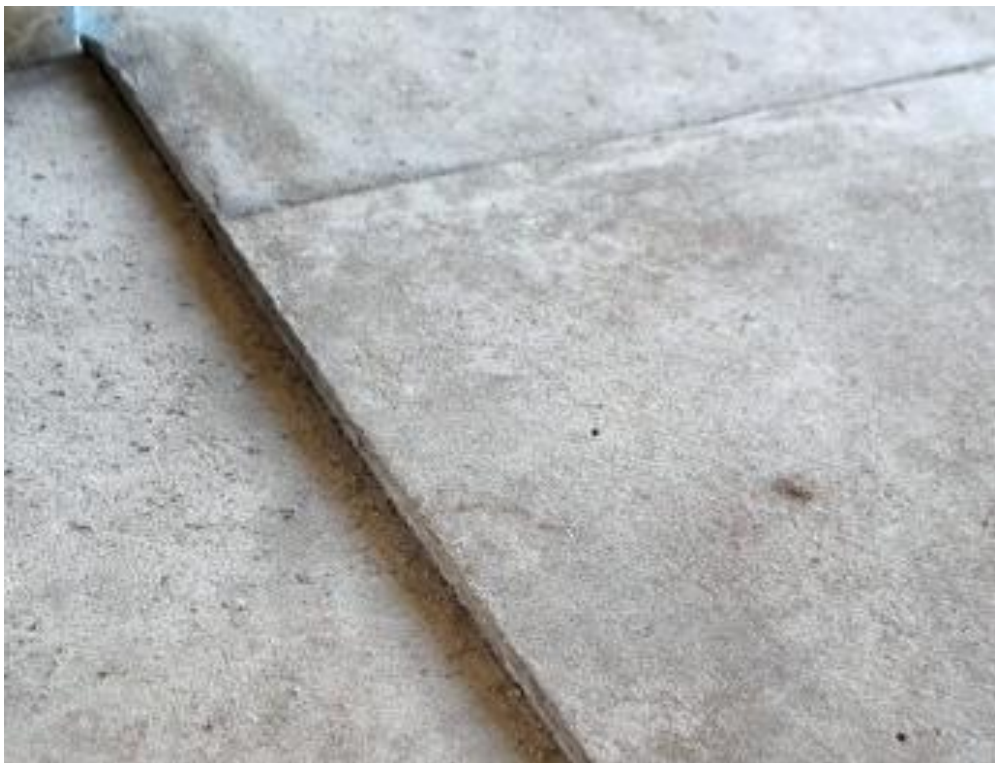
Photograph 4 Differential settlement of the concrete foundation slab.
