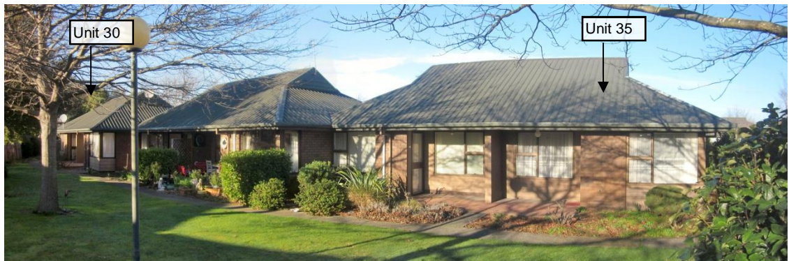
PHOTO 2: Maurice Carter Court Owner/Occupier Units – Exterior rear view of the property from North-East. The apartment units 30-35 (from left to right).
