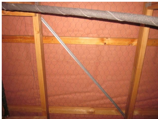
PHOTO 15: Maurice Carter Court Owner/Occupier Units – Interior view of roof space above Unit 30.
