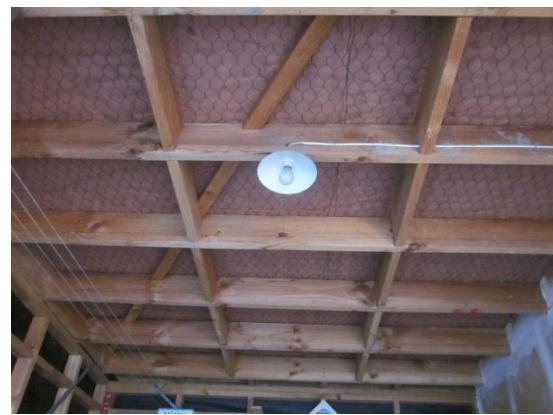
PHOTO 18: Garage 1 – Roof timber bracing
