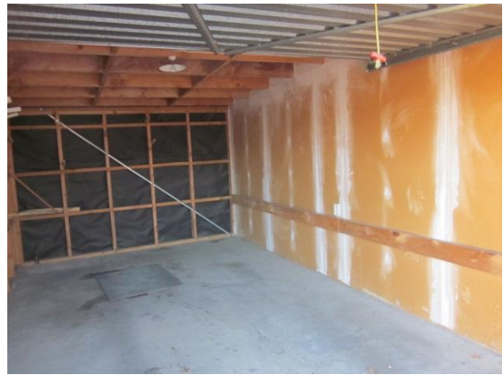
PHOTO 26: Garage 3 – Interior view (partition wall to the right)
