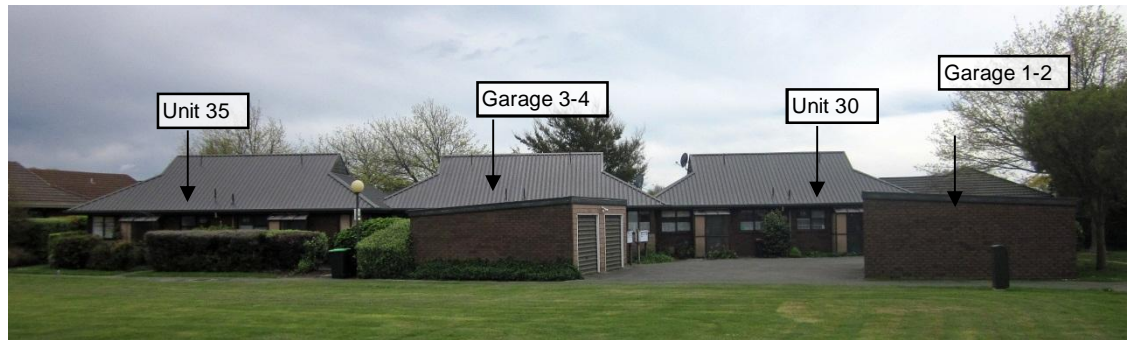
PHOTO 1: Maurice Carter Court Owner/Occupier – Exterior front view of the property from south-west. Two garage buildings to the front, apartment units 30-35 (from right to left) to the rear.
