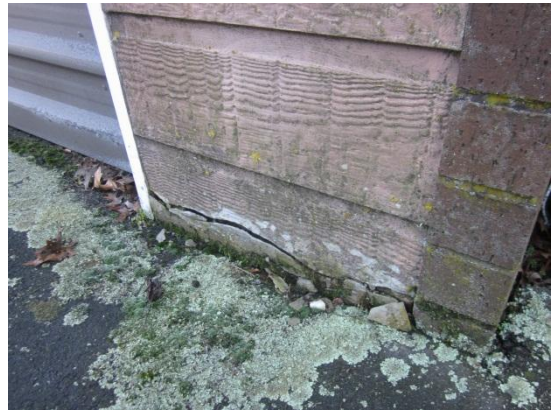
PHOTO 28: Garage 4 – Cracked hardies to the bottom of the front elevation (possibly earthquake damage)
