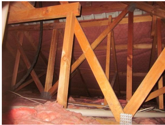
PHOTO 11: Maurice Carter Court Owner/Occupier Units – Interior view of roof space above Unit 30 towards east
