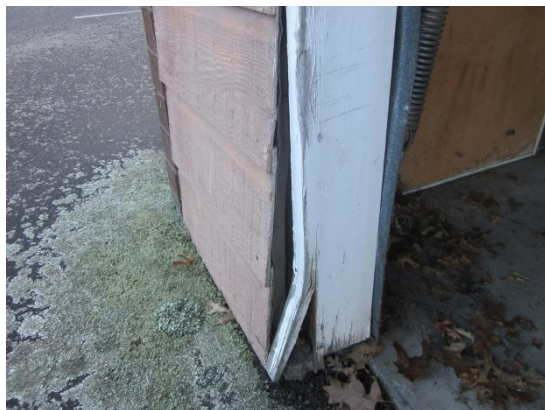
PHOTO 23: Garage 1 – Damage to door frame (not earthquake related)
