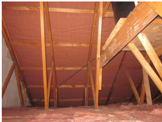
PHOTO 13: Maurice Carter Court Owner/Occupier Units – Interior view of roof space above Unit 30 towards north
