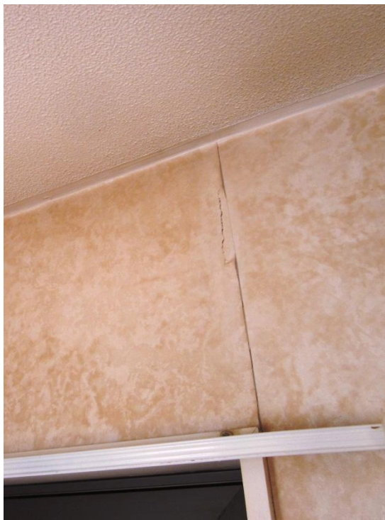
PHOTO 9: Detail of previous photo (probably earthquake damage)
