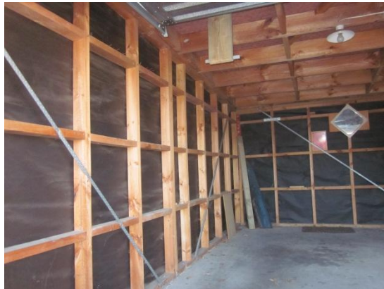
PHOTO 21: Garage 1 – Interior view
