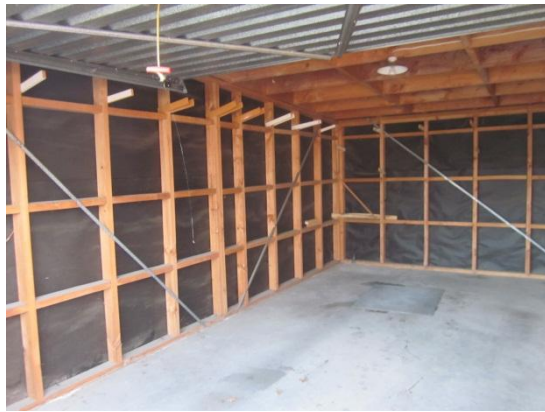
PHOTO 25: Garage 3 – Interior view
