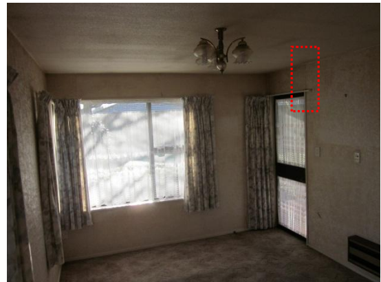
PHOTO 8: Maurice Carter Court Owner/Occupier Units – Interior view of the Unit 35. Hairline cracking in the gip lining above the rear entrance door.
