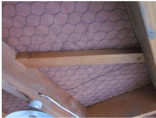
PHOTO 19: Garage 1 – Roof timber bracing
