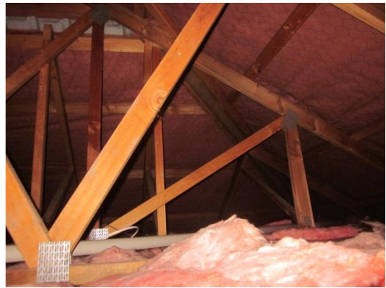
PHOTO 12: Maurice Carter Court Owner/Occupier Units – Interior view of roof space above Unit 30 towards east
