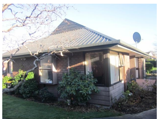
PHOTO 4: Maurice Carter Court Owner/Occupier Units – Exterior view of the Unit 30 from the East.
