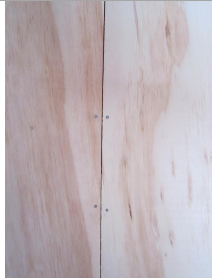
PHOTO 29: Close up view of the nail fasteners
