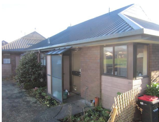
PHOTO 3: Maurice Carter Court Owner/Occupier Units – Exterior view of the Unit 30 from the South
