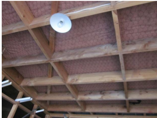
PHOTO 27: Garage 3 – Roof timber bracing
