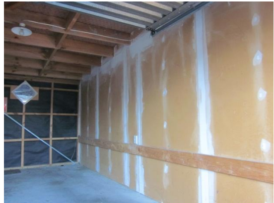
PHOTO 22: Garage 1 – Interior view (partition wall to the right)
