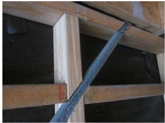
PHOTO 20: Garage 1 – Perimeter wall bracing
