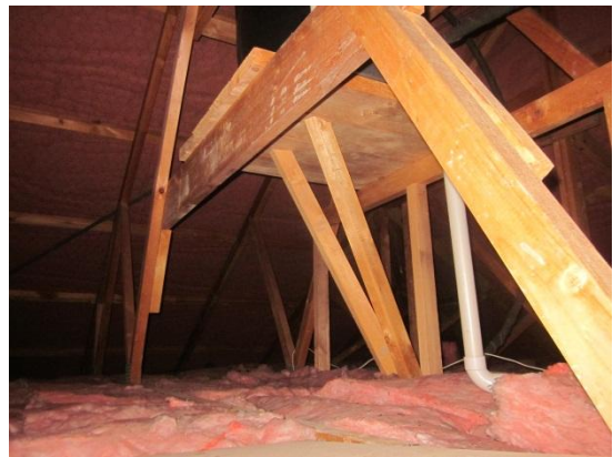
PHOTO 14: Maurice Carter Court Owner/Occupier Units – Interior view of roof space above Unit 30 towards north
