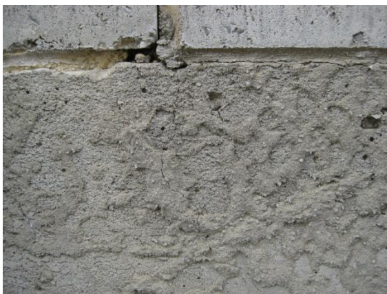
Photo 19: Typical vertical hairline cracking in the footing render
