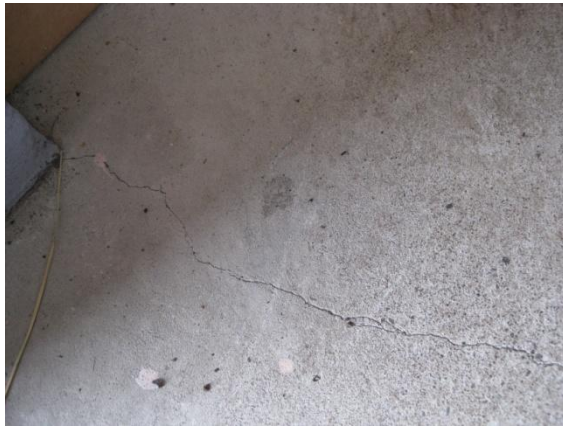
Photo 5: 0.5mm cracking in the internal slab in the women's toilet adjacent to an re-entrant corner
