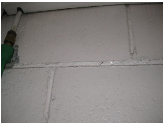
Photo 13: Hairline cracking below the top course of blocks in the north east corner of the men's toilet
