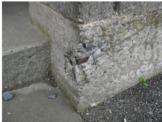
Photo 3: Typical spalled concrete and exposed reinforcement adjacent to door openings on the south side of the building
