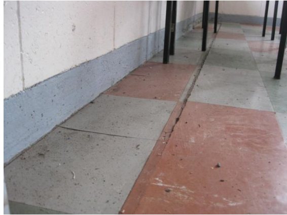
Photo 1: Differential settlement between the masonry wall footing and internal concrete slab in the lunchroom on the west side of the building
