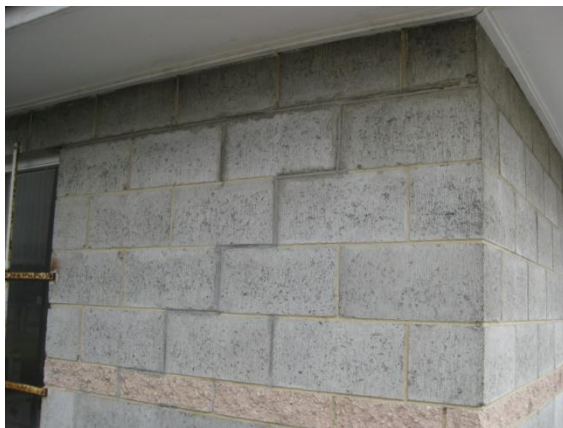
Photo 7: Repairs to the northern wall of the building completed prior to the earthquake. No damage to the repairs detected
