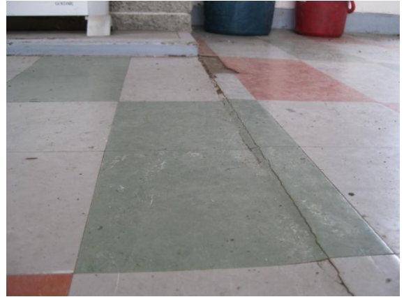
Photo 2: Differential settlement between sections of the internal floor slab in the lunchroom
