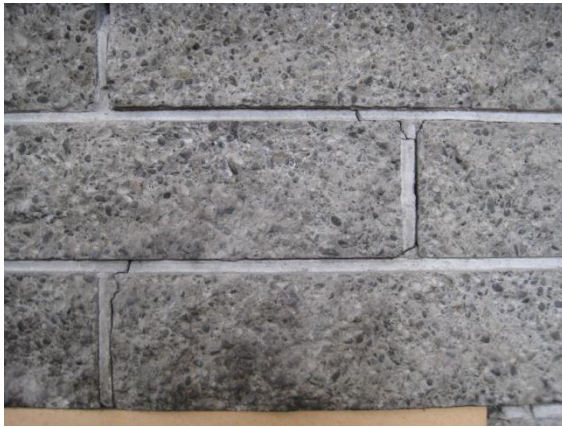
Photo 15: Cracking to the masonry render on the fireplace
