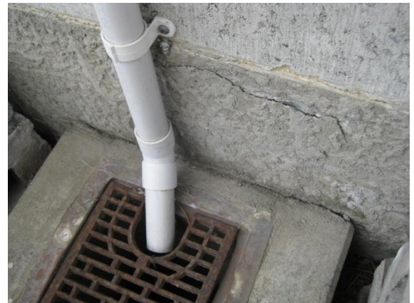
Photo 18: Render spalling off the northern masonry wall footing, adjacent to a drain
