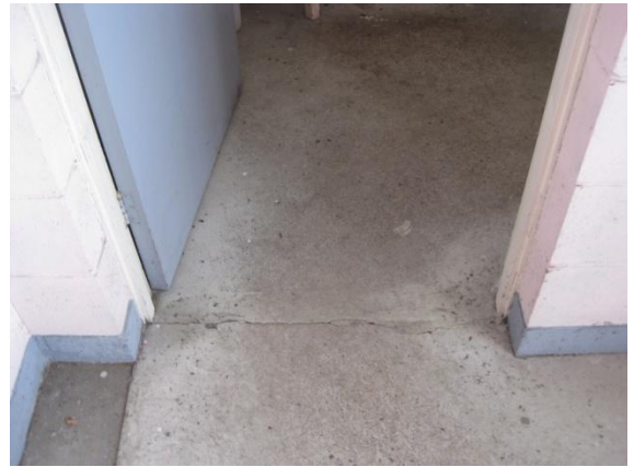
Photo 6: Cracking in the internal floor slab in the women's toilet at the doorway between the changing rooms and cubicles
