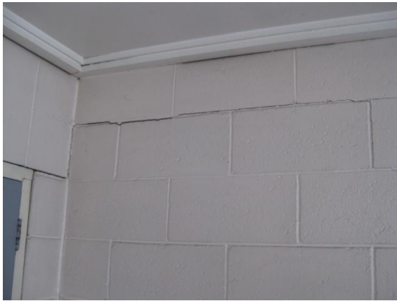
Photo 9: Cracking in the southern wall adjacent to the entrance to the lunchroom
