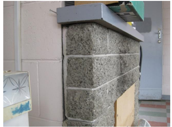
Photo 16: Separation between the masonry render and chimney in the lunchroom
