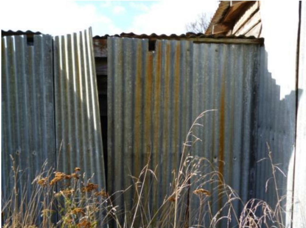
**Photograph 5 Loose Corrugated Iron cladding/sheeting.**
