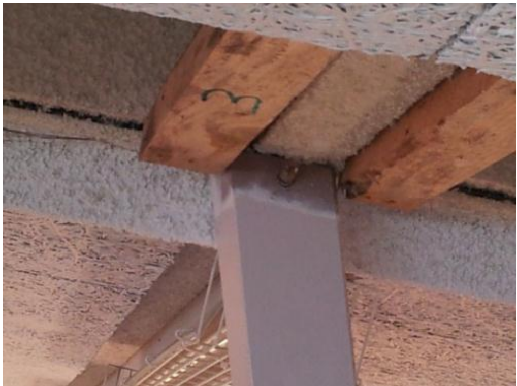
Photograph 25: Opening up works on roof showing the connection between the angle and box steel frame.
