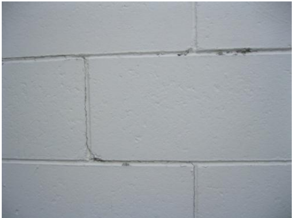
Photograph 9: Minor cracking along mortar lines to concrete blockwork
