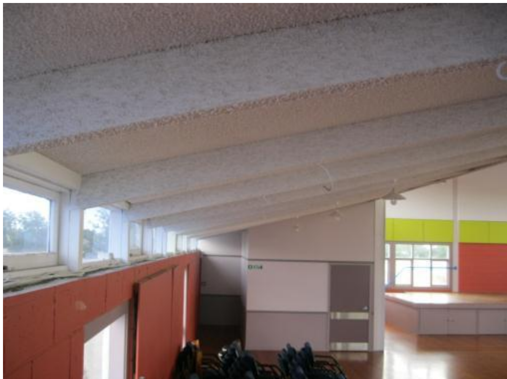
Photograph 8: Ancillary building blockwork not directly connected into roof
