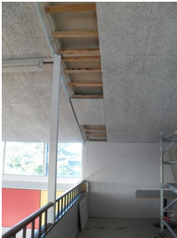
Photograph 20: Opening up works on roof within the mezzanine floor area
