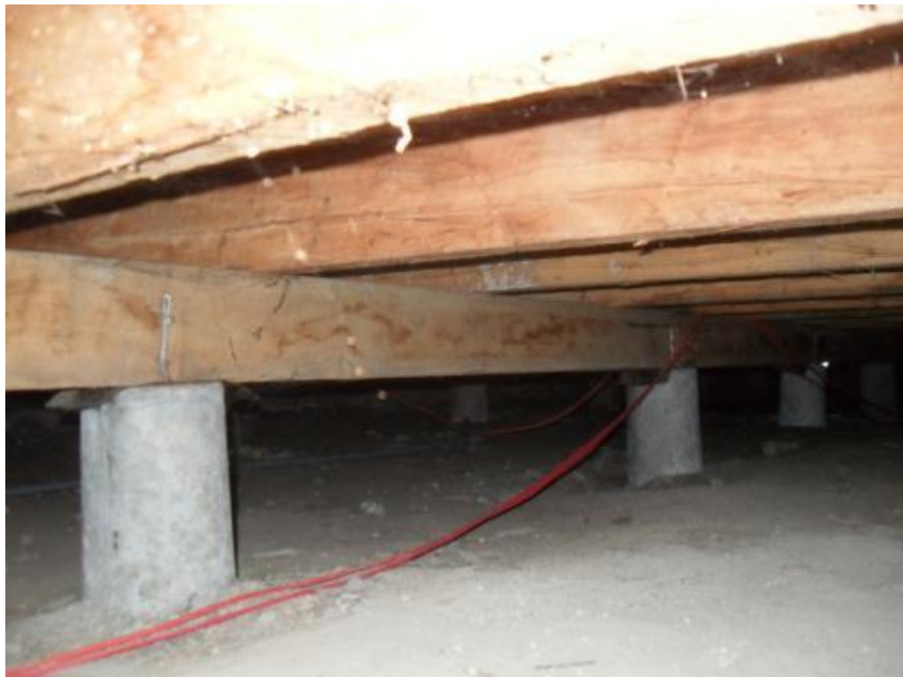
Photograph 19: Opening up works showing the timber floor system and foundation support
