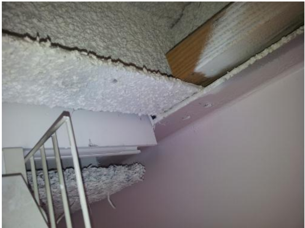
Photograph 27: Opening up works on roof showing the connection between steel portal frame and RSJ's
