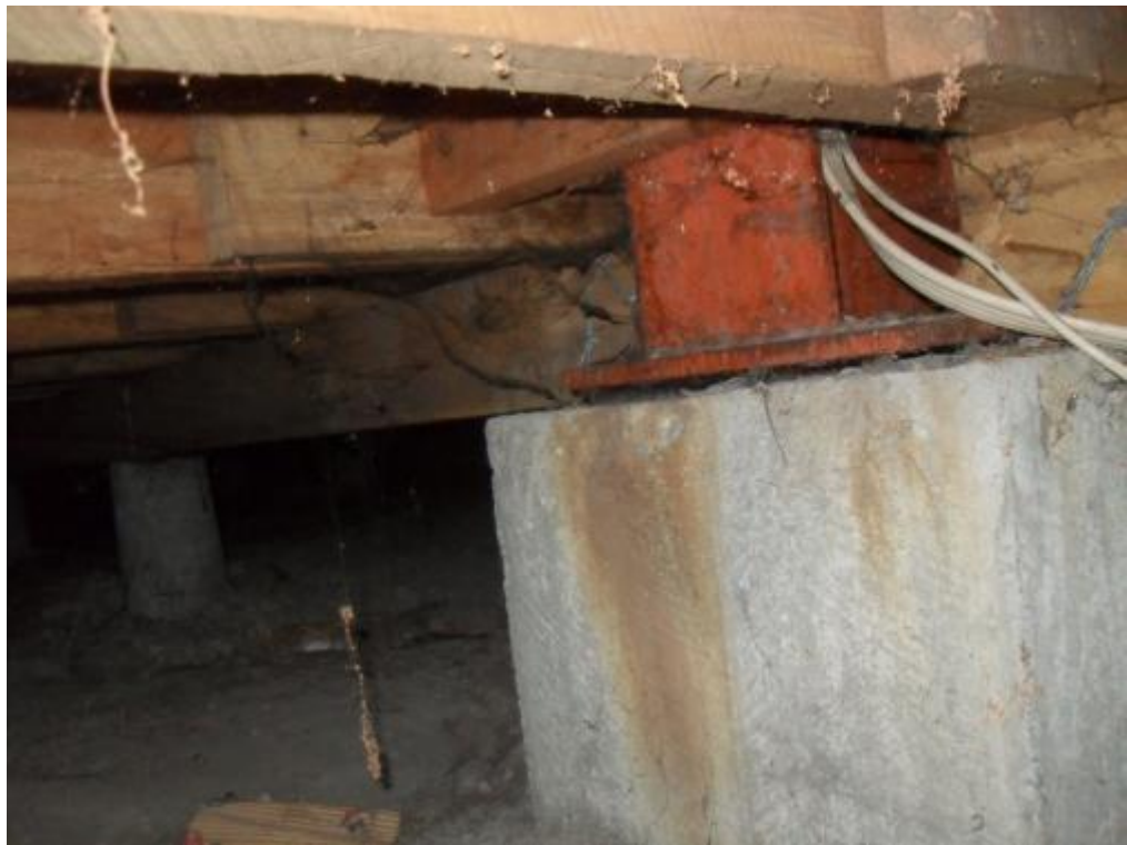
Photograph 17: Opening up work showing the foundation support under the steel portal frame
