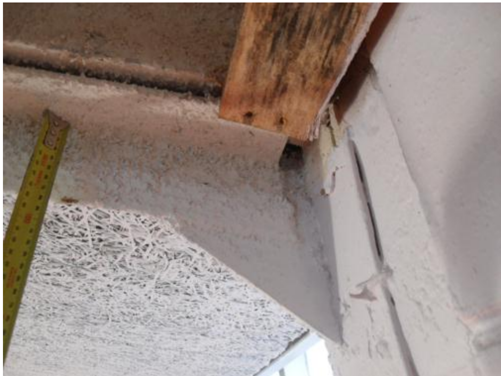
Photograph 21: Opening up works on roof showing connections between the steel frame and reinforced concrete column
