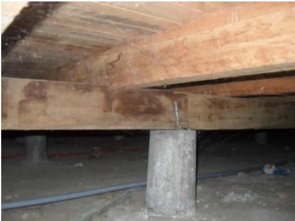
Photograph 15: Opening up works showing the timber floor system and foundation support
