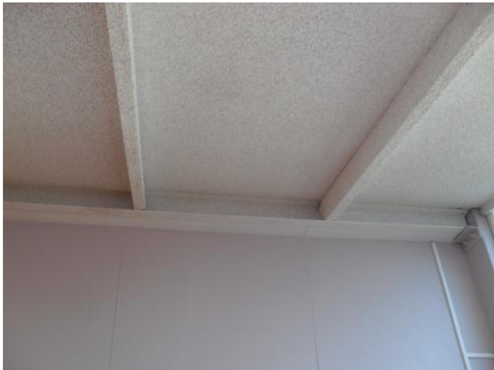
Photograph 31: Timber frame connections to PFC
