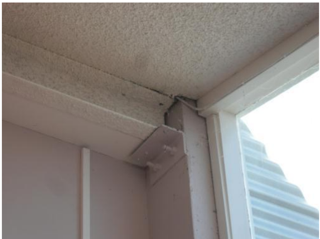
Photograph 30: Connection between the PFC and concrete frame
