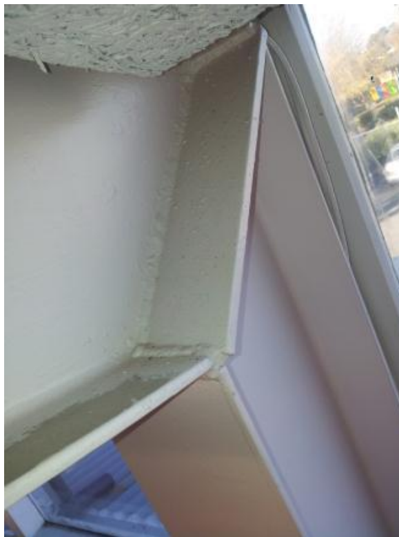
Photograph 28: Steel portal frame connections
