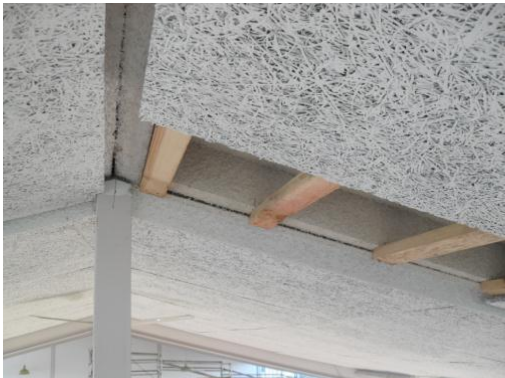
Photograph 22: Opening up works on roof within the mezzanine floor area. Shows the connection between the steel frame
