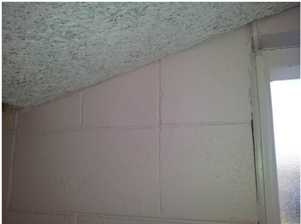
Photograph 26: Minor cracking along mortar lines to exterior blockwork walls located at mezzanine floor area
