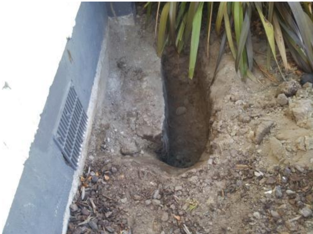
Photograph 13: Opening up works at exterior masonry wall showing the connection to foundation
