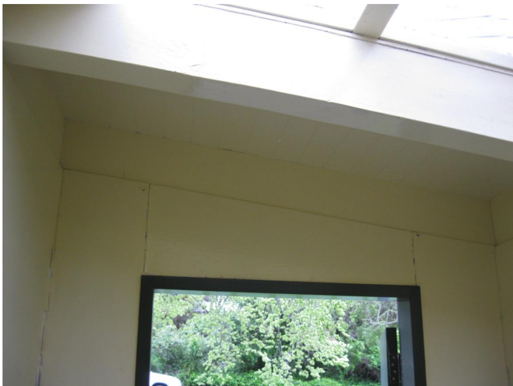
Photograph 6 Paint peeling at villa board lining joints.
