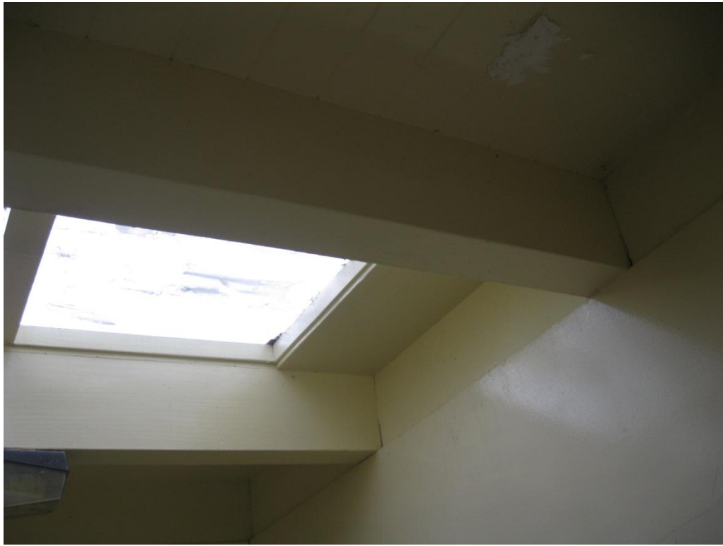
Photograph 5 Sun roof and timber beams.
