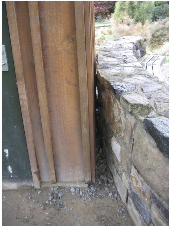
Photograph 7 Stonewall at southeast face of the building
