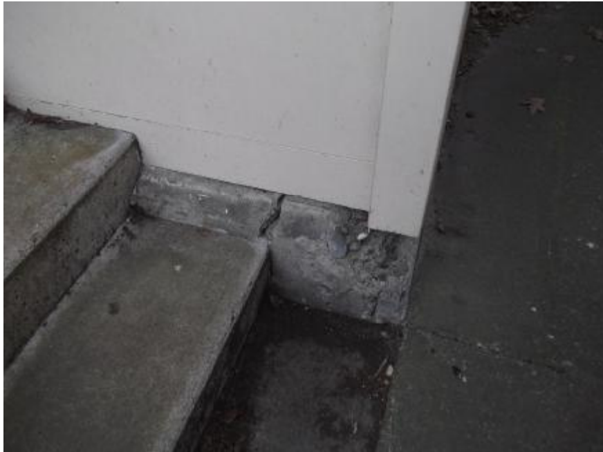
Photo 1: Cracking and spalling to foundation wall
