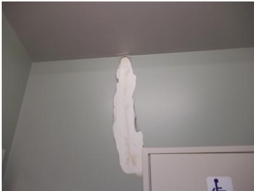
Photo 2: Cracking to wall lining with leaking stain
