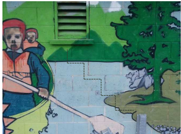
Cracking along the mortar on the eastern side of the building.
