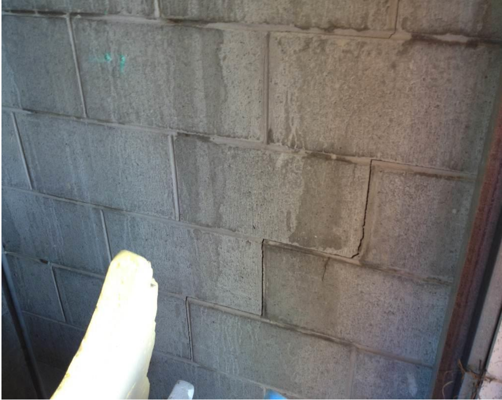
Photo 3: Blockwall at ground level.
