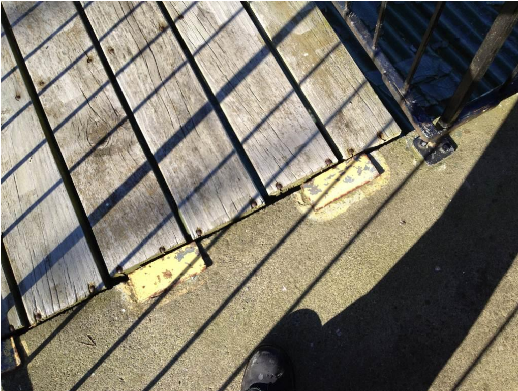
Photo 9: South staircase upper deck
