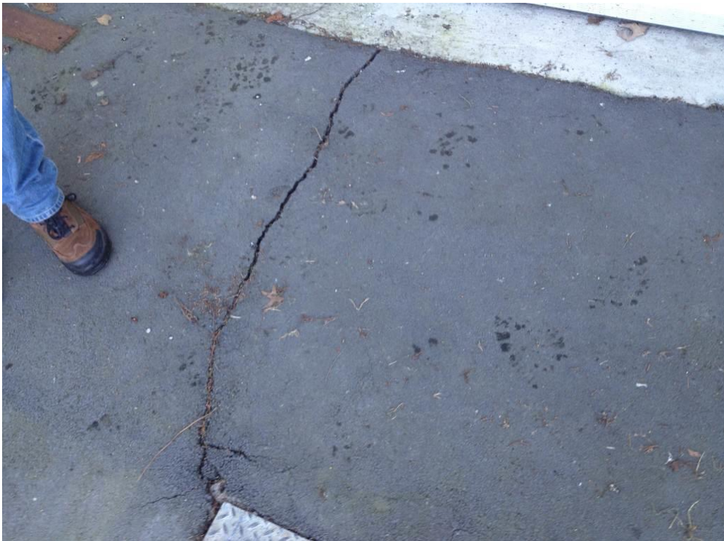
Photo 4: External asphalt pavement.
