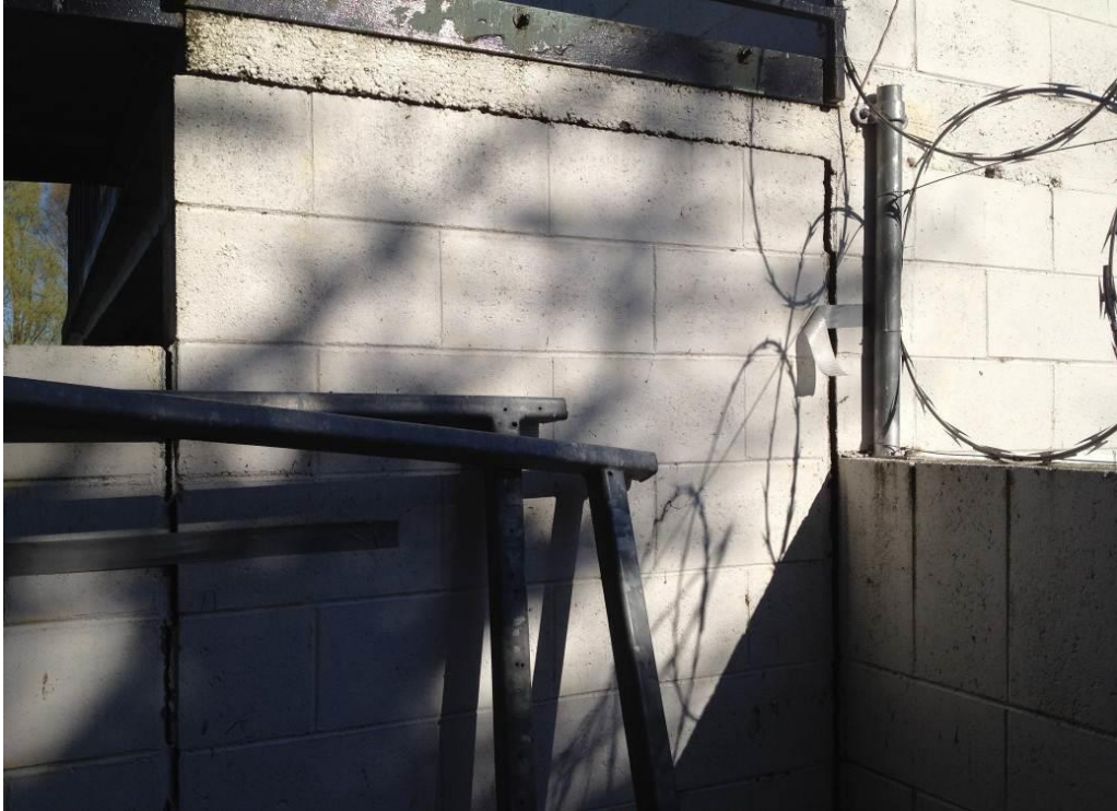
Photo 5: East blockwall supporting the exterior precast floor units
