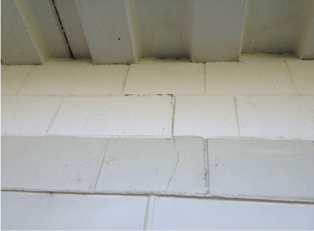
Photo 8: West blockwall underneath the precast floor units.
