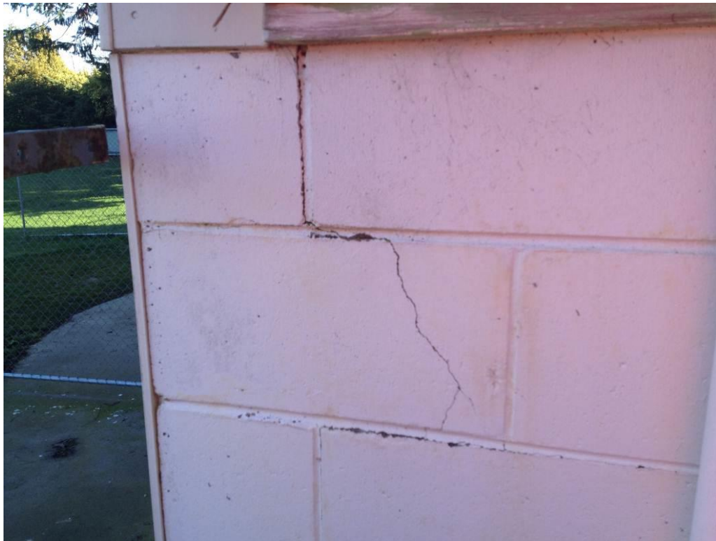
Photo 8: Ground level blockwall damage.
