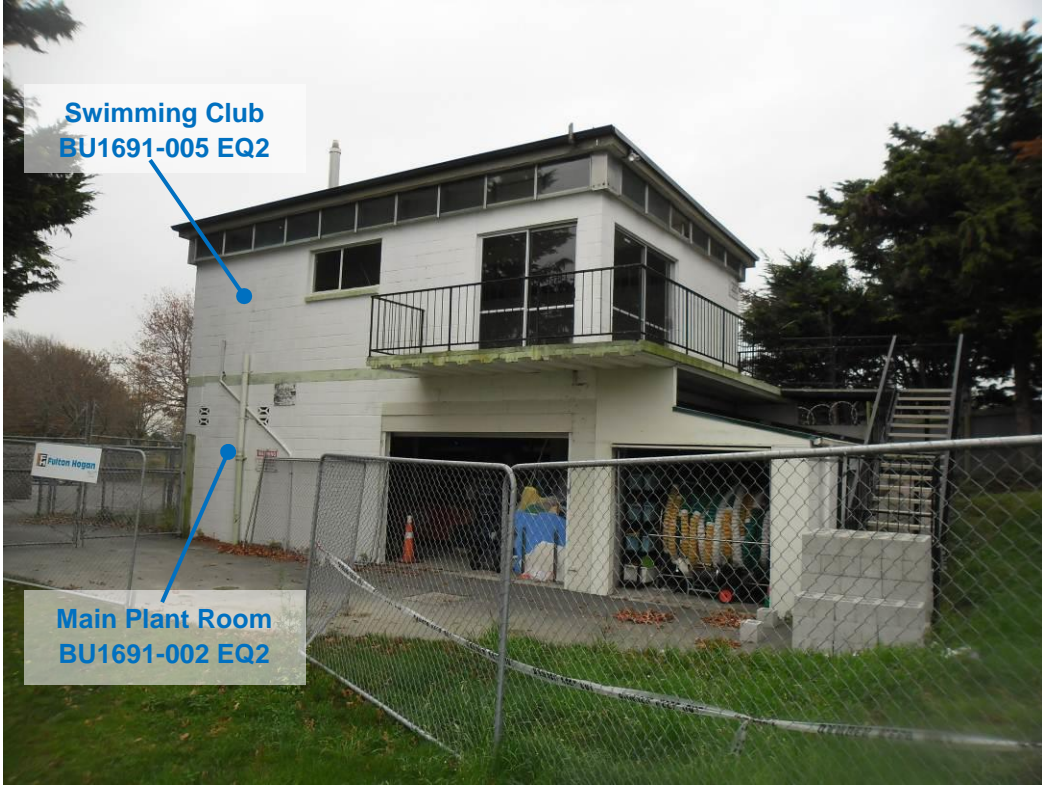
Photo 1: External view of North East elevation
