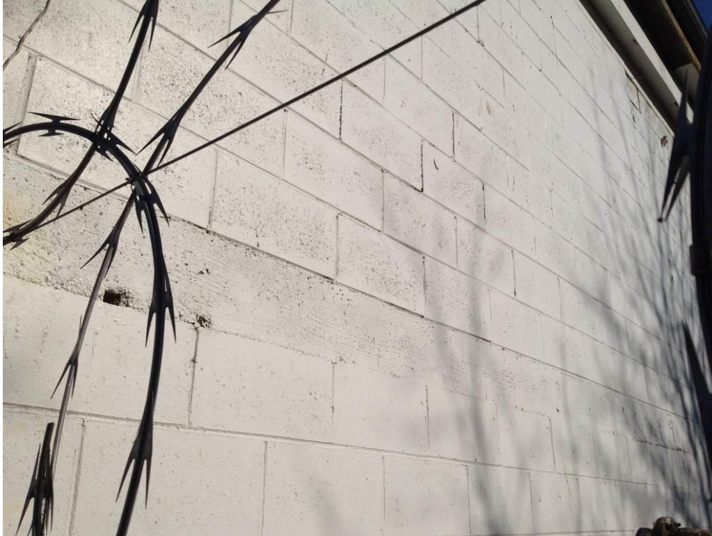
Photo 7: East blockwall elevation
