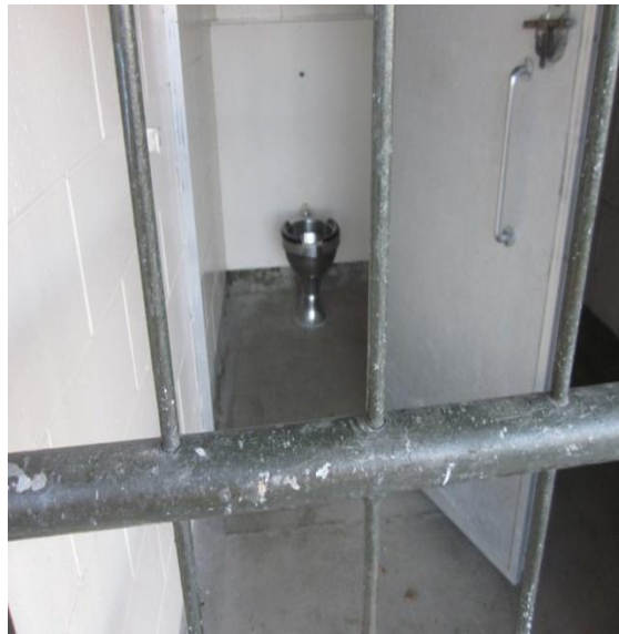
Photo 9: Interior of one of the toilets on the south side showing the concrete floor slab.
