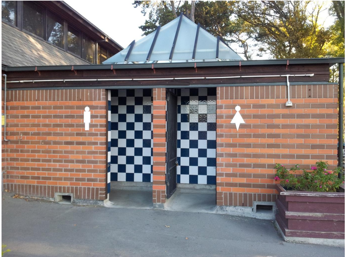
■ Figure 9 Overview of structures – Netball toilets
