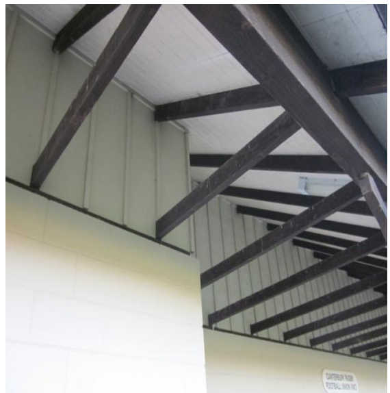
Photo 12: Soffit on east side.
