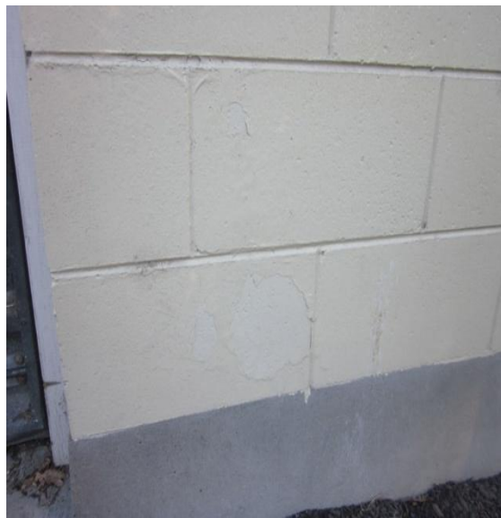
Photo 19: Existing paint damage to north masonry wall.
