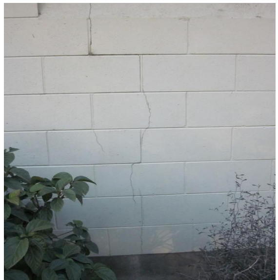
Photo 24: Vertical crack through masonry blocks on west wall.
