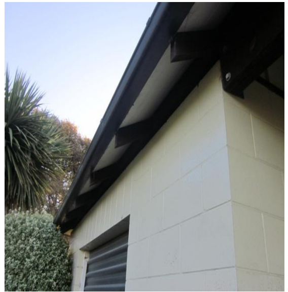
Photo 6: Soffit of south side of building
