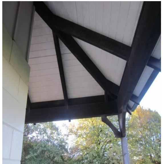
Photo 16: Soffit and support on northeast corner.
