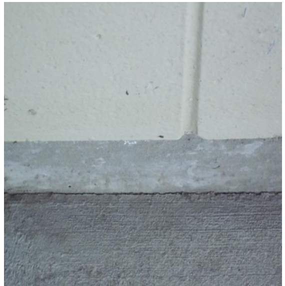
Photo 10: Gap opening up between the concrete strip under the masonry wall and the external concrete ground slab on the east side.
