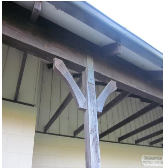
Photo 13: Soffit and support on east side.
