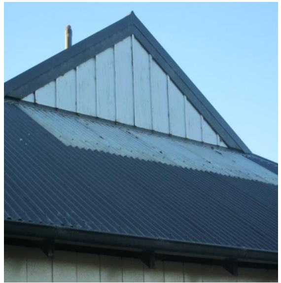
Photo 26: External roof cladding on south side.
