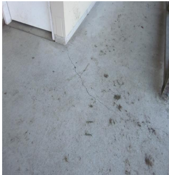
Photo 15: Crack in external concrete ground slab on east side.
