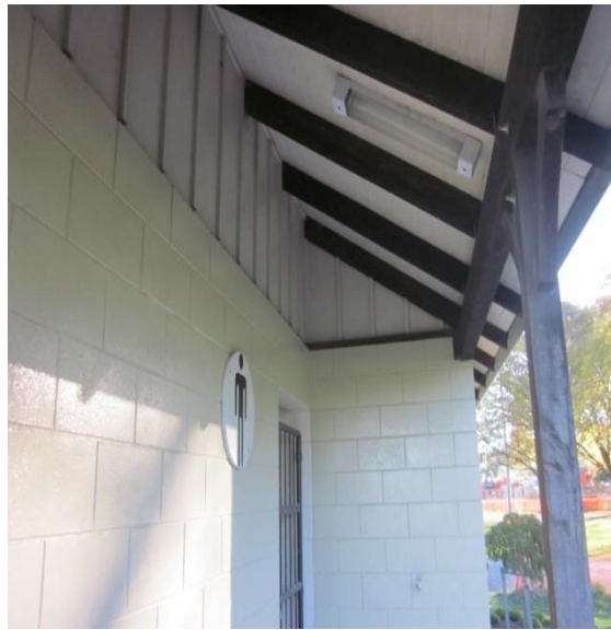
Photo 17: Soffit and support on north side.
