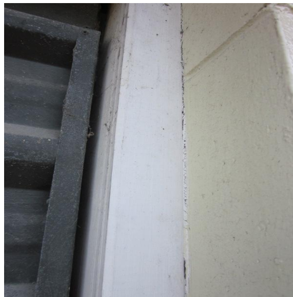
Photo 20: Gap opening up between timber doorframe and masonry wall on north side.
