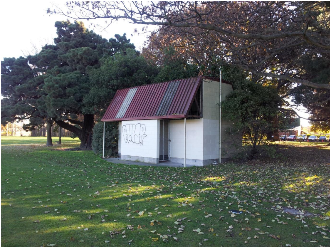
■ Figure 8 Overview of structures – Hospital toilet
