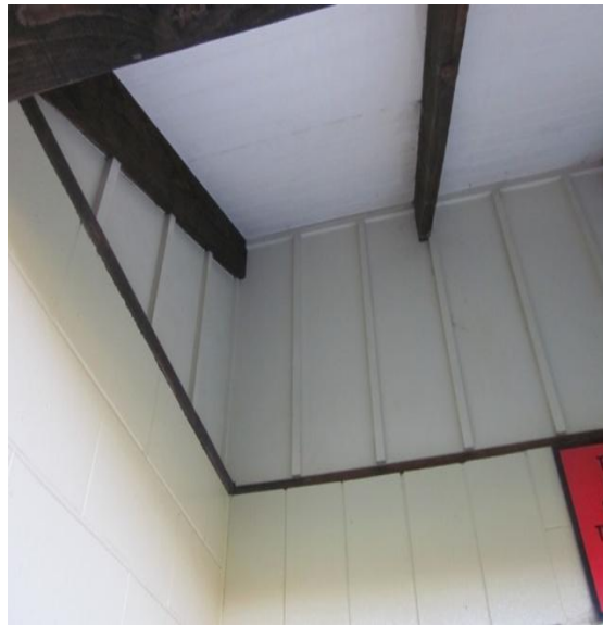
Photo 5: Soffit of south side of building.
