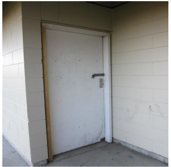
Photo 14: One of two doors on east wall.
