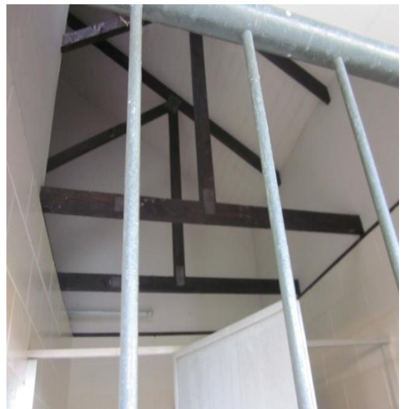
Photo 8: Interior of one of the toilets on the south side showing timber roof framing.
