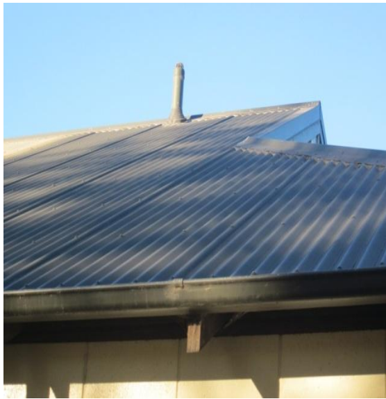
Photo 25: External roof cladding on west side.
