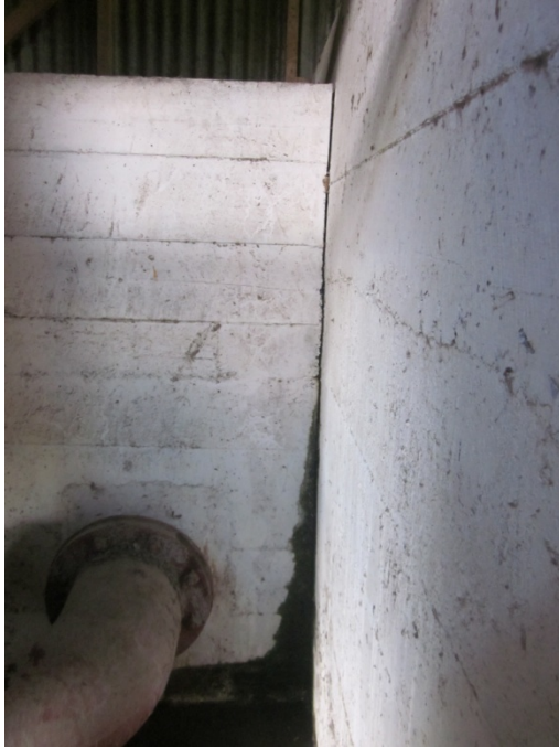
Photo 13: Walls separated at junction.
