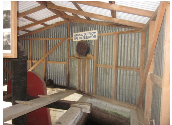
Photo 4: Interior view of pumphouse-South east elevation
