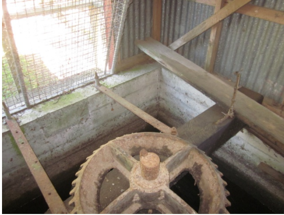
Photo 9: Tank above the creek. Southern view
