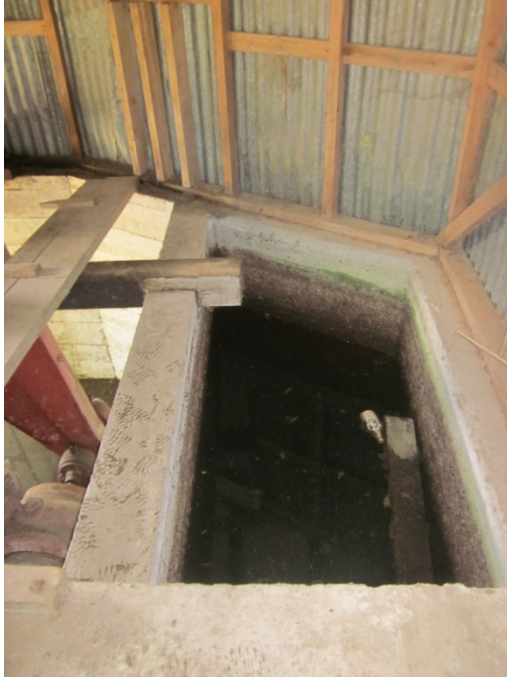
Photo 5: Interior view of water tank at south east.
