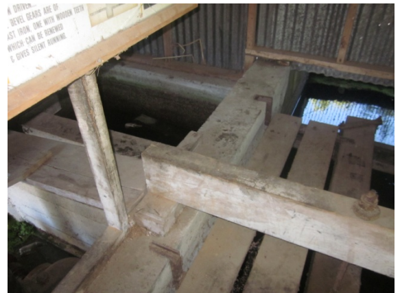
Photo 12: Interior wall dividing the rooms of the pumphouse
