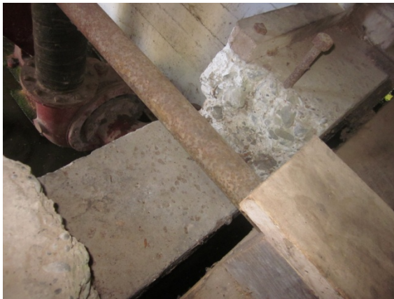
Photo 15: Cut out in interior wall exposes the quality of concrete.
