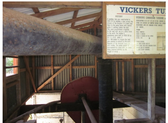
Photo 8: West view of pumphouse.
