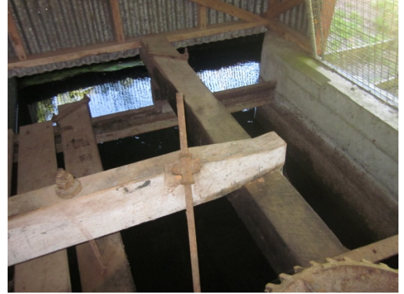
Photo 10: Tank above the creek. Northern view
