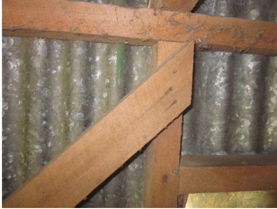
Photo 17: Connection of bracing elements in timber structure. Note that connection is made just with three nails.
