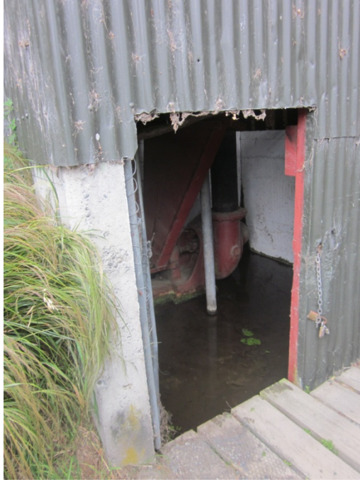
Photo 1: Entrance to the pumphouse at north east
