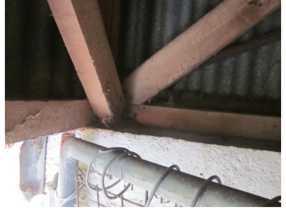
Photo 18: Connection of elements in timber structure.
