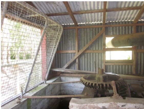
Photo 7: Interior view of pumphouse. South west elevation
