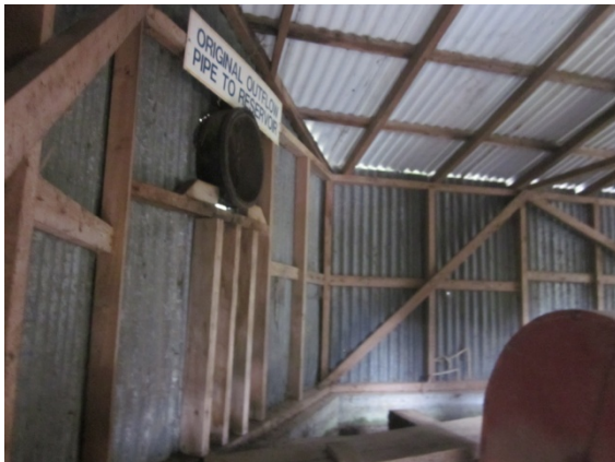
Photo 3: Interior view of timber structure-North elevation
