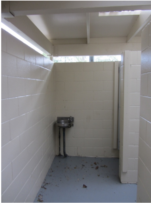
Photo 5: Interior of womens toilet
