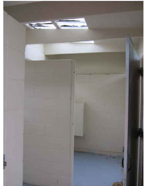
Photo 4: Interior of womens toilet
