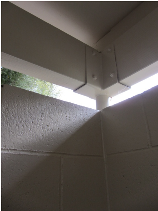
Photo 7: Steel tube connection
