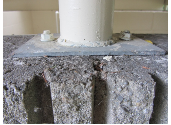
Photo 10: Roof connection
