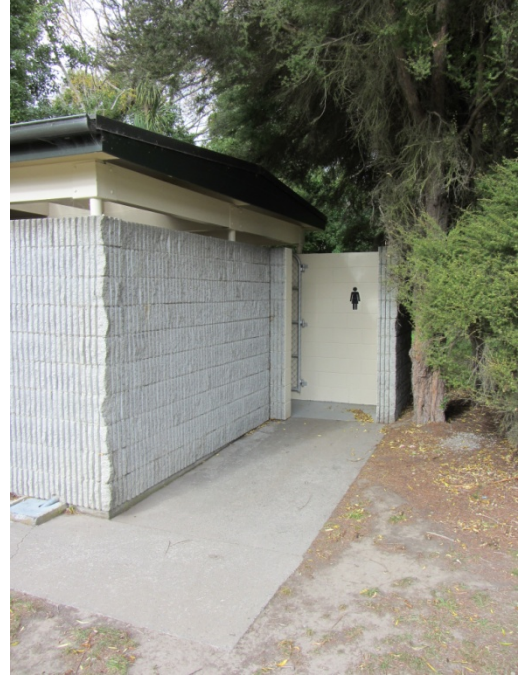
Photo 2: West Elevation. Womens toilet
