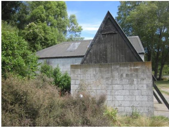
Photo 23: East of the building showing timber cladding to toilet A frame structures
