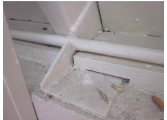
Photo 8: Top of 1.4m tall concrete masonry walls connected to RHS by bolted and welded cleat. M8 bolt
