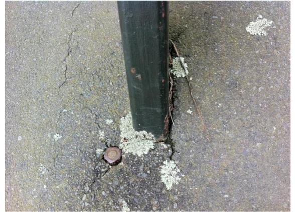
Photo 6: Base of the rectangular hollow sections (RHS) passing through asphalt into foundations
