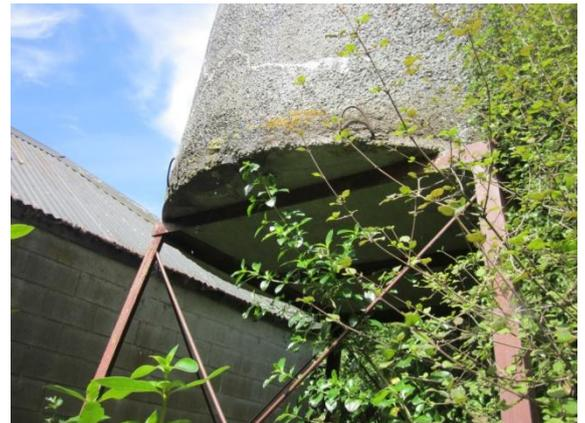
Photo 26: Supports constructed of a braced steel frame with equal angle legs and beams
