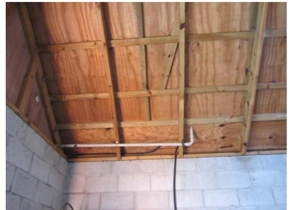
Photo 22: Light timber battens on timber rafters with a plywood lining beneath the profiled metal cladding
