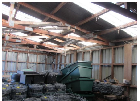
Photo 6: Interior view looking along west wall
