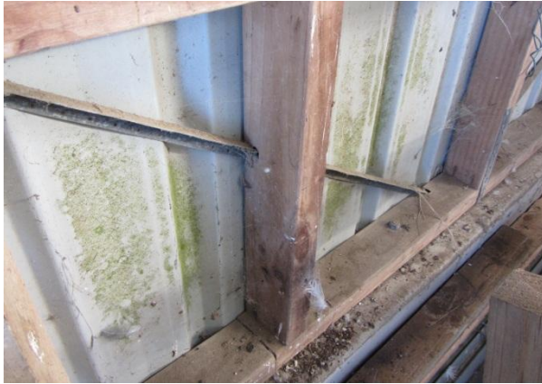
Photo 9: Close up view of the angle brace on south wall.
