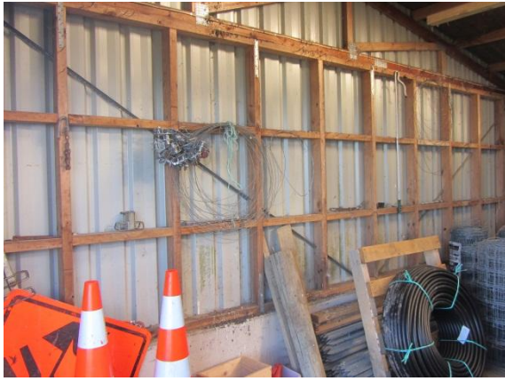
Photo 7: Interior view of south wall
