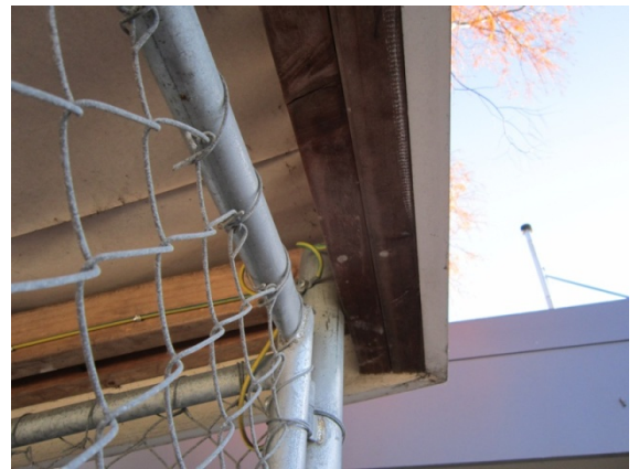
Photo 12: Connection between steel hollow section column and timber roof edge beam on north east corner.
