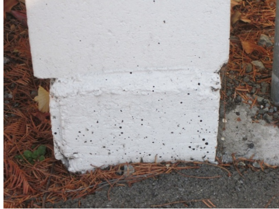
Photo 5: Concrete strip footing directly under masonry walls.
