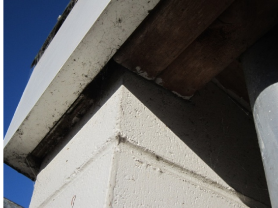
Photo 9: Timber edge beam on east side.
