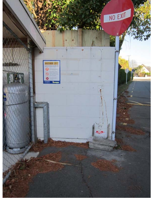
Photo 14: Masonry wall extension past roof on west side.
