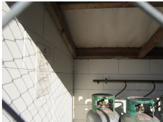
Photo 7: Timber-framed roof and masonry walls.
