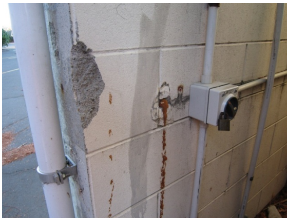
Photo 15: Existing impact damage to west wall extension and traces of ceiling foam in an existing cavity.
