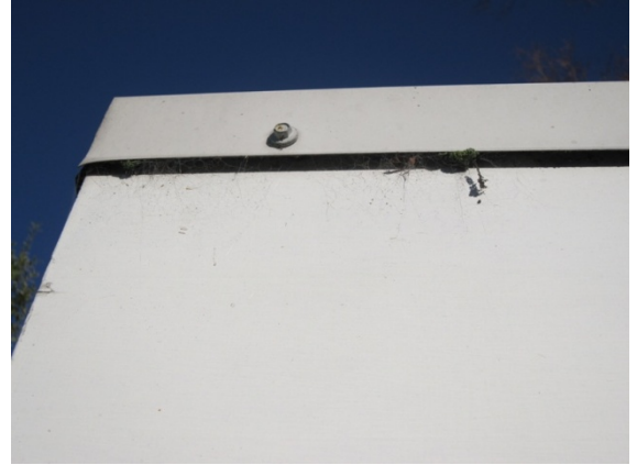
Photo 10: Steel cap plate above east wall.
