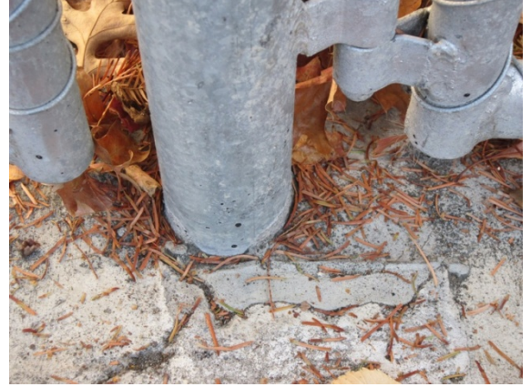
Photo 18: Ground connection of steel hollow section columns (typical).
