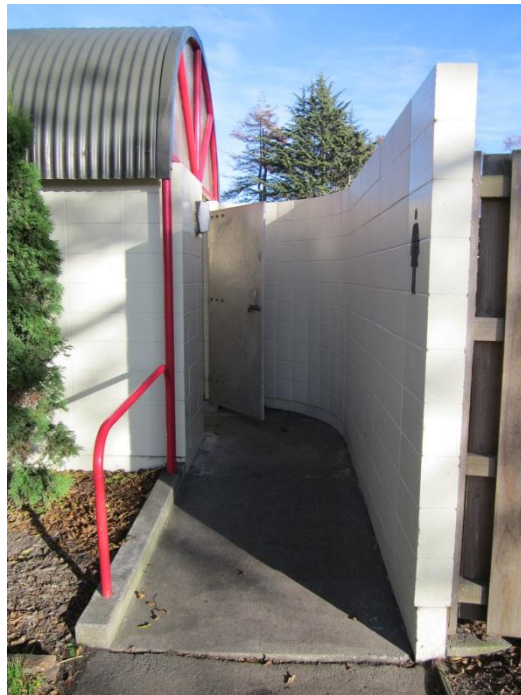
View of external reinforced concrete block-walls (North end).
