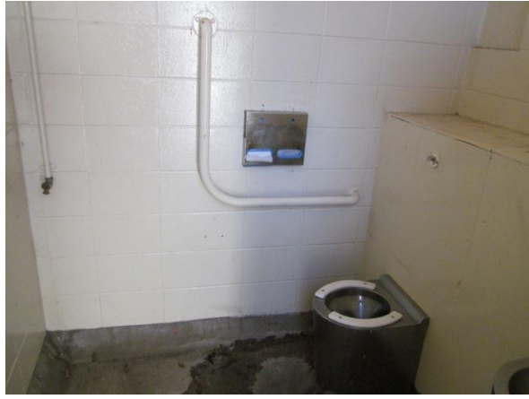
Interior view of reinforced concrete block-walls.
