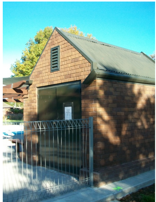
Photo 4: Plant Room – South Elevation
