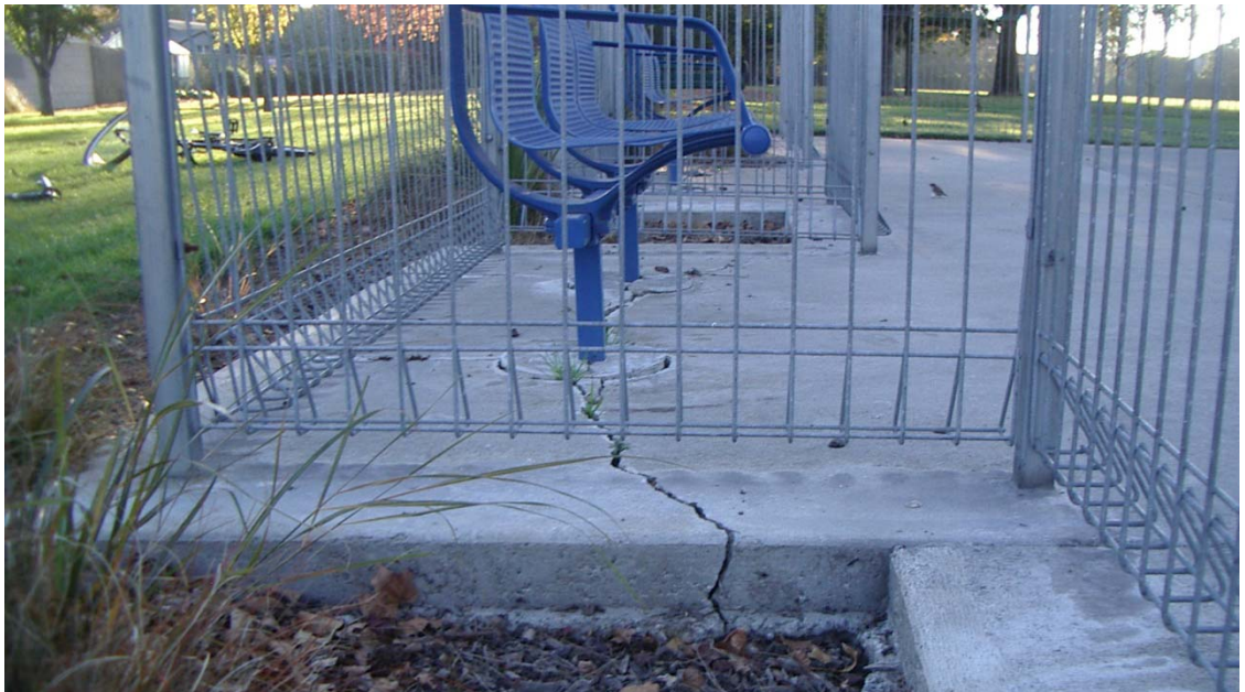
■ Figure 7 Observed cracking around the seating area
