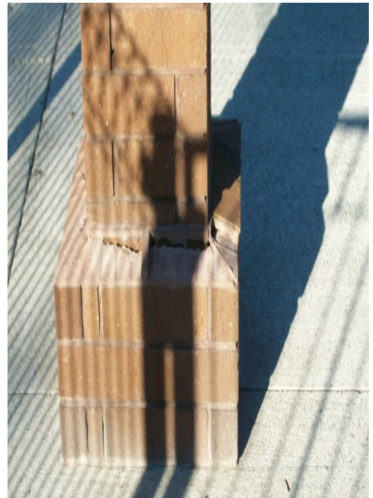
Photo 8: Missing Capping Bricks
