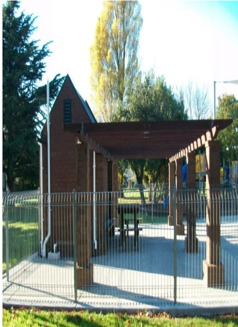
Photo 1: Plant Room – West elevation
