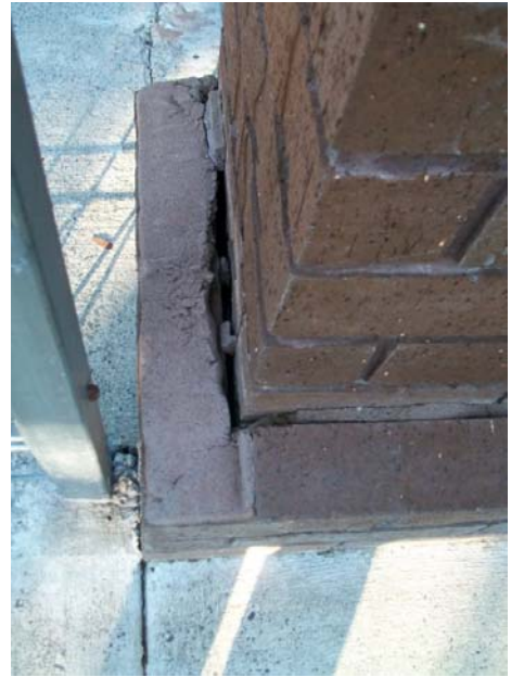
Photo 6: Missing Capping Bricks at the Top of The Foundation
