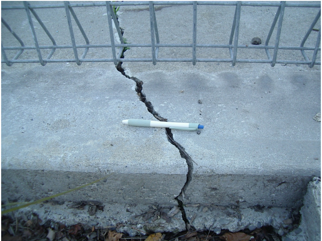
■ Figure 6 Observed cracking around the seating area near the paddling pool
