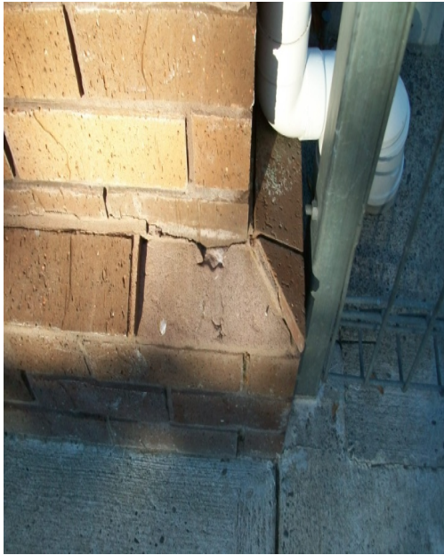
Photo 5: Missing Capping Brick at the Top of The Foundation
