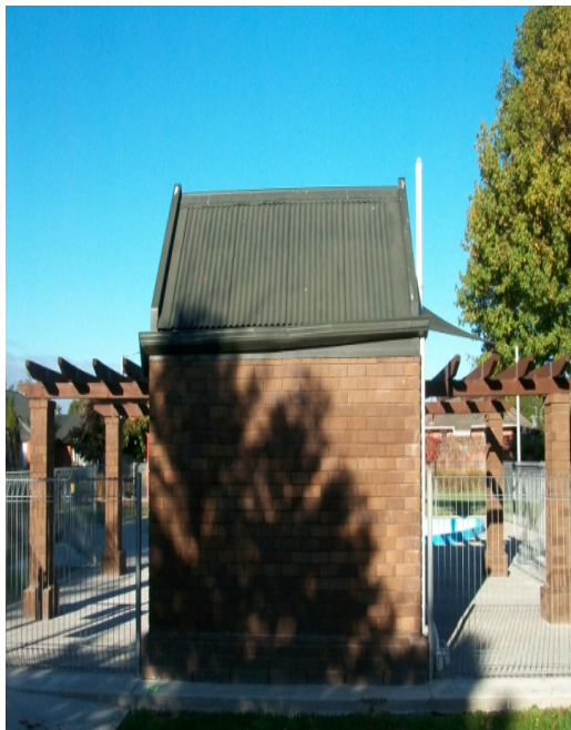
Photo 3: Plant Room – North Elevation
