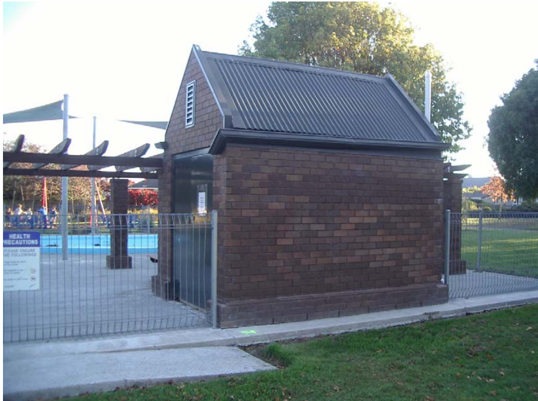
■ Figure 5 Overview of shed with the paddling pool visible in the background
