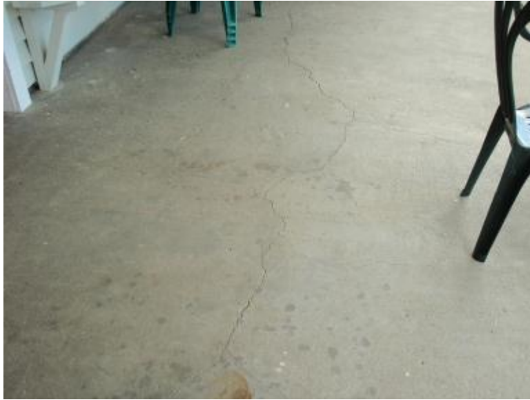
Photo 11 Cracking on Veranda Concrete Slab On-Grade
