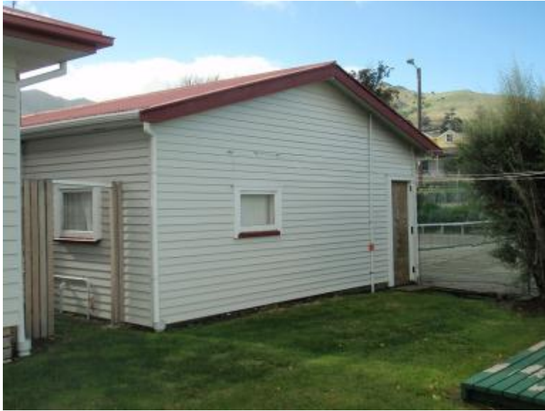
Photo 3 South Elevation of the Building
