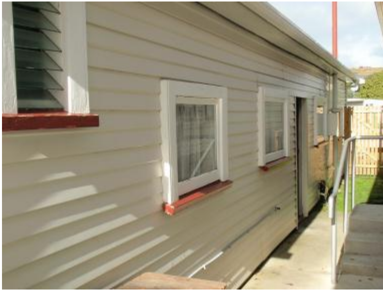
Photo 1 West Elevation of the Building
