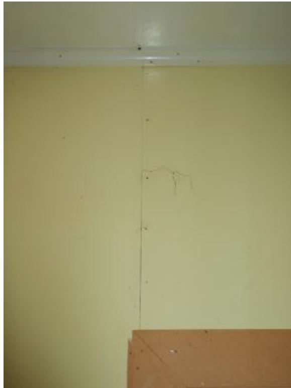
Photo 9 Cracking to Interior Linings
