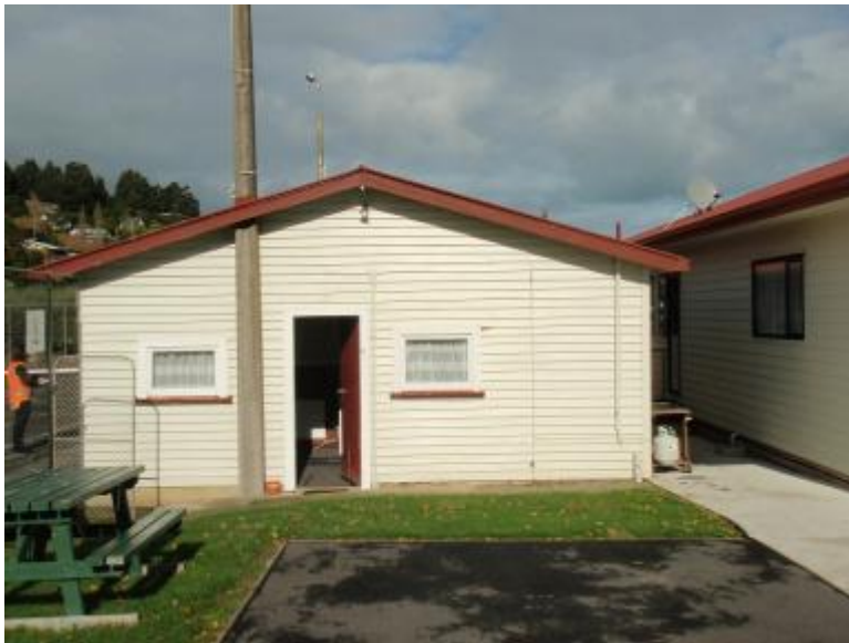
Photo 2 North Elevation of the Building
