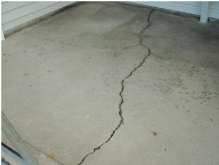
Photo 10 Cracking on Veranda Concrete Slab On-Grade
