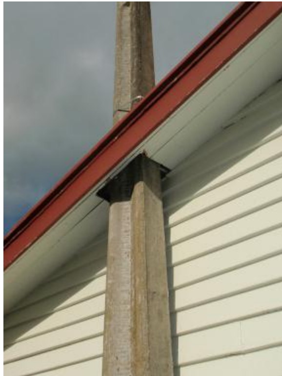
Photo 5 Light Pole Adjacent to North Elevation of the Building
