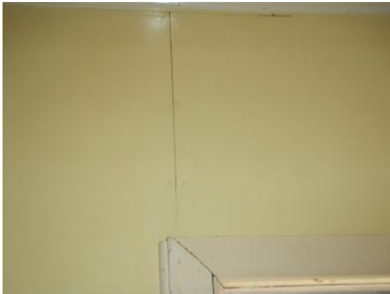
Photo 8 Opening to Joint of Interior Linings
