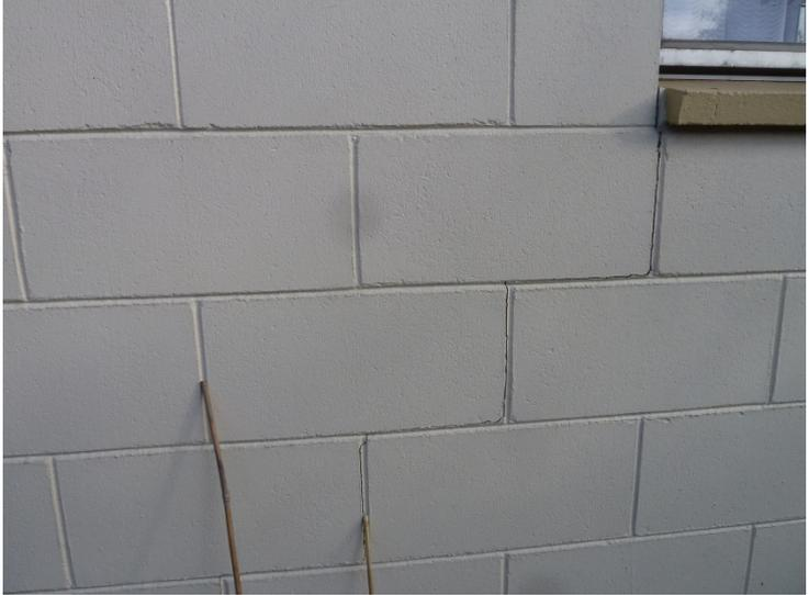
A close-up photograph of a wall made of grey concrete blocks. The mortar joints between the blocks show significant stepped cracking, where the mortar has crumbled away, creating a jagged, uneven surface.                                                                                                |
