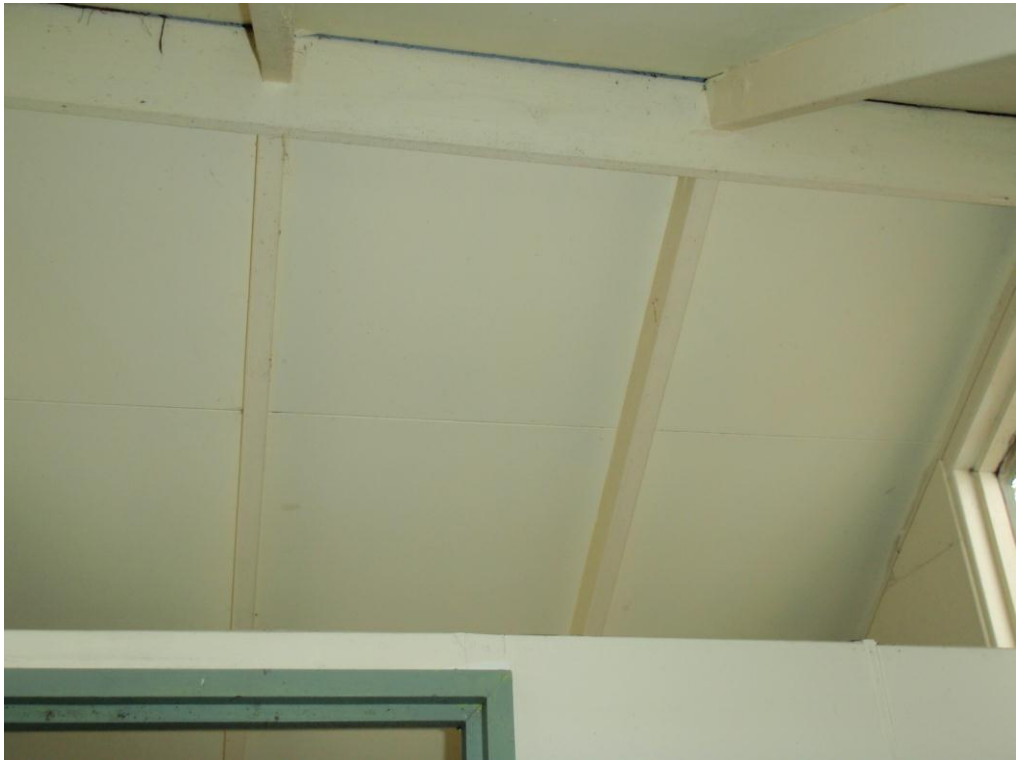
Photograph 10: View of roof rafters and plywood lined ceiling
