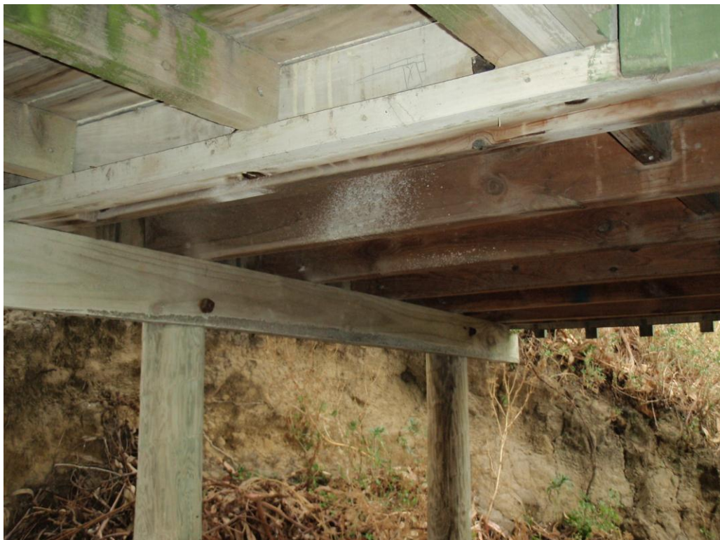
Photograph 6: View of timber bearer and timber piles forming the subfloor structure
