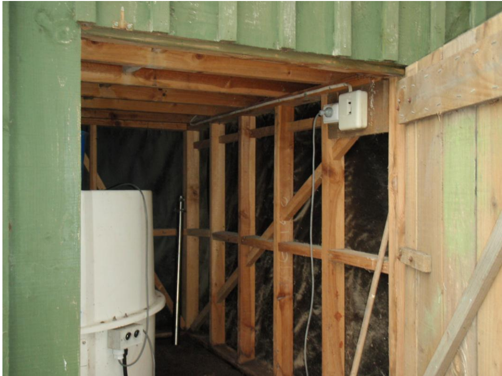
Photograph 5: View of timber framed subfloor walls
