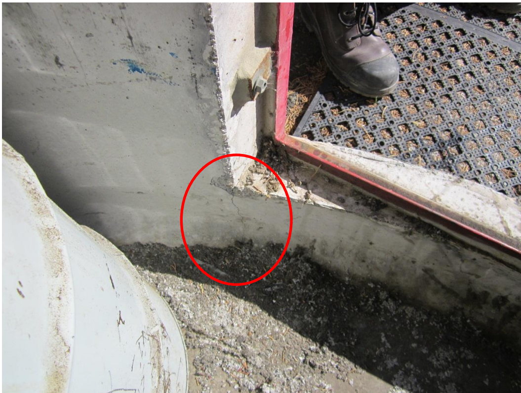
Fresh crack around the door opening
