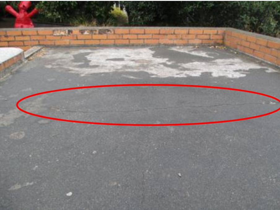
A photograph showing the exterior of a roof. The roof surface is dark asphalt, showing signs of weathering and discoloration. A prominent crack runs across the middle of the frame. A red circle is drawn around this crack to highlight it. In the background, there is a brick wall and some greenery, including a red sculpture or structure. |
