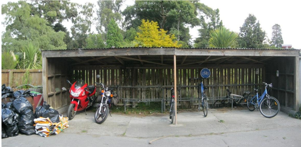
Photograph 5 Eastern view of the cycle shelter.
