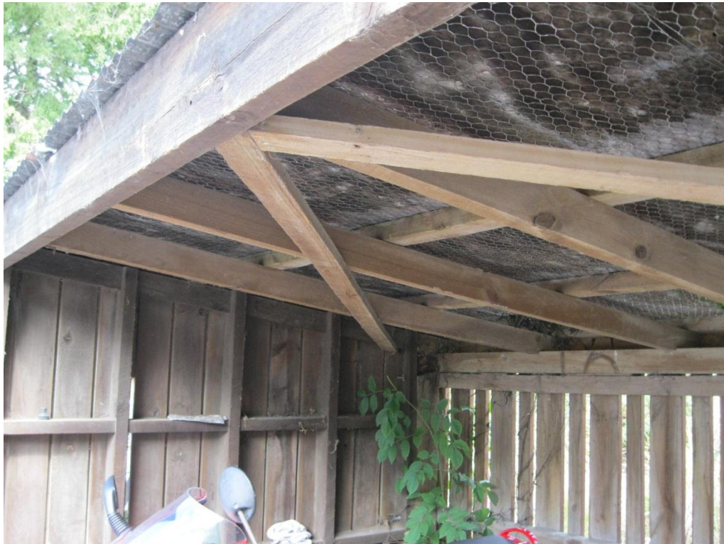
Photograph 3 Underside of the roof of the building showing cross bracing, rafters, purlins and metal cladding.
