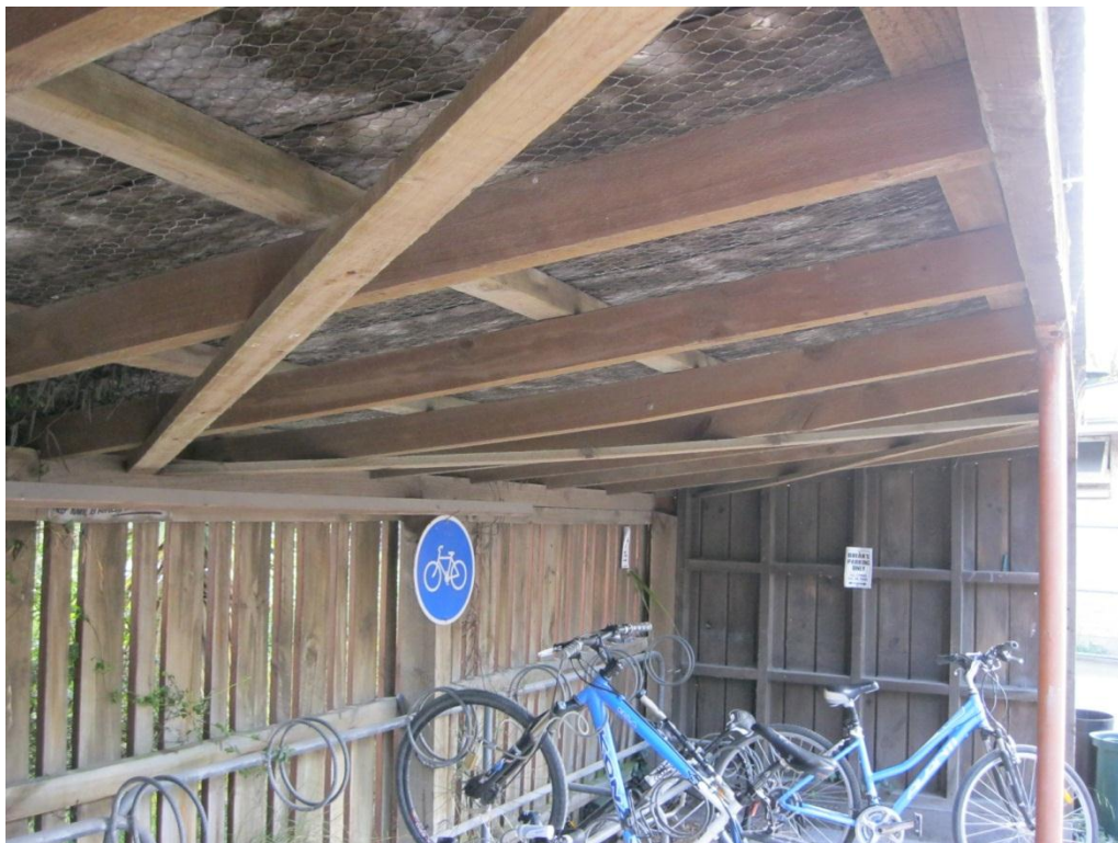
Photograph 4 Internal view showing steel CHS post at front and timber post system at the rear. Timber framed end walls are clearly visible.
