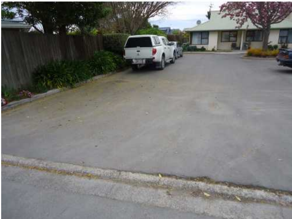
Figure 2: An area of the south car park (approximately 6.5 m X 7.0 m) has undergone heaving and settlement.
