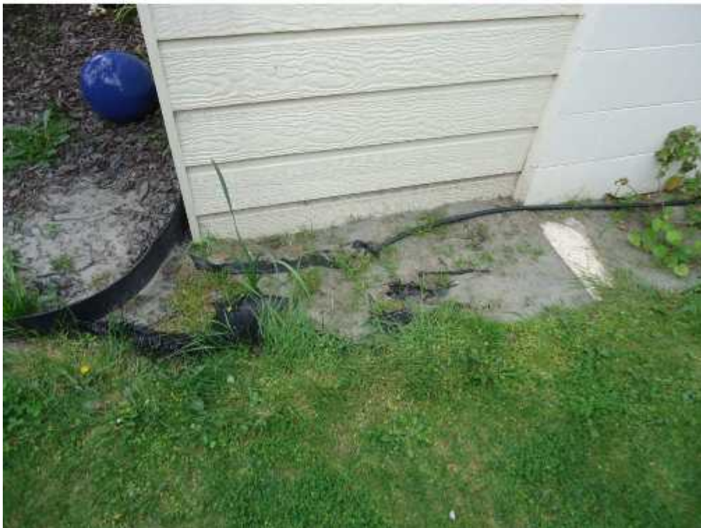
Figure 8: Liquefied material ejected (grey silt with some fine sand) from sand boils that surrounded the Middle building.
