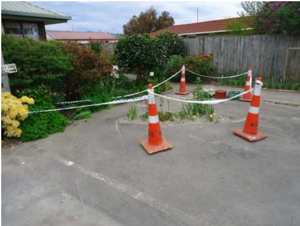
Figure 17: South side of the North building, as a result of liquefaction during 13 th June 2011 earthquake. The dimensions of the bulge are 4.50 m X 3 m and the ground heave is 100 mm. Ejected Silty material (grey, non-plastic) is deposited.
