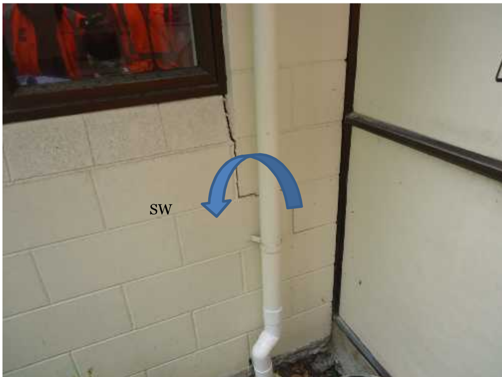
Figure 16: Settlement crack below the corner of the window, South building. The crack has width <5\text{mm} and possibly penetrates through the wall. Movement may have taken place towards the South west.
