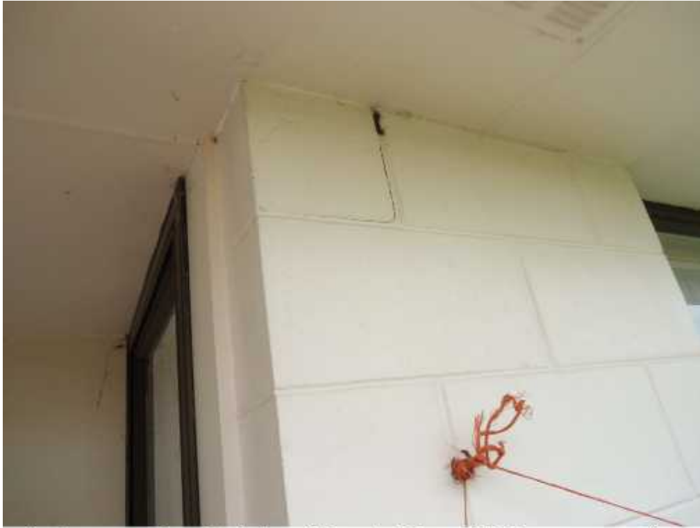
Figure 13: A minor crack at the joint of the cladding. Width: 5-10mm. The crack does not appear to penetrate through the cladding in the North side of the North building.
