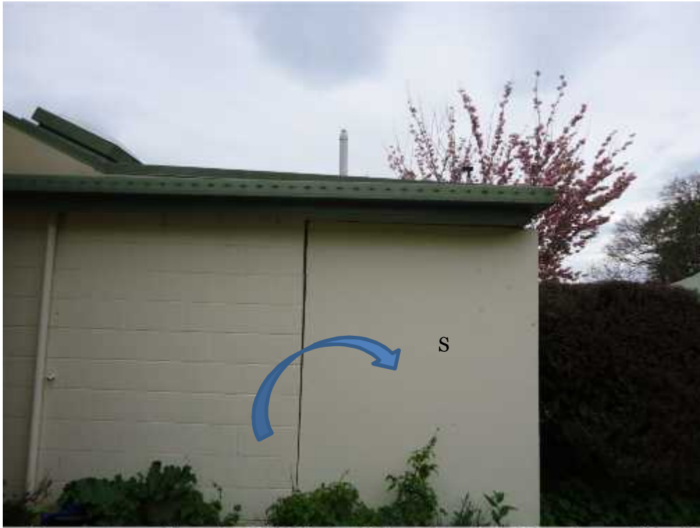
Figure 3: A 20mm crack at the Middle building that detaches the walling from the cladding.
