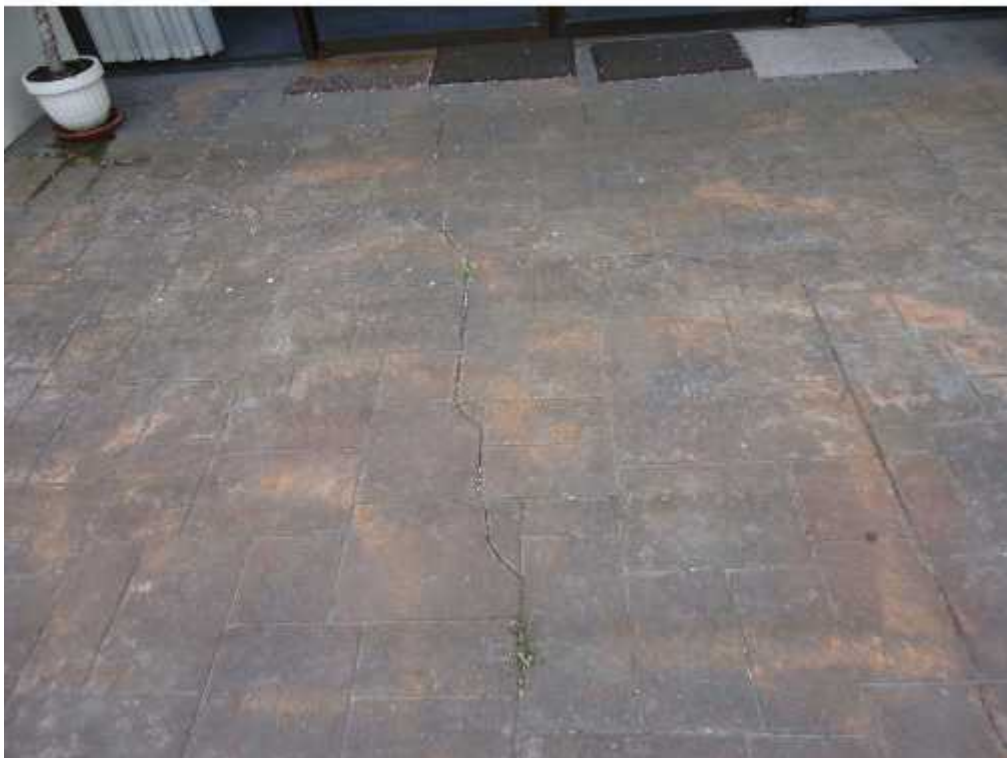
Figure 6: Longitudinal 5 mm wide cracks outside the residents' lounge, Middle building on stone paved entrance.
