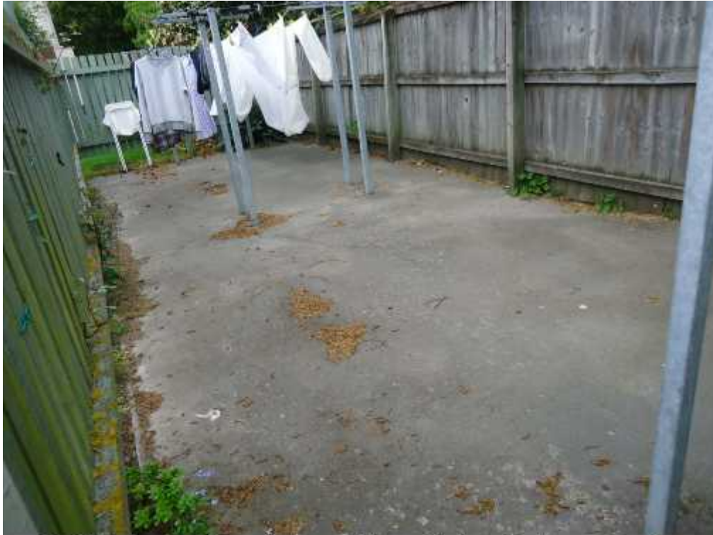
Figure 9: Undulating surface of the residents clothes drying areas. Some minor cracking up to 5 mm wide.
