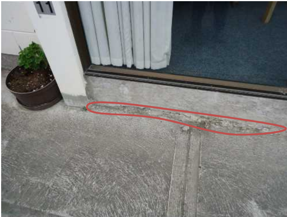
Figure 5: The foundation of the middle building is exposed by 70 mm from its initial position due to possible settlement of the surrounding ground. (Middle building, east side).
