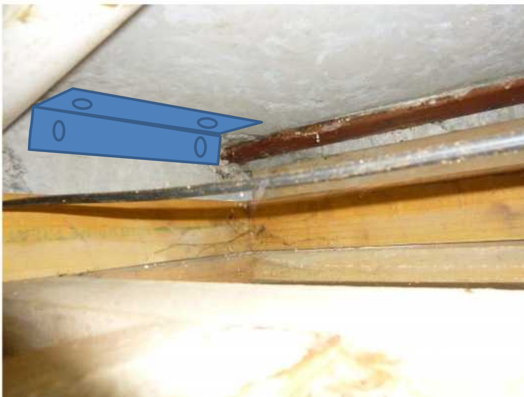
Indicative location of angles above bathroom ceiling.
