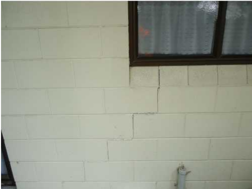
Figure 14: Stepped pattern of crack <5mm just below the window of flat 3, South building.
