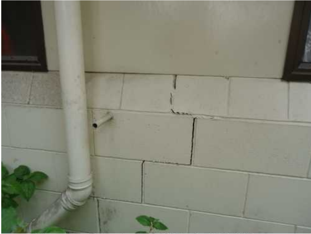
Figure 15: Stepped settlement crack at flat 1, South building, 3-5mm wide.
