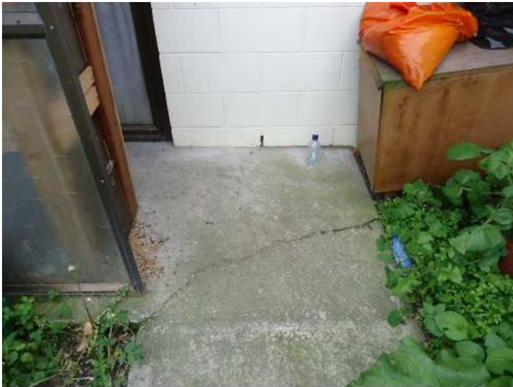
Figure 7: A 5 mm diagonal crack developed at the concrete footpath, Middle building. There are no signs of damage on the cladding.
