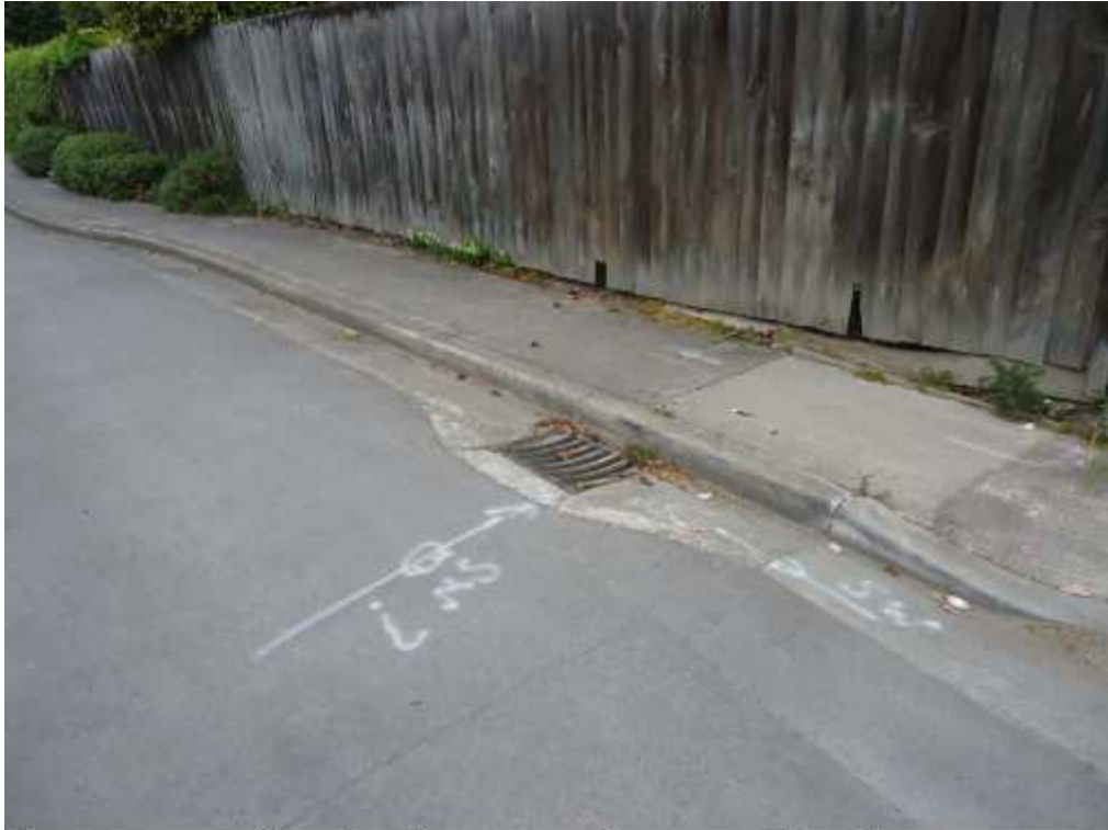
Figure 1: Up to 50 mm of heaving has occurred surrounding the storm water sewer in the entrance area.
