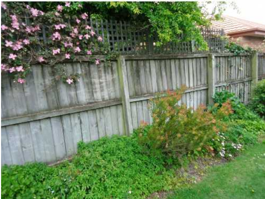
Figure 10: A wooden fence at the West side of Biddick Courts that leans outwards towards the adjacent property. The tilt is estimated as 10°.
