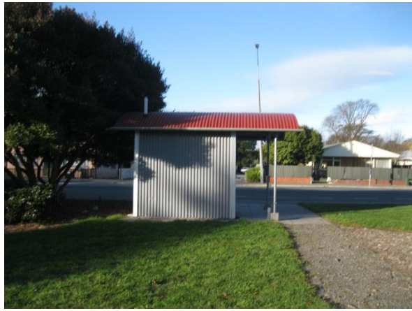
Western elevation of the Beverley Park Toilets.
