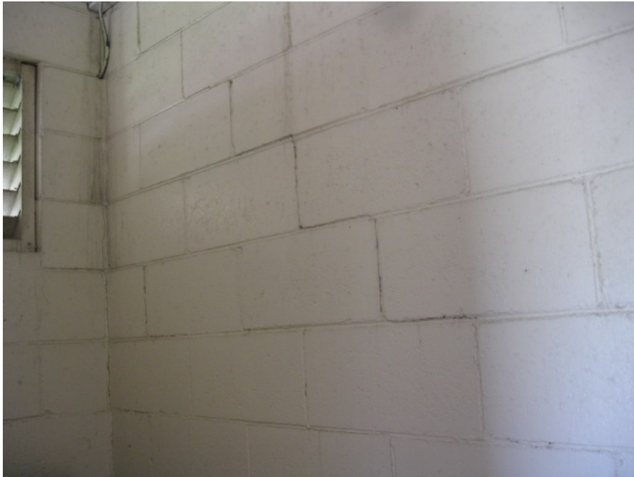
Photograph 11: Typical stepped cracking on the eastern wall
