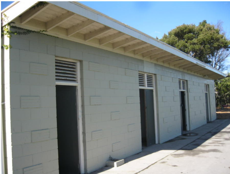
Photograph 6: Mono pitched roof and the front elevation
