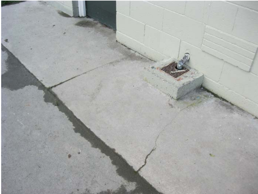
Photograph 9: Minor cracking to the exterior concrete floor slab
