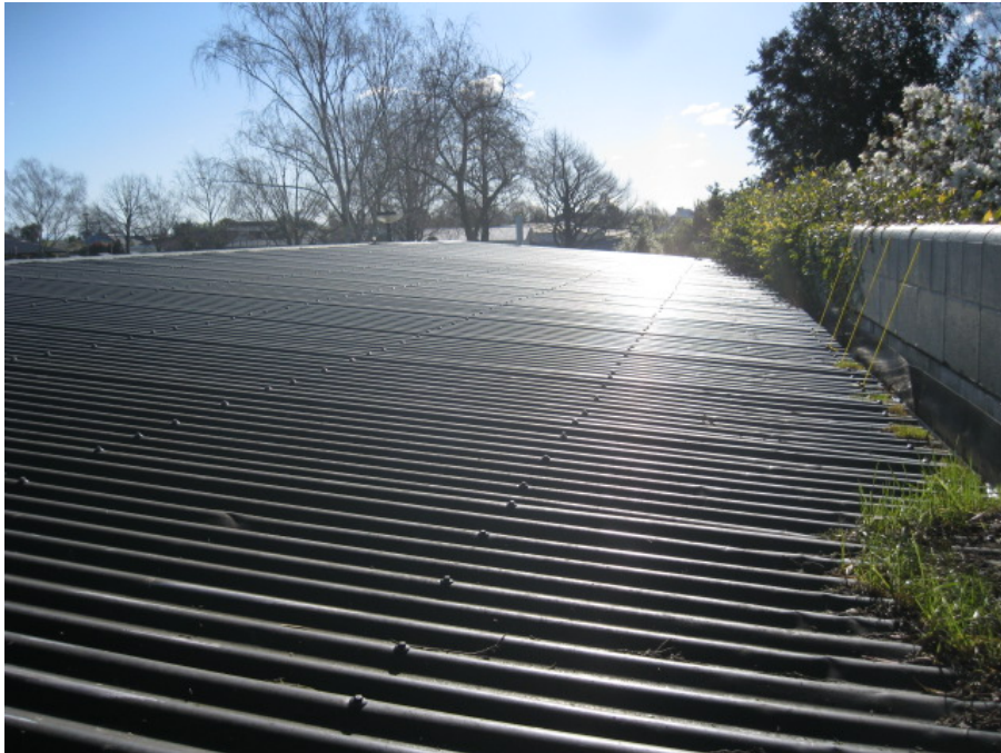
Photograph 5: Corrugated metal roofing
