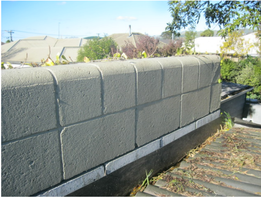
Photograph 7: Blockwork Parapet on the eastern boundary wall
