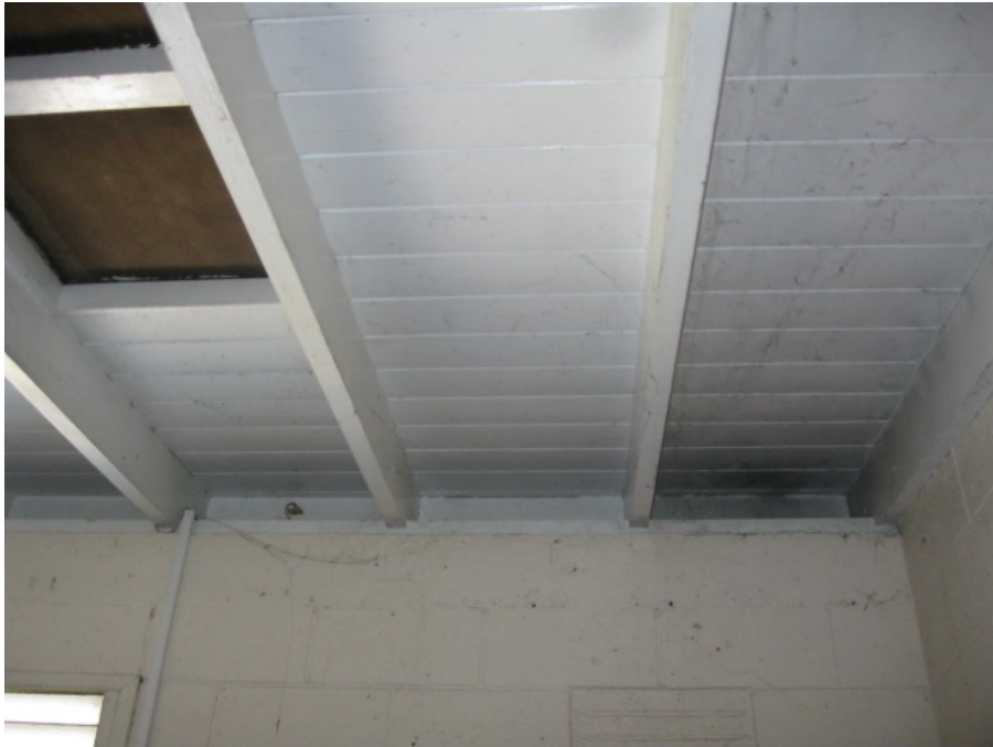
Photograph 13: Timber sarking
