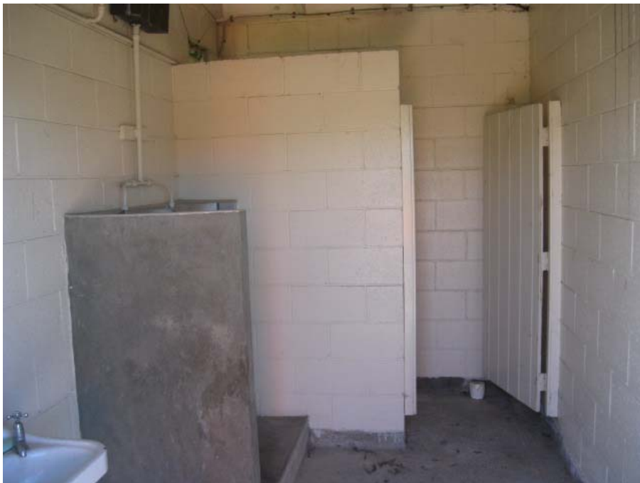
Photograph 10: Cantilever partition wall in the toilet area
