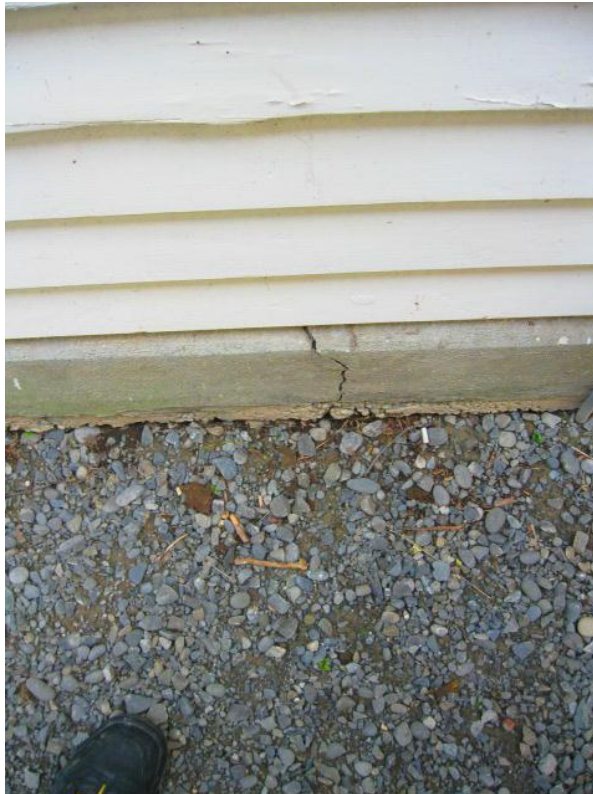
Photograph 5 Typical of cracking to the foundations
