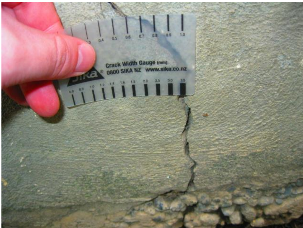
Photograph 6 Crack width is greater than 3.5 mm
