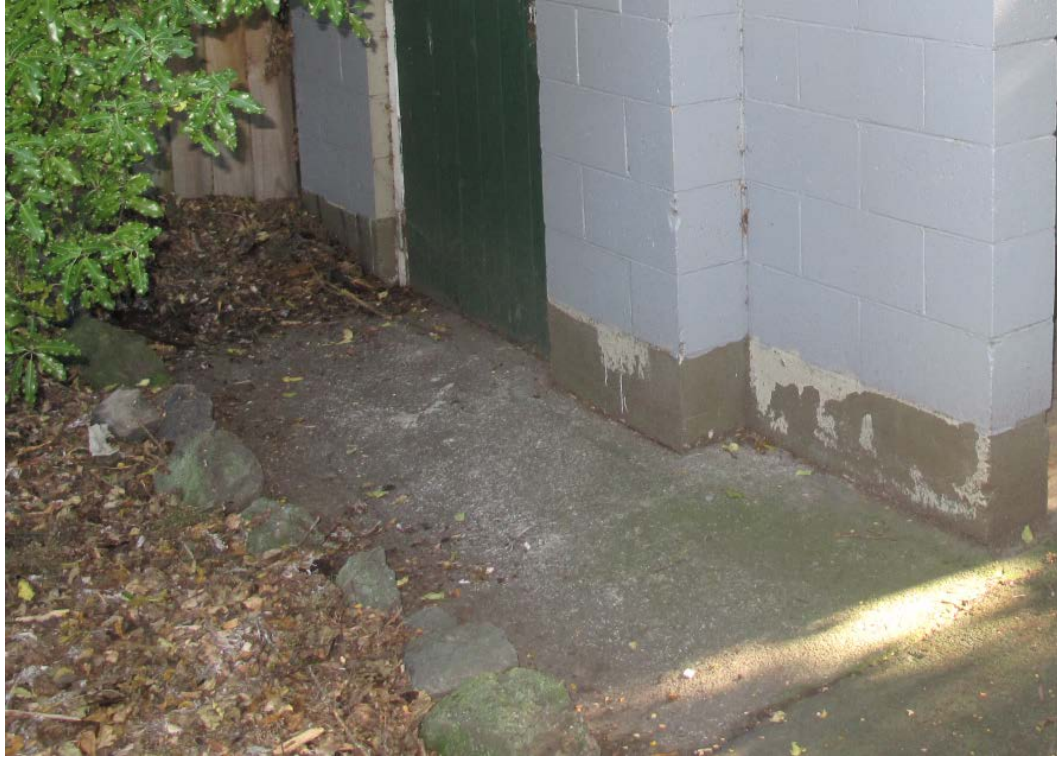
Photograph 5 Cracking in the concrete path on the south side may indicate differential movement.
