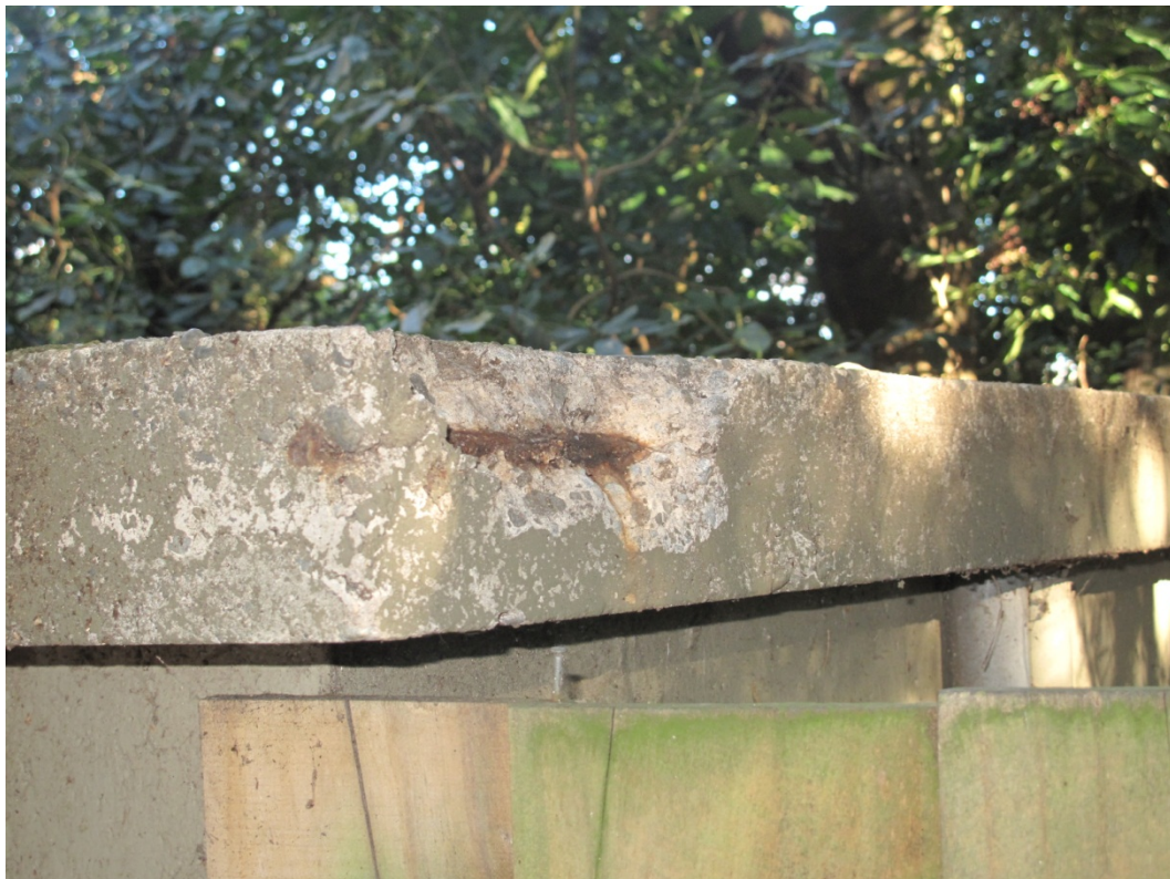
Photograph 6 Corrosion on the edge of the concrete roof slab appears to be historic.
