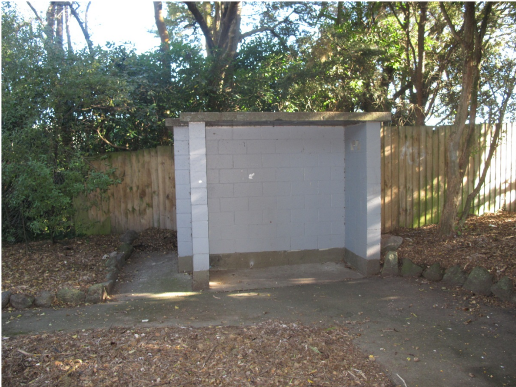
Photograph 2 View of the shelter from the east.
