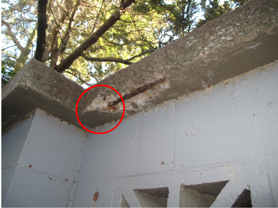
Photograph 7 The concrete exposed around the spall appears fresh.
