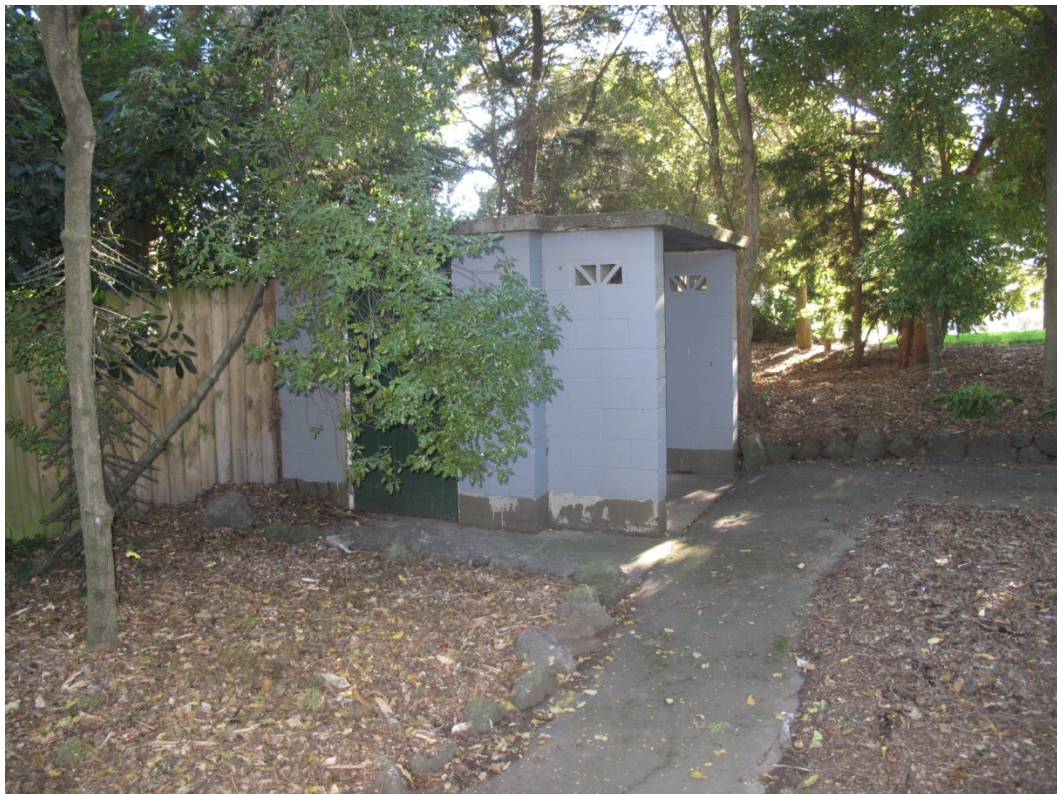
Photograph 4 The building is located near the top of the slope above the Heathcote River.
