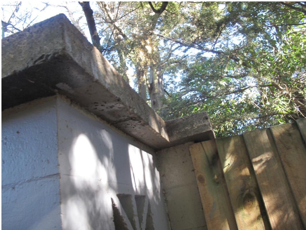
Photograph 8 The heavyweight roof increased the height of the seismic mass.
