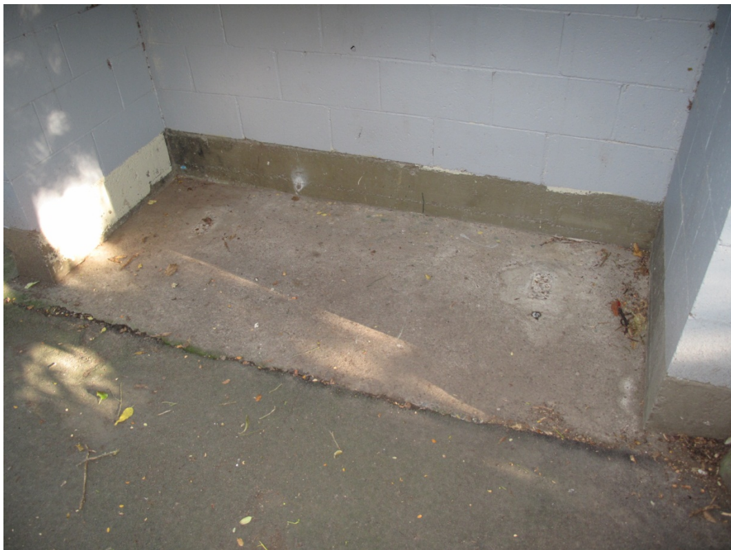
Photograph 10 No visible damage or cracking of the concrete slab on grade floor.
