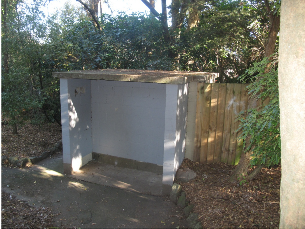
Photograph 9 The simple structure appears to be adequately braced.
