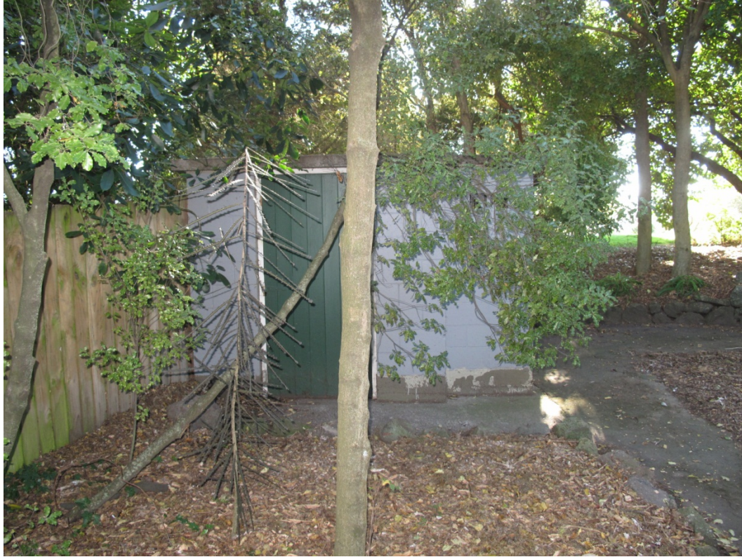
Photograph 3 View of the shelter/shed from the south.
