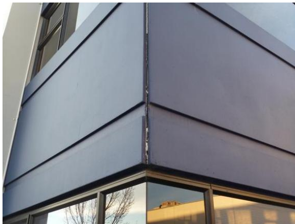
Figure 3: Corner joints, external walls
