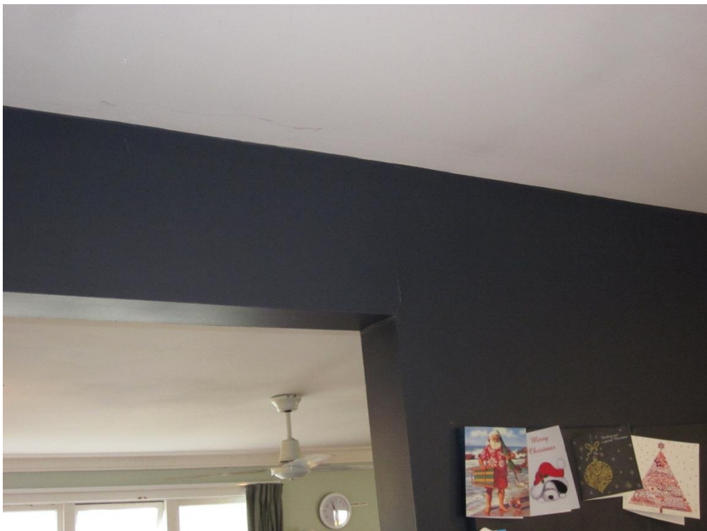
Photograph 4 Vertical cracking in plasterboard lining of timber beam where original exterior wall was removed.
