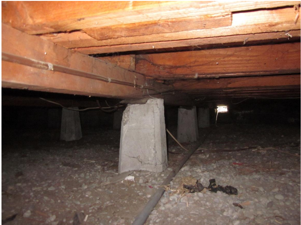
Photograph 9 Suspended timber floor support system of the original structure as seen from the access manhole.
