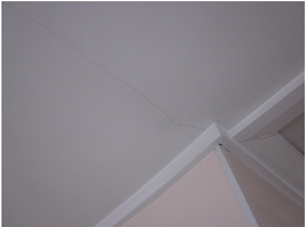
Photograph 10 Minor cracking to the ceiling plasterboard in the bathroom.
