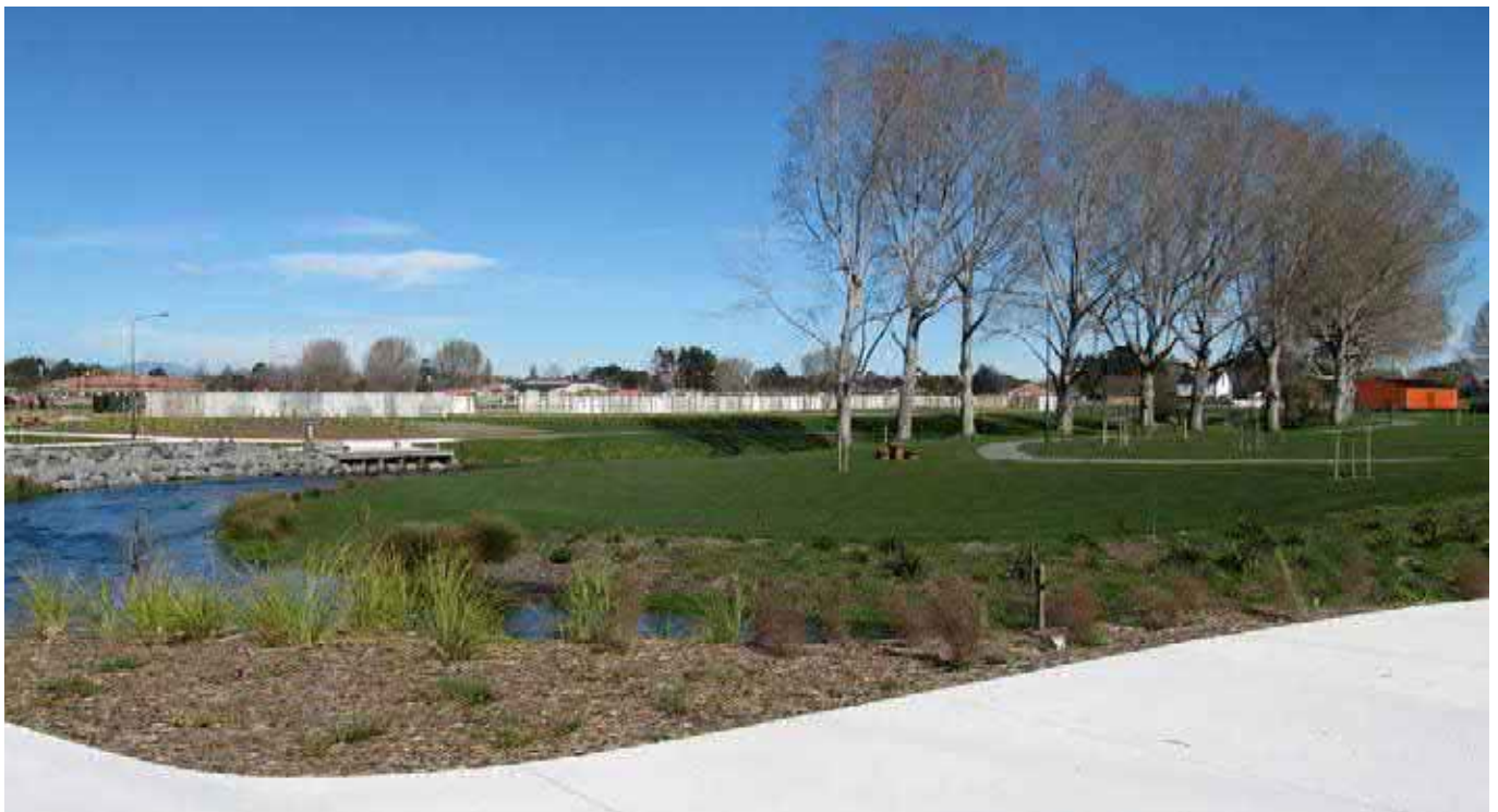
Silverstream, Kaiapoi. Stormwater facility.
