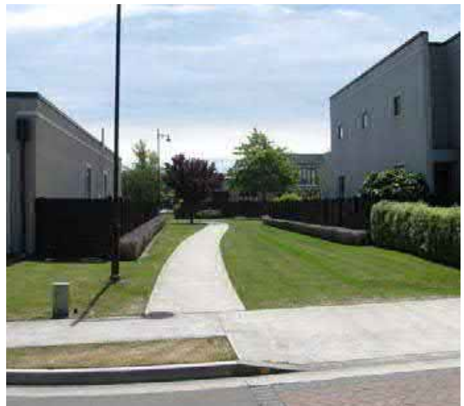
Northwood, Belfast. A walkway reserve is overlooked and has a clear view through.
