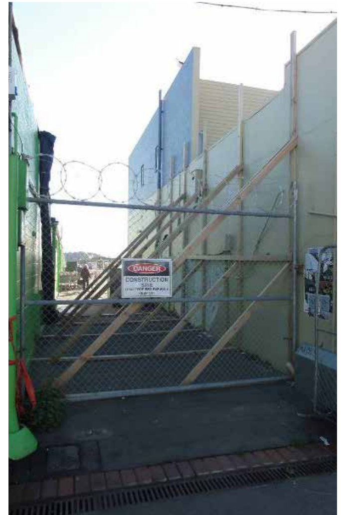
Figure 49: Earthquake damaged building, New Brighton.
