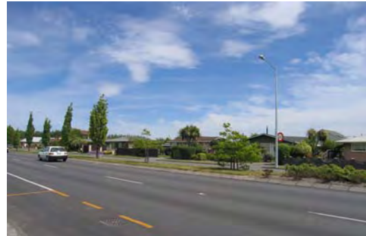
Main North Road frontage adjacent to Section 293 site
